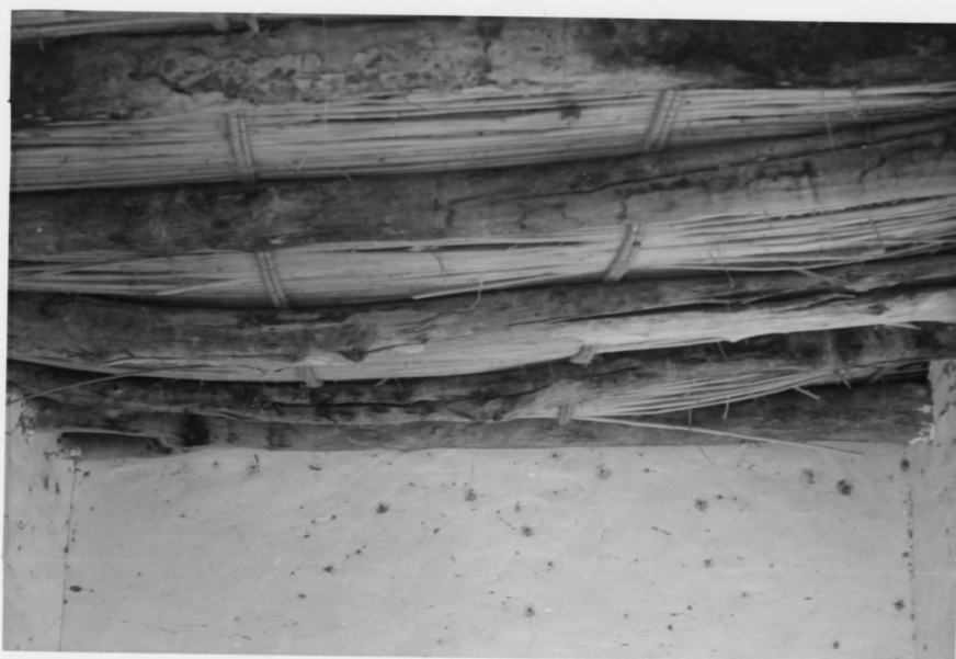
INTERIOR OF ONE-ROOM SHED, BBH-616 Note wrong placing of latia.
