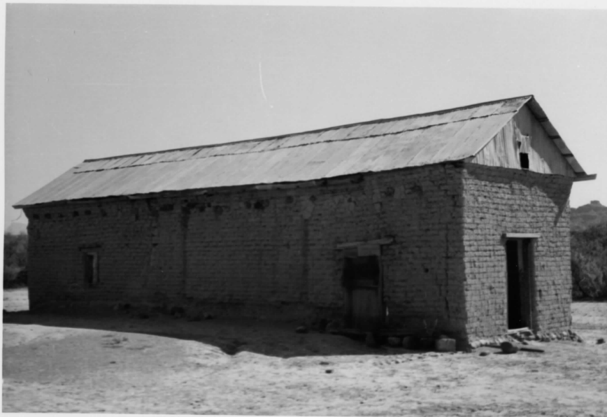
SOUTHWEST VIEW OF OLD CASTOLON STORE, BBH-618 Note erosion and failure of adobe wall.
