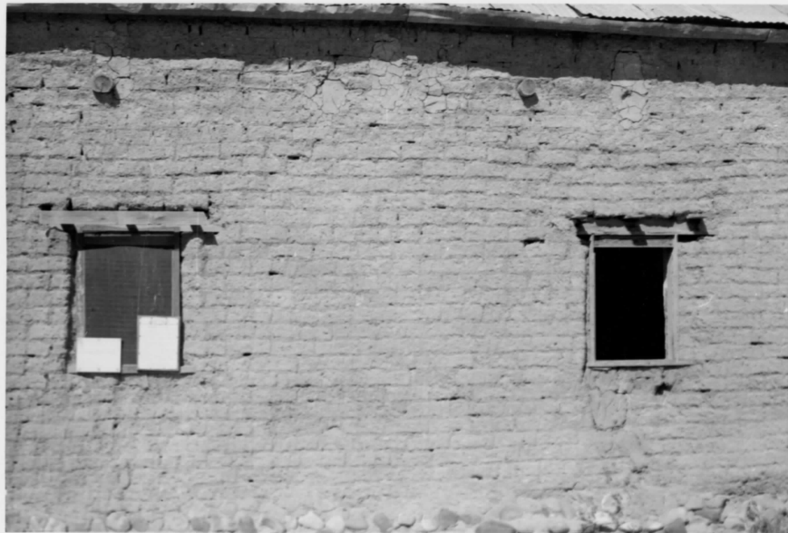
WALL DETAIL OLD STORE, BBH-618 Note remnants of window caps and condition of corrugated iron roof and gutter.
