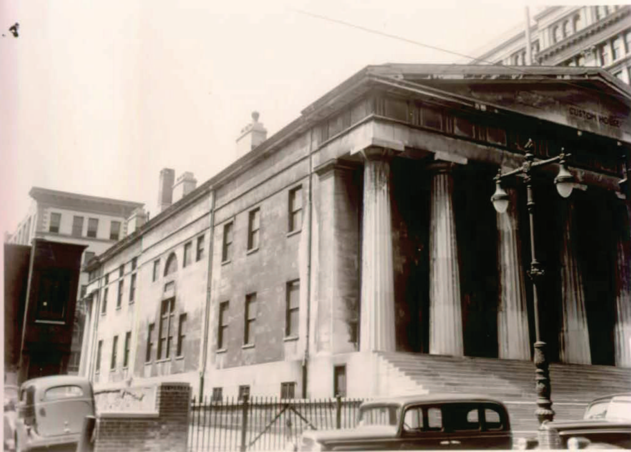
Northeast Corner - Showing good condition of Stonework Generally.
