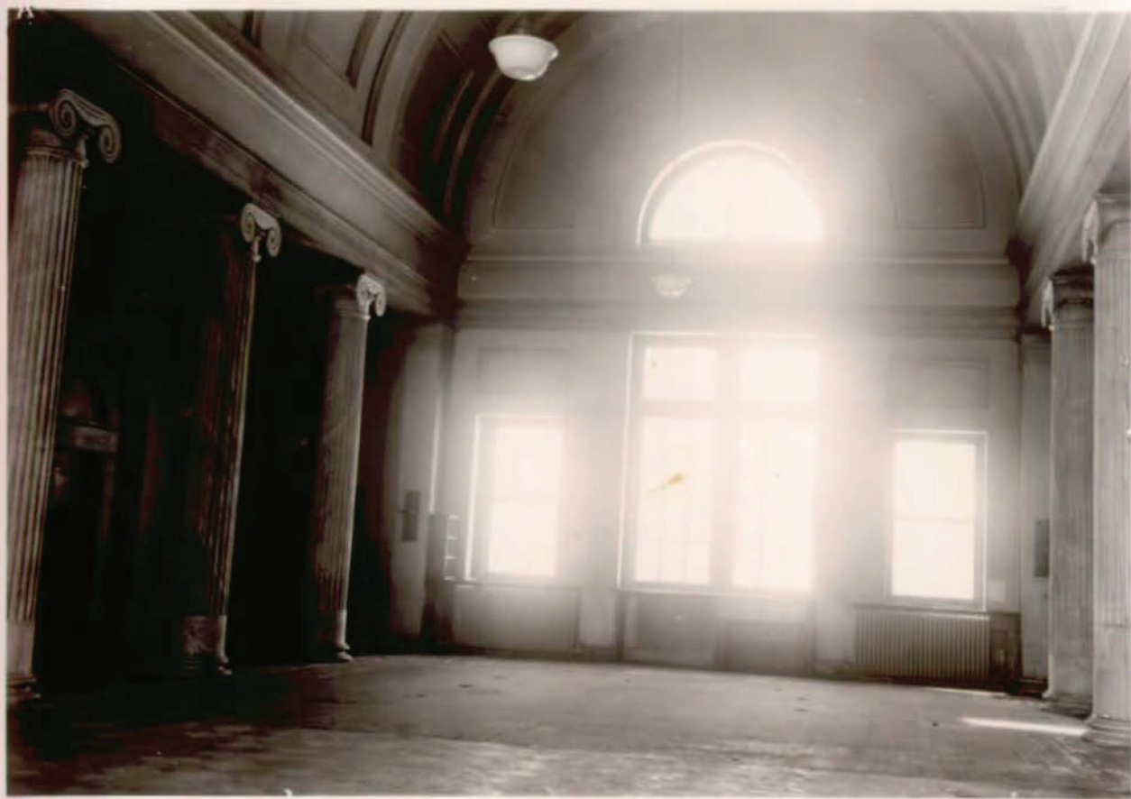
Interior of Main Banking Room. It has been agreed that this room should be restored to its original appearance.
