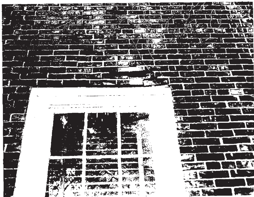
Fig. 10. North end of east wall. Note bricks above window.
