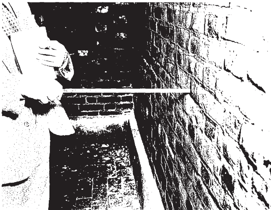
Fig. 6. West wall of south arm, showing interstice \pm 9'' deep. Behind this wall is a vault in which are kept early church records.
