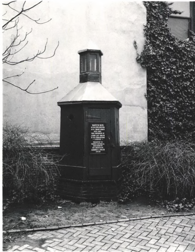
Photograph of old watchbox in yard of Friends Meeting House, Arch Street at Third. This watchbox was located at Eighth and Walnut Streets until 1850 and later removed to its present location and placed on a brick base. Note its hexagonal shape and the peep-holes which appear on four sides of the box. The lower part of the watchbox has rotted and been repaired with new work.
