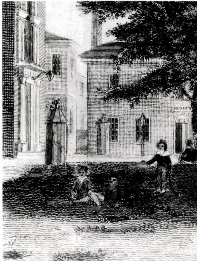
Detail of watchboxes at rear of State House. Note hexagonal shape of both boxes. Note especially what could be funnels emanating from peak of each roof. Stoves are known to have been used in watchboxes at the State House. From Birch print, 1799, in Collection, Independence National Historical Park, Plate No. 22.
