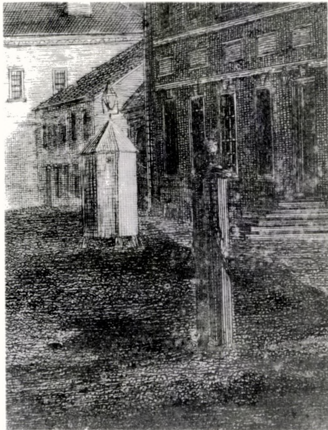
Detail of watchbox before State House. Note hexagonal shape, lamp on forked bracket atop watchbox, and splayed "feet" upon which box rests. Note also circular peep-hole on one side. From Birch print, 1798, in Collection, Independence National Historical Park, Plate No. 21.
