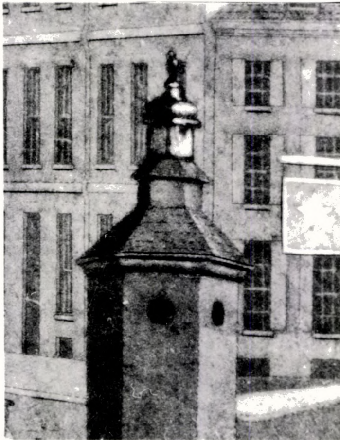
Detail from engraving of Philadelphia Exchange showing six-sided watchbox. Note peep-holes, shape of moulding at edge of roof, and texture of roof itself, possibly indicating shingling. Appearance of lighting device at top of watchbox should also be noted. Photograph in Independence National Historical Park files, negative No. 1692.
