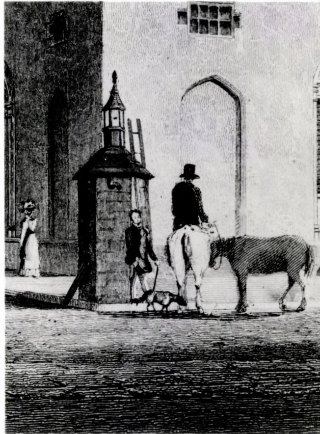
Detail of hexagonal watchbox near Academy of Natural Science. Note appearance of roofing and of siding on box itself. Notice especially the suggestion of a peep-hole near roof line. Curved pipe protruding from hole was probably connected to stove inside. From engraving by C. Burton, 1831, in Collection, Independence National Historical Park.
