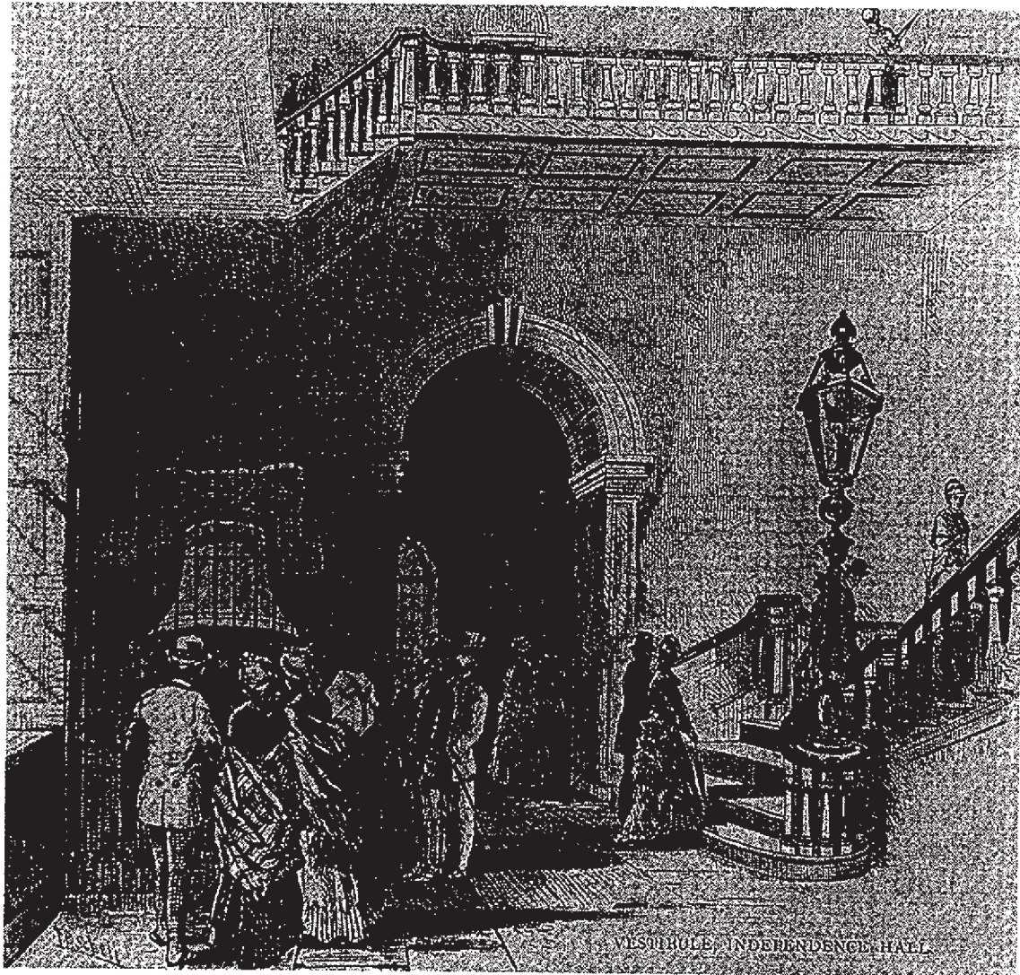
Figure 4. F.B. Schell's "Vestibule, Independence Hall" in 1875 illustrates the presence of stone paving in the Tower Stairhall and the location of the Liberty Bell in the northwest corner (Temple University Urban Archives print reproduced in Stevick 1996:51).
