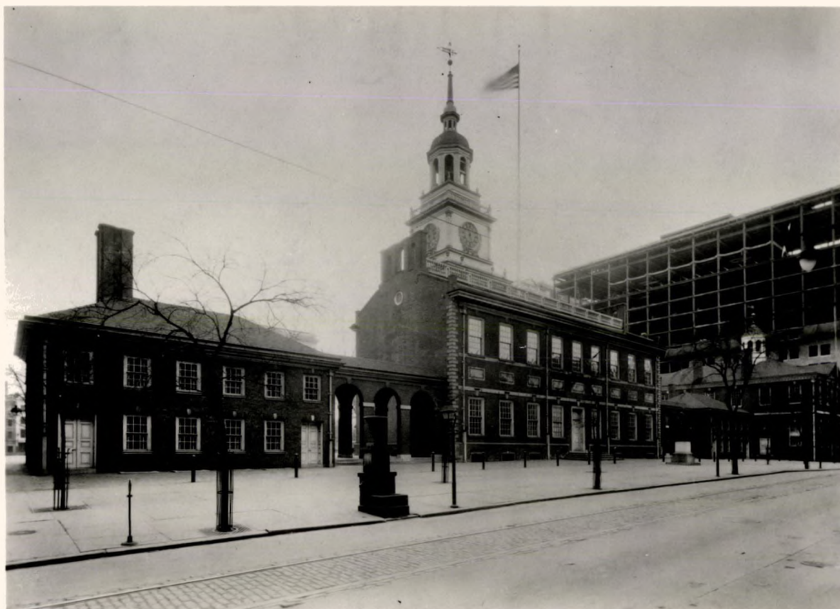
Independence Hall, 1925. The rectangular copper downspouts as they appear today. Courtesy of City of Philadelphia.
