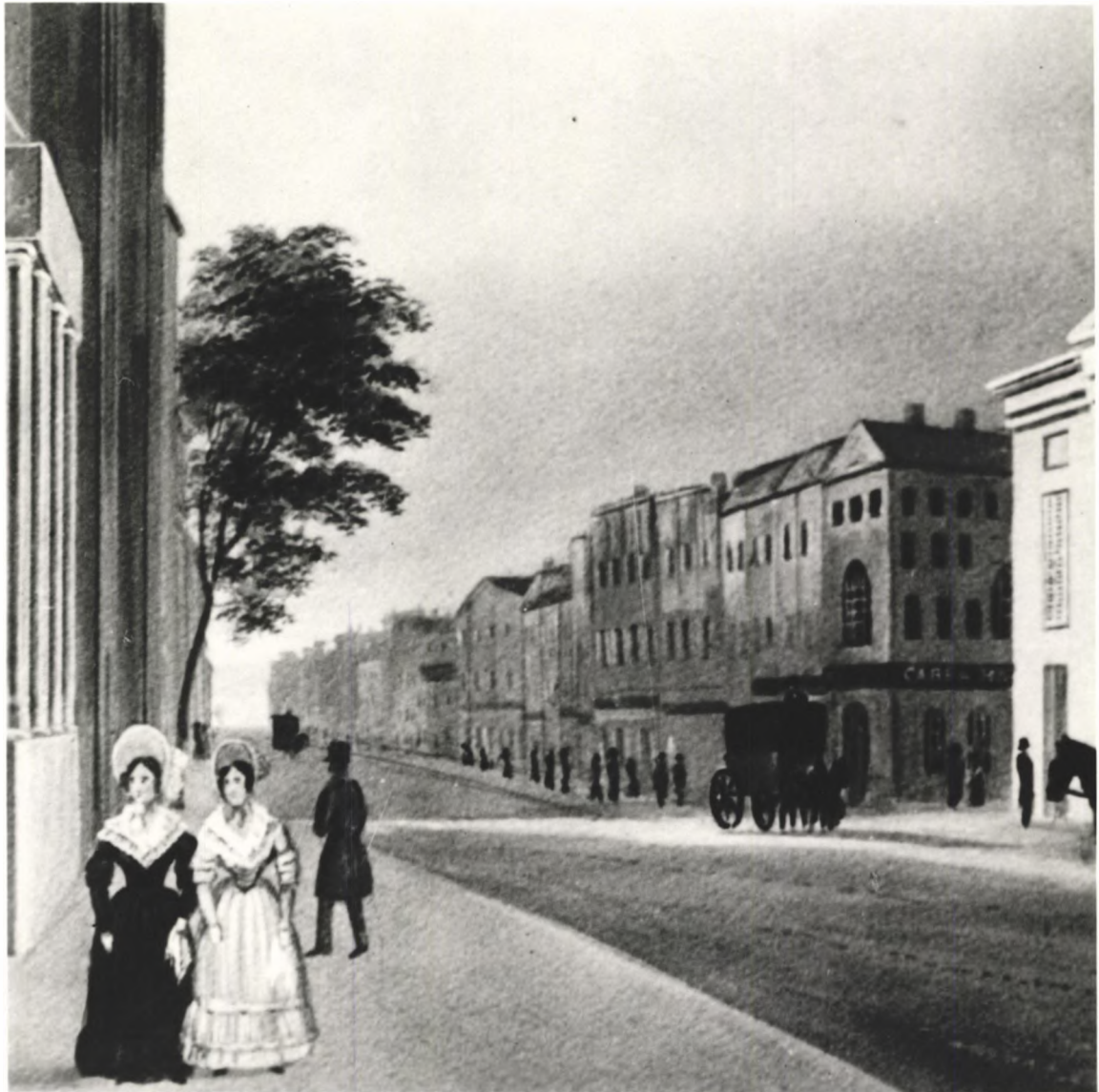
Joseph Pemberton House at midterm. William Strickland post-1836 watercolor shows in background not-yet-altered house on other side of four-story structures at 118 and 120 Chestnut Street. Note particularly forward slope of roof. Photograph in Independence National Historical Park files.
