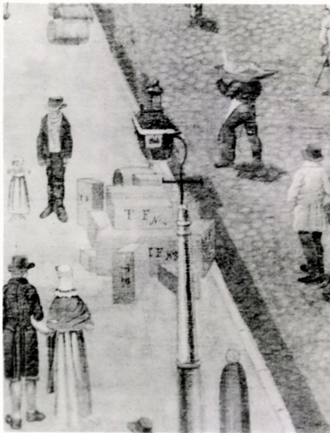
Detail of lamp on corner of Market Street at Second. Note the appearance of the funnel and the crook-shaped bracket with cross-piece. Photograph in Independence National Historical Park files, negative No. CN 13112.
