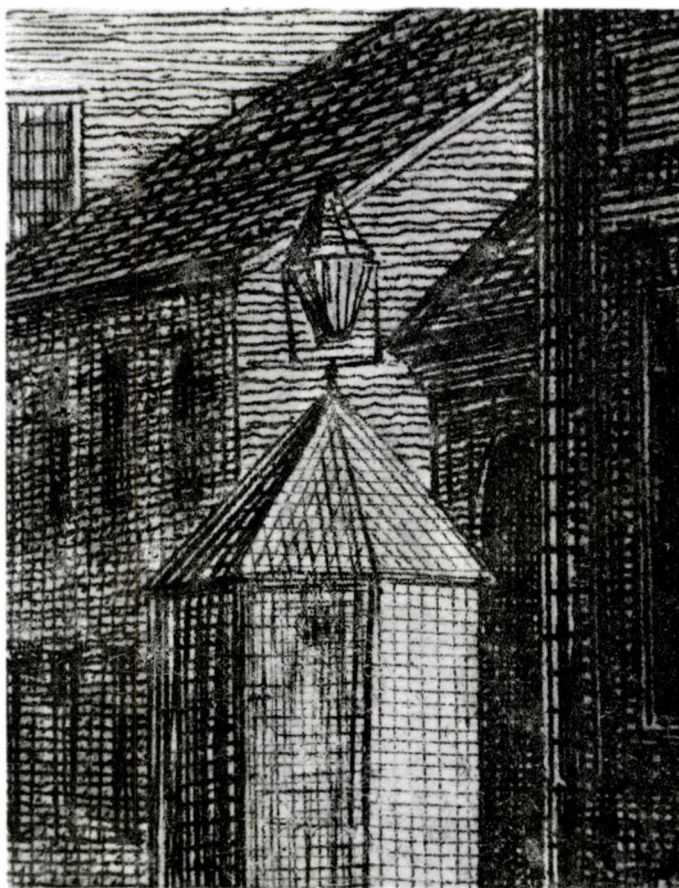
Detail of watchbox Lamp before State House. Note forked bracket and hexagonal shape of head, from Birch print 1798, in Collection, Independence National Historical Park, Plate No. 21.
