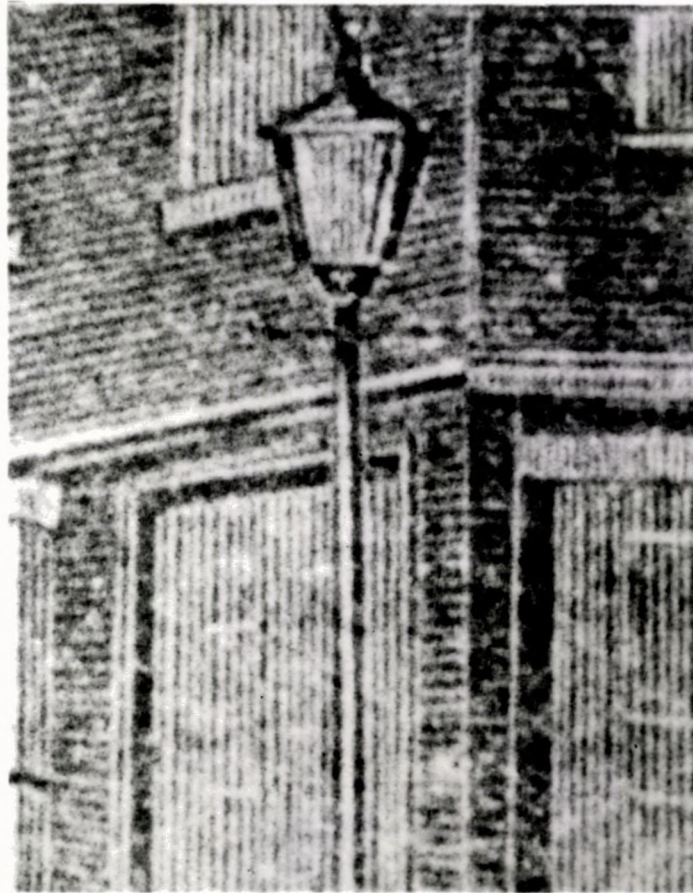
Detail of lamp located at edge of footway on the corner. Note attachment between post and head of lamp, position of cross-piece, and funnel atop lamp. (See E. P. Oberholtzer, Philadelphia: A History of the City and its People , II, 298.)
