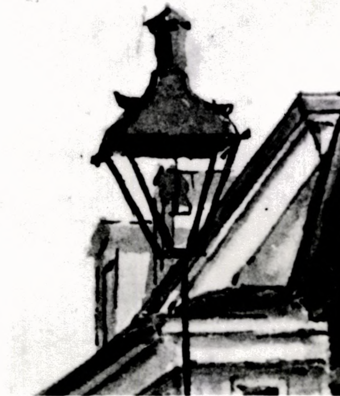
Detail of lamp located near Drawbridge Wharf. Note curvature of vented hood and the funnel with cap. Note appearance of bracket joining lamp to post, and point of attachment between lamp and bracket. Photograph in Independence National Historical Park files, negative No. A-2204.
