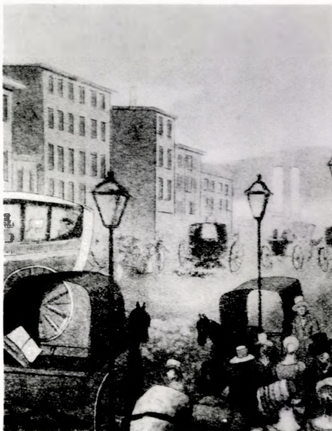
Detail of lamps along Chestnut Street in vicinity of Sanderson's Franklin House. Note that hoods of all lamps appear to be of glass, and that heads rest directly upon standards. Note also the uniform placement of public lamps along Chestnut Street. Photograph from Independence National Historical Park files, negative No. 213.
