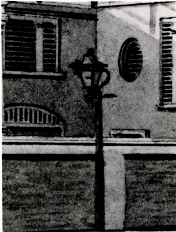
Detail of lamp in vicinity of President's House. Note contour of lamp's hood, curvature of bracket, position of cross-piece, and plain post. From engraving by William Strickland, c. 1830. Photograph in Independence Historical Park files, negative No. 301.
