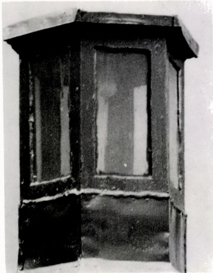
Detail from photograph showing lighting device atop old watchbox. Note hexagonal shape and rectangular glass panes. Photograph from Independence National Historical Park files, negative No. 1405.
