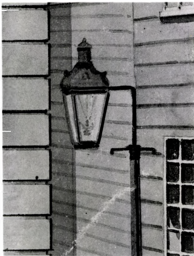
Detail of lamp next to Lafayette Arch showing right angle bracket, cross-piece and wires and cup in lamp. From S. H. Kneass watercolor sketch in Collection, Independence National Historical Park, Museum SN 14.001.
