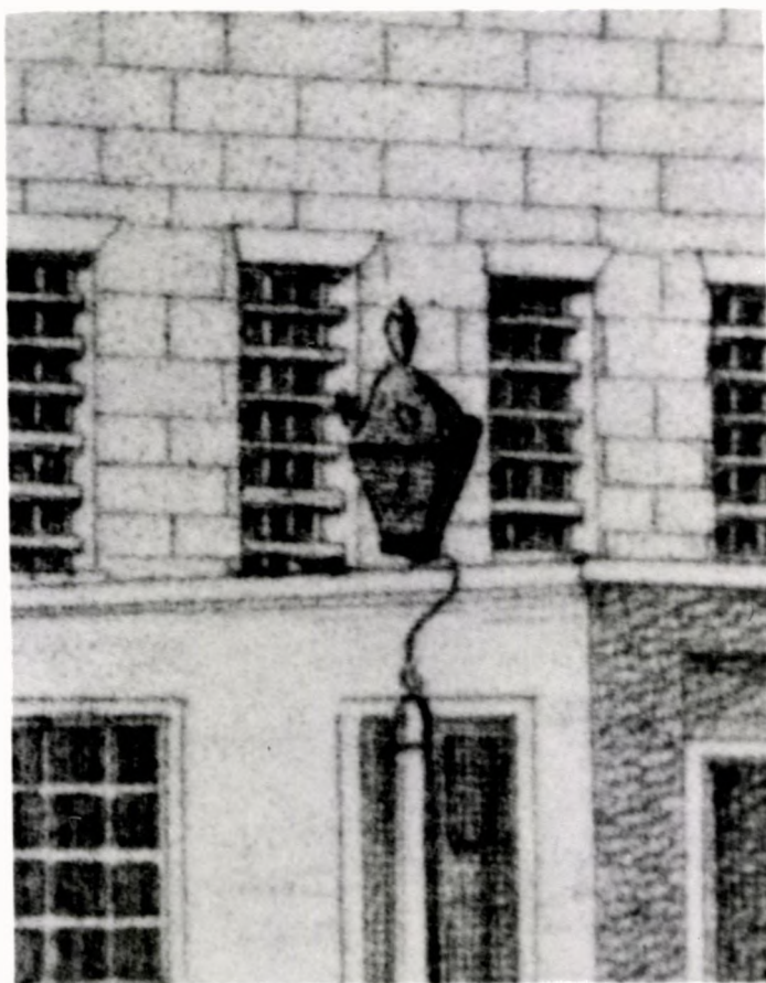
Detail of lamp in front of Walnut Street Jail. Note configuration of bracket and point of attachment. Also shape of funnel and suggestion of finial atop it. Hood is "s"-shaped with vents. Plain wooden post has cap, perhaps to prevent splitting. From Birch print; photograph in Independence National Historical Park files, negative No. 422.
