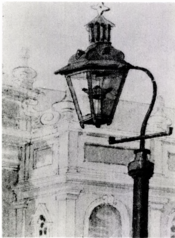
Detail of lamp in Svin'in watercolor is definite as to several of installation's features. Note especially double-branch fixture in lamp, shape of lamp head including vented "s"-shaped hood, vents in funnel, shape of cap and its finial. Note also bracket and location and design of cross-piece. Post has cap with moldings, but is in other respects typical. Photograph from reproduction in Pennsylvania Magazine of History and Biography , LXXV, following p. 24.
