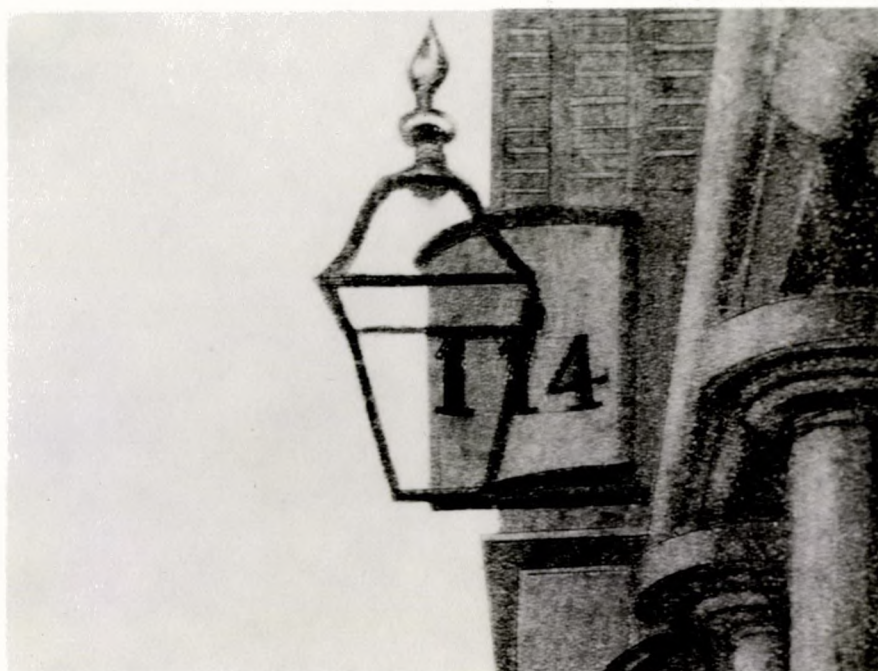
Detail of lamp attached to building across the street from Sanderson's Franklin House. Note manner in which lamp is bracketed to building. Note curvature of glass paned hood, and the funnel surmounted by cap with finial. Photograph from Independence National Historical Park files, negative No. 213.
