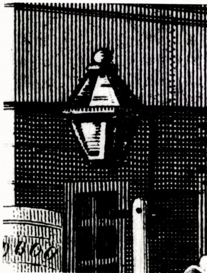
Detail of lamp on Chestnut Street. Note design of bracket and post with bolt to hold cross-piece. From Thomas Birch print; photograph in Independence National Historical Park files, negative No. 1724.
