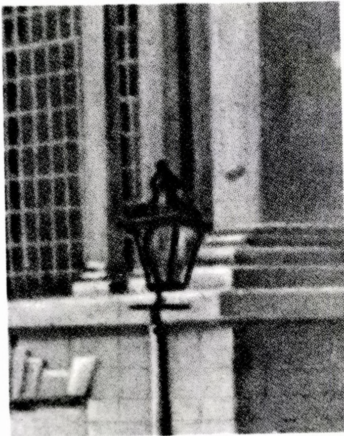
Detail of lamp on Second Street, in front of Christ Church, showing "s"-shaped hood, crook-shaped bracket, cross-piece above post, and high-crowned funnel cap, from 1811 painting by William Strickland, in Collection, Independence National Historical Park, Museum No. 1126.
