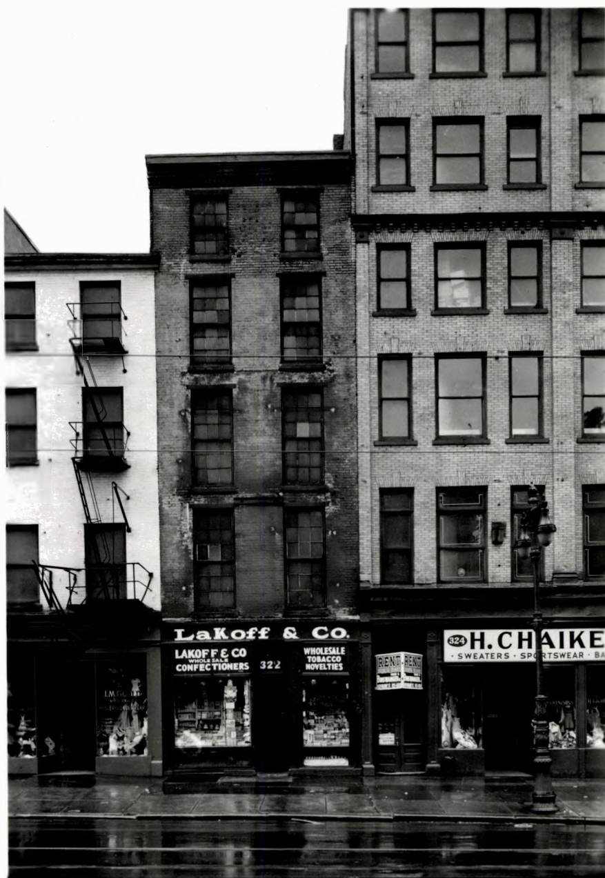
322 Market Street, looking south, 1951. Note jointure of roof to adjoining building. National Park Service photo.
