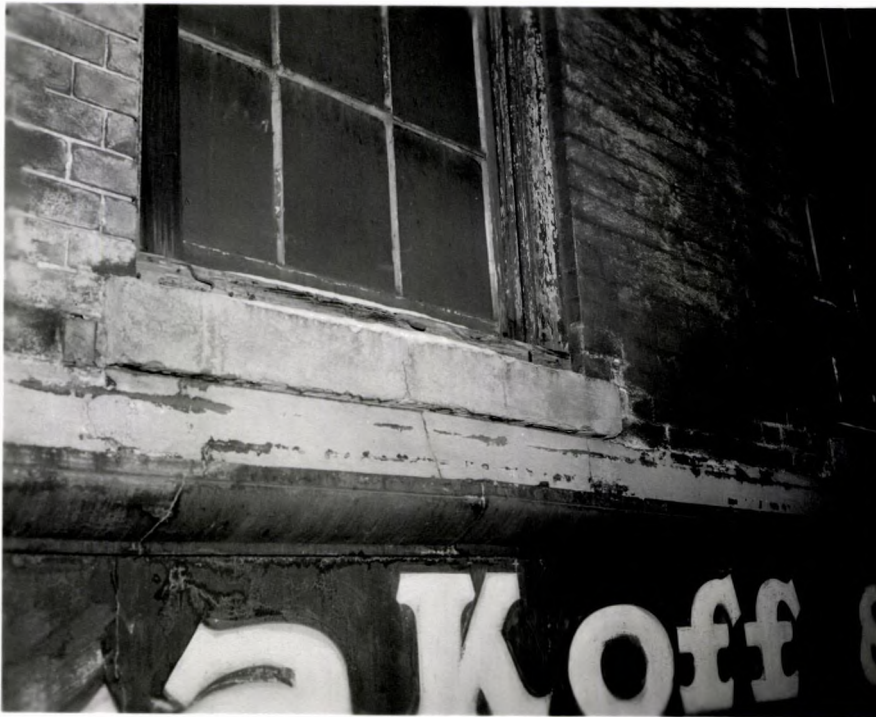
Stone band course of building at 322 Market Street can be seen between sign and window sill in this 1961 photograph. Note also Flemish bond of brickwork. National Park Service Photo.
