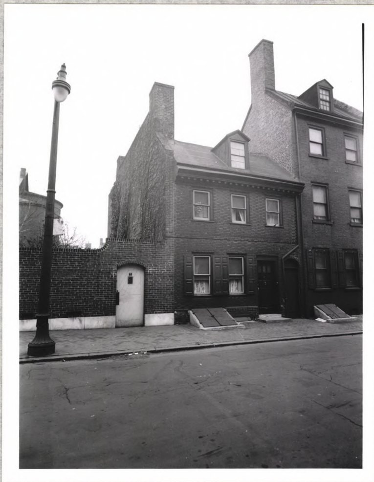
408 Locust Street. National Park Service Photo.
