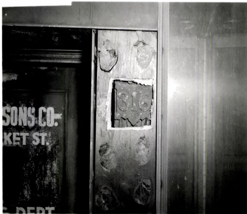
Street number found on cast-iron column beneath mirror glass of modern store front. This number is part of the casting and thus dates the remodelling as after 1854.
