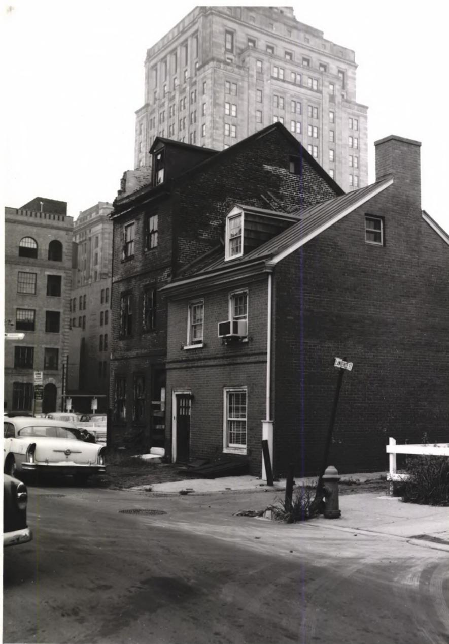
Recent view of structure at 421 Locust (423 Locust has since been restored) shows repaired building. Note the removal of the 19th century cornice.
