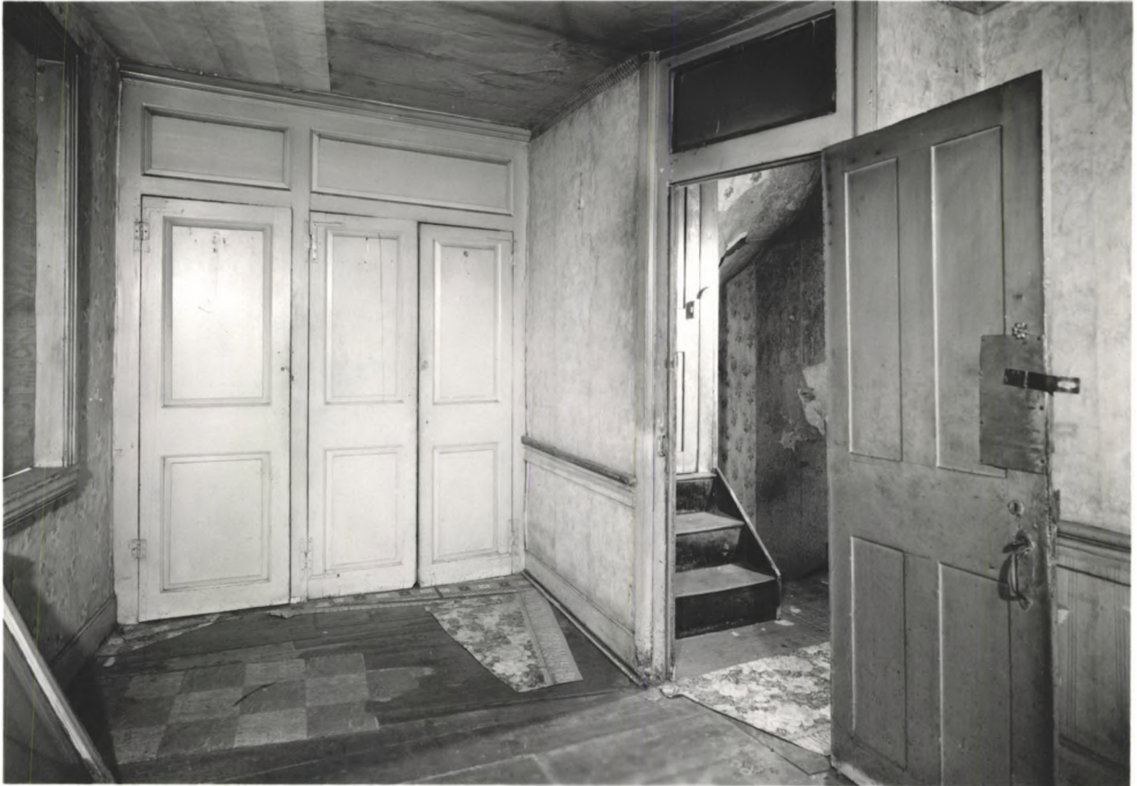
Second floor, front room of No. 20 Christian Street, looking east, 1963. Original architectural features include "HL" hinges, beaded base board, deeply-recessed panelling, chair rail, flooring, door, and casing. In hallway can be seen board newell staircase, in place since 1762-1763. National Park Service photo.
