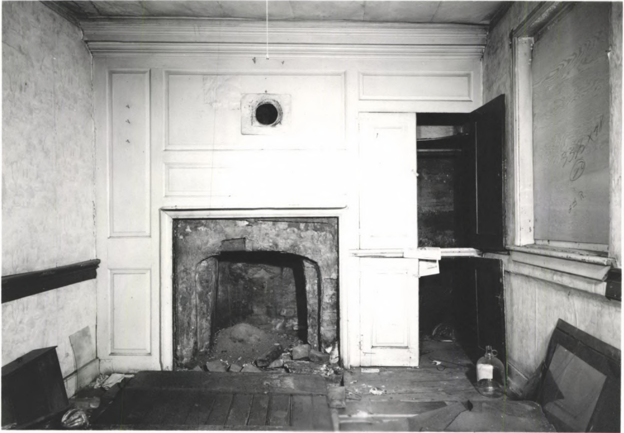
A beautiful small room: second floor, back room, No. 20 Christian Street, looking east, 1963. Panelled wall is intact survival from 1762-1763. Double architrave of cornice and shaped shelf of double-doored closet mark this as room of importance to house. Note also "HL" hinges, details of fireplace, and chair rail at left. National Park Service photo.
