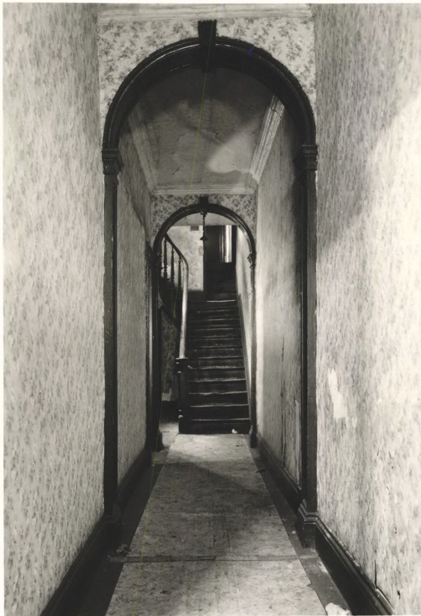
First floor hallway of No. 22 Christian Street looking south, 1963. National Park Service photo.
