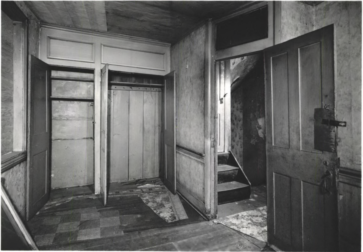
Second floor, front room of No. 20 Christian Street, looking east, 1963, closet doors open. Board for cloak pegs can be seen in closet at right, shelf profiles in closet at left. National Park Service photo.
