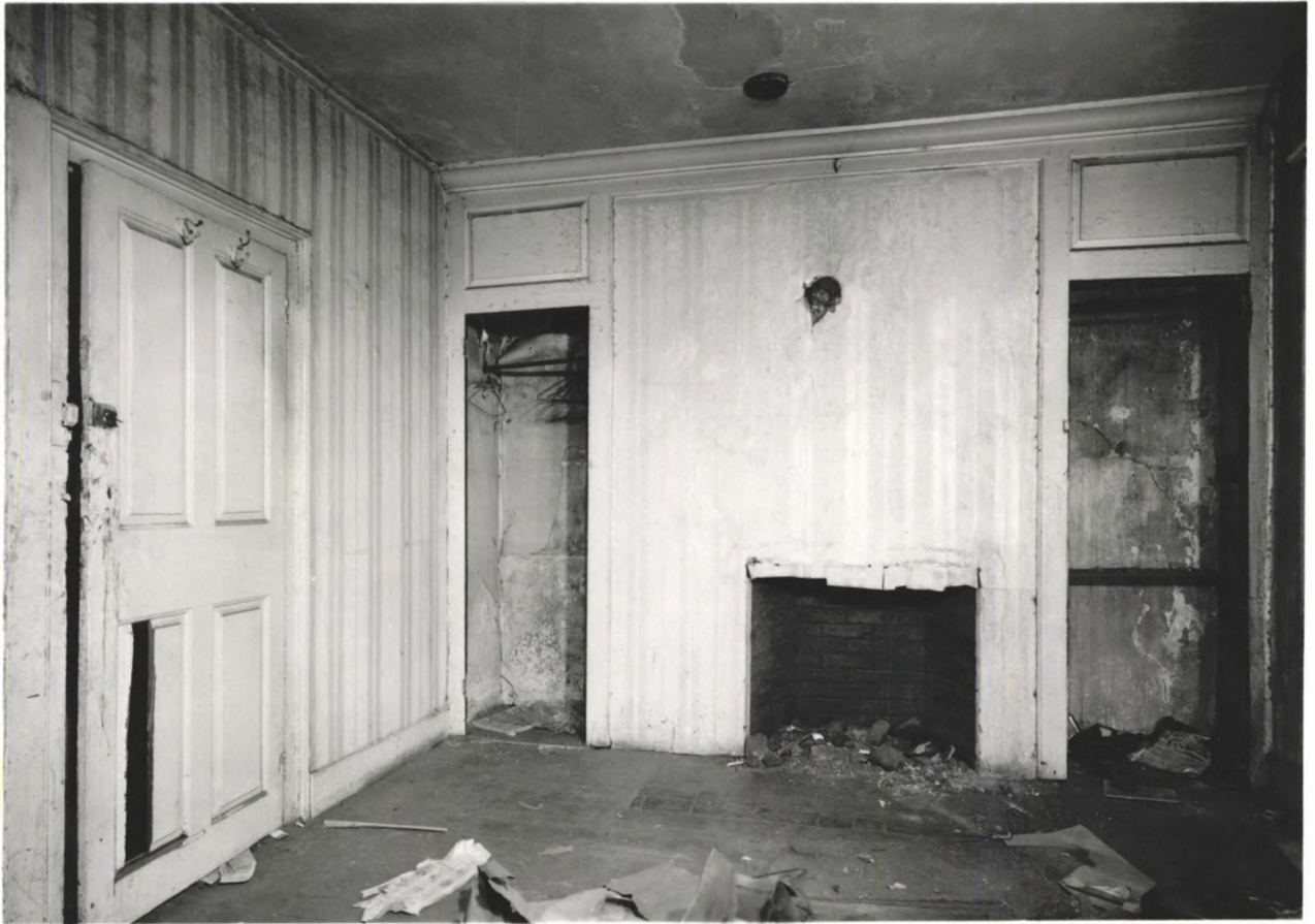
Second floor front room of No. 14 Christian Street, 1963. Deeply recessed panels over closet, pegged joinery and fireplace wall, cornice and door at left are survivals from house of 1760's. Fireplace, brick hearth, and flooring also date from this period. National Park Service photo.
