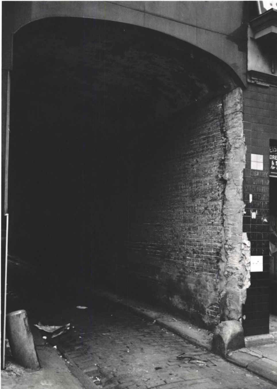
The section of passageway at the Market Street entrance to Franklin Court, 1951. Wall is of first story to 318 Market Street. Vaulted ceiling of arched passageway dates to Franklin. National Park Service photo.
