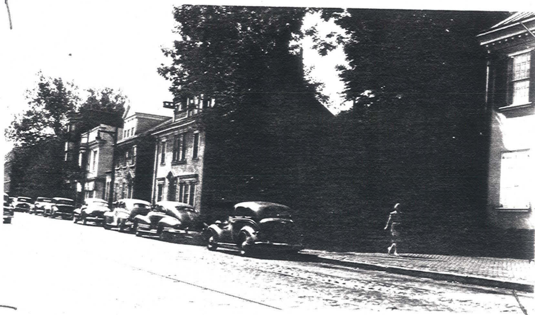
No. 7 View looking South along West side of Germantown Ave. Corner of Morris House shows at extreme right. Wood fence enclose grounds of Morris House.
