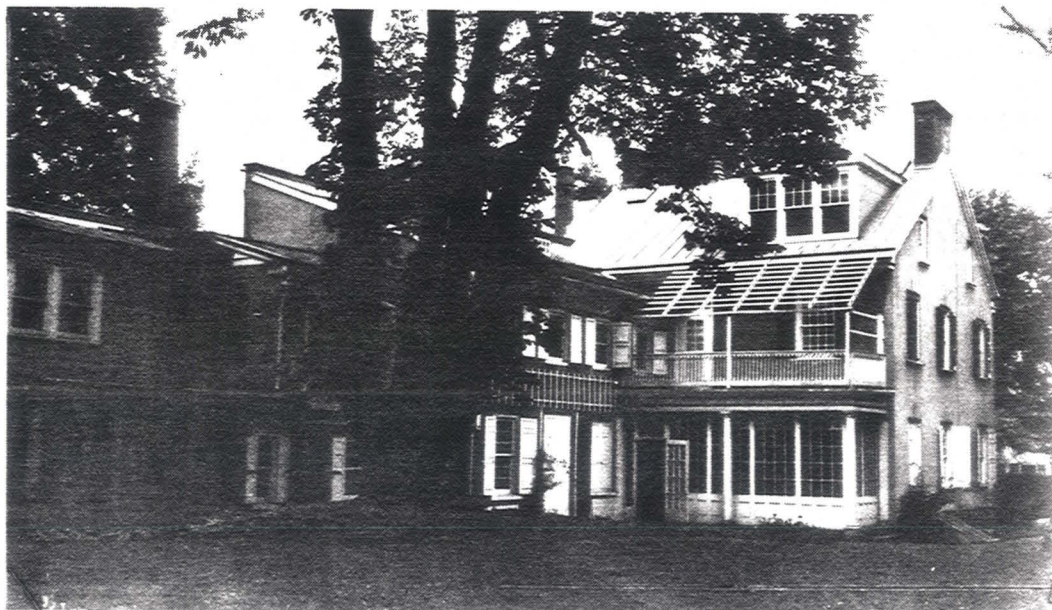
No. 9. View looking east from grounds to rear wing additions to Morris House. The enclosed porch, or conservatory, and the second story portico attached to original Beshler House shown at right. Note cellar door on right to front part of cellar under original house.
