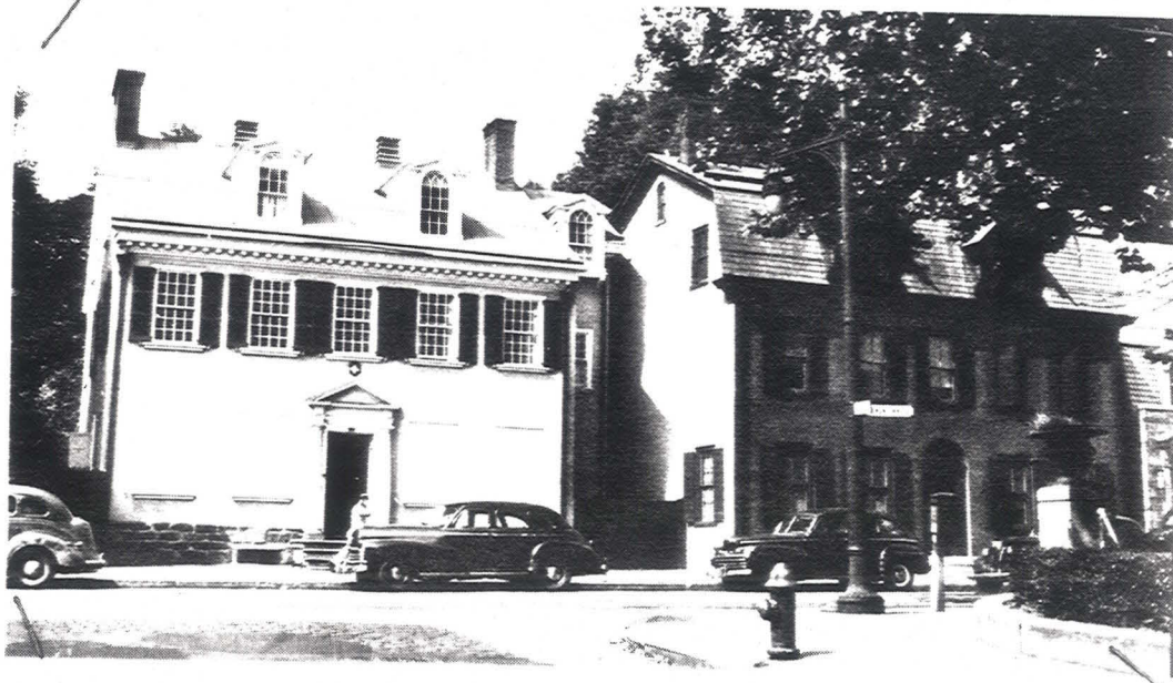
No. 5. View looking west to Morris House from Church Lane. The house to the right (north) of the Morris House dates from about 1796, excepting the Mansard roof which is a change from the original. This house is scheduled to be torn down in the near future.
