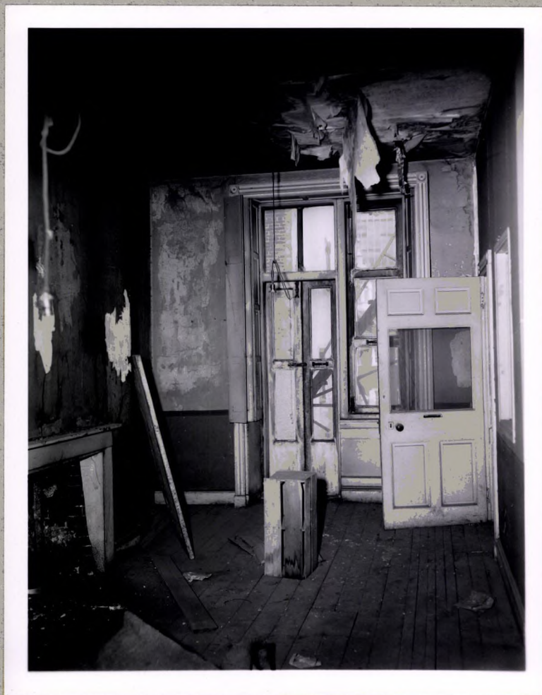
Third floor, north room, looking north.
