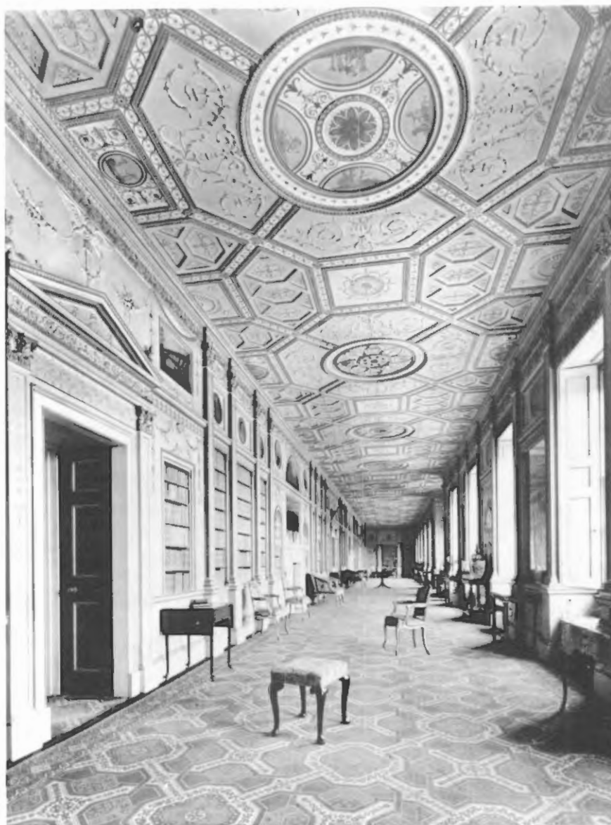
Illustration #3. Long Gallery Syon House, Middlesex, England. Architect, Robert Adam, c.1762. This Long Gallery post-dates the one in the Pennsylvania State House by thirty years, but provides us with a supreme example of the idea of the English Country house and public building area for promenades, balls, entertainments and banquets. From: English Country Houses, Mid Georgian, 1760-1800 , by Christopher Hussey. Page 93.
