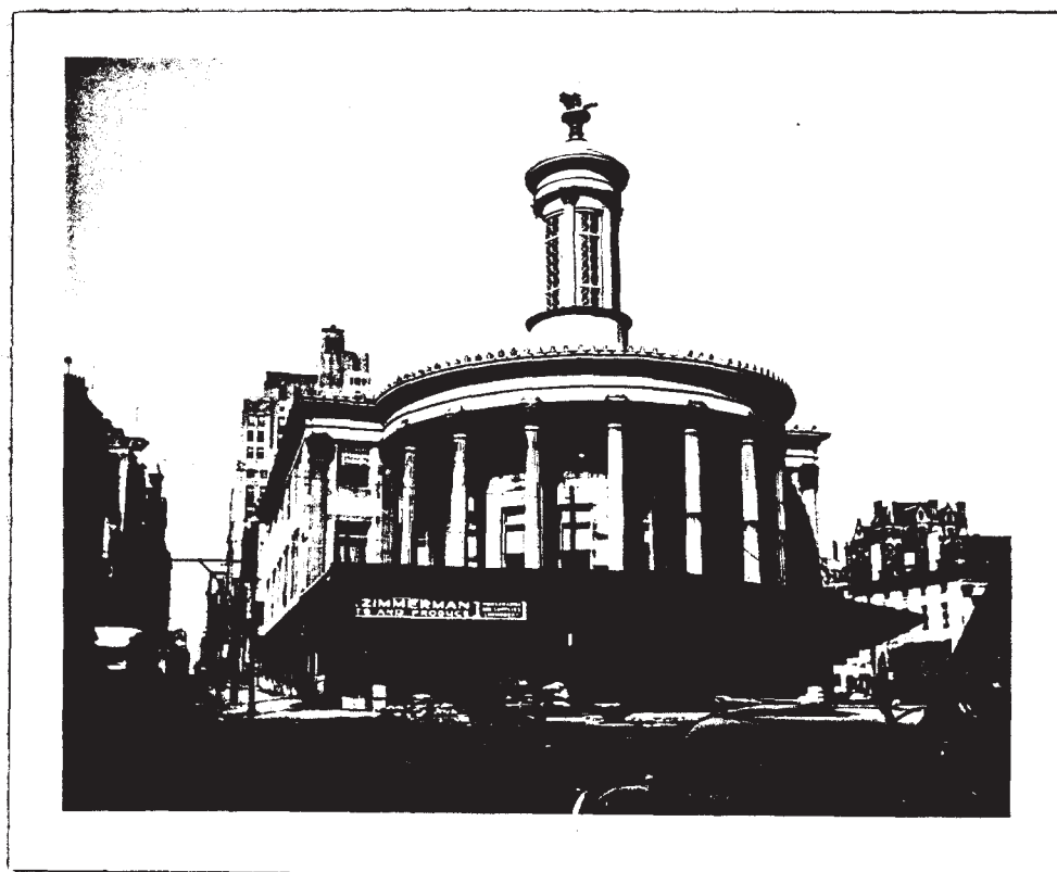
View from the southeast showing the produce sheds constructed in 1922.
