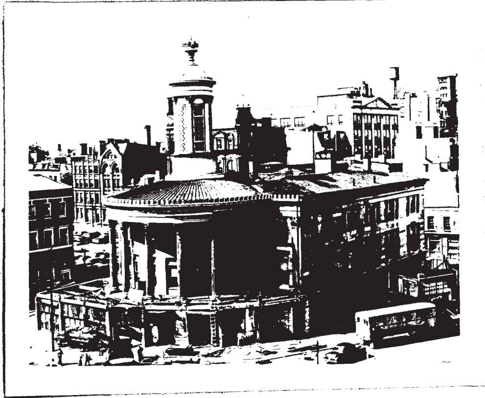
Philadelphia Exchange during demoliton of market stalls, September, 1953. National Park Service Photo.
