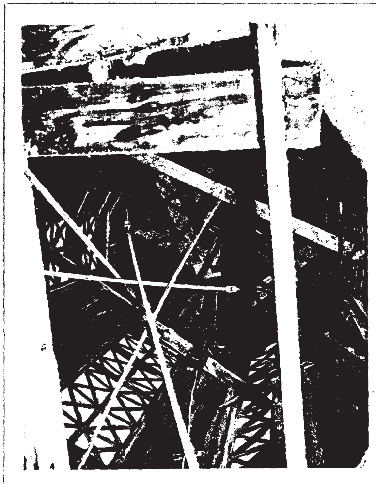
Interior view of the existing Hickman tower looking up to the roof showing methods of framing and bracing.
