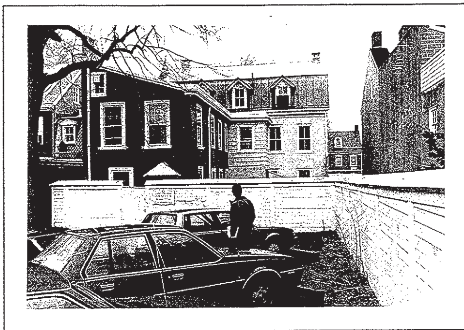
Plate 12. View of the Bringhurst House from the west. Most of the rear yard has been paved for parking.
