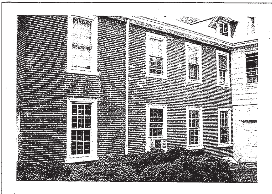
Plate 10. View of the rear extension showing Section 4 at the left of the downspout, Section 3 is to the right. Note the difference in the brick bonding patterns.
