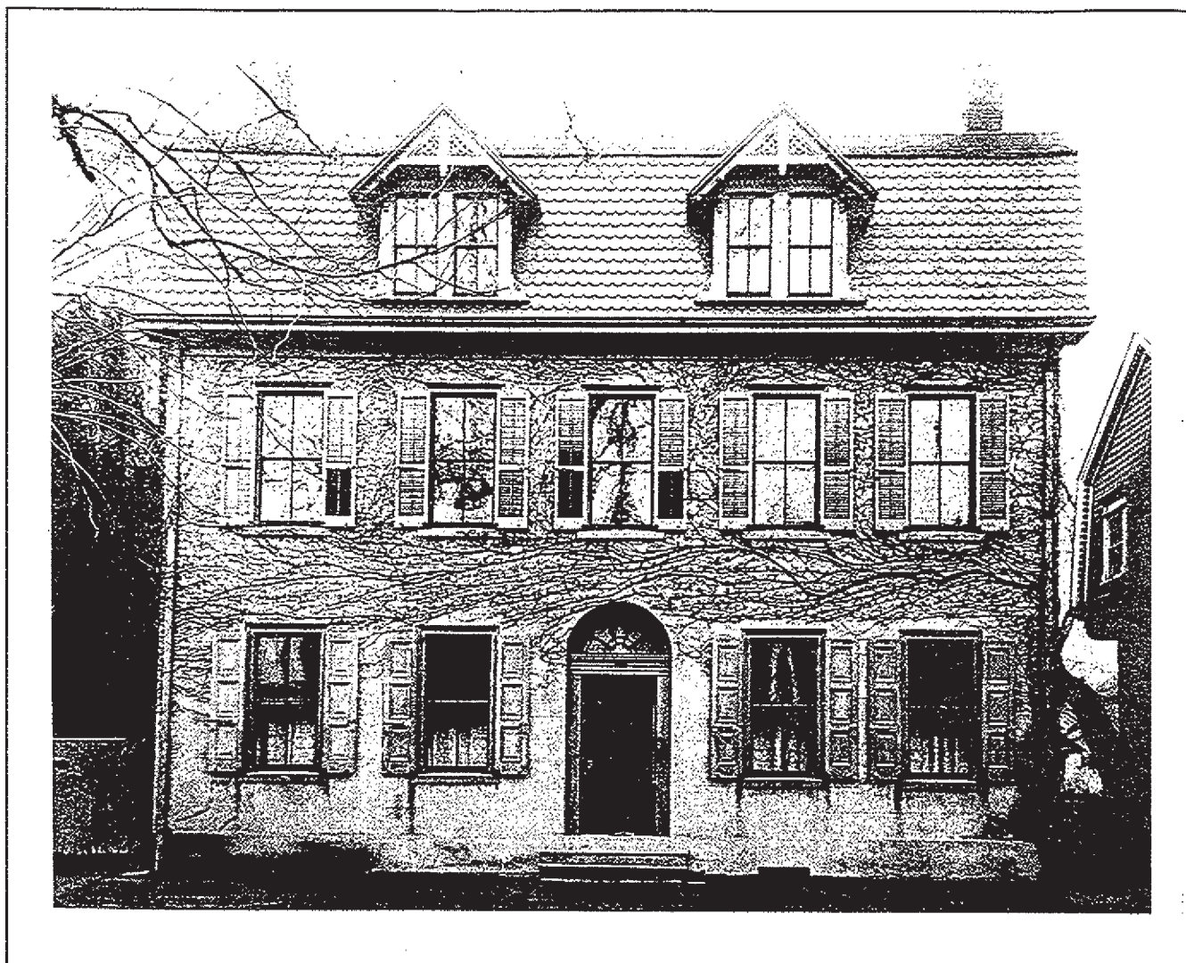
Plate 5. Historic photo showing the full east facade of the Bringhurst House as it looked in the early 20th century. This view clearly shows the full impact of the c.1895 renovation.
