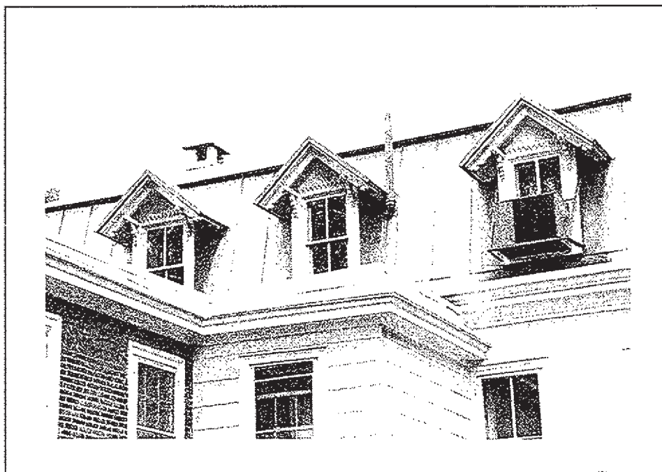
Plate 9. A detail of the c.1895 dormer windows surviving on the rear of the main roof.
