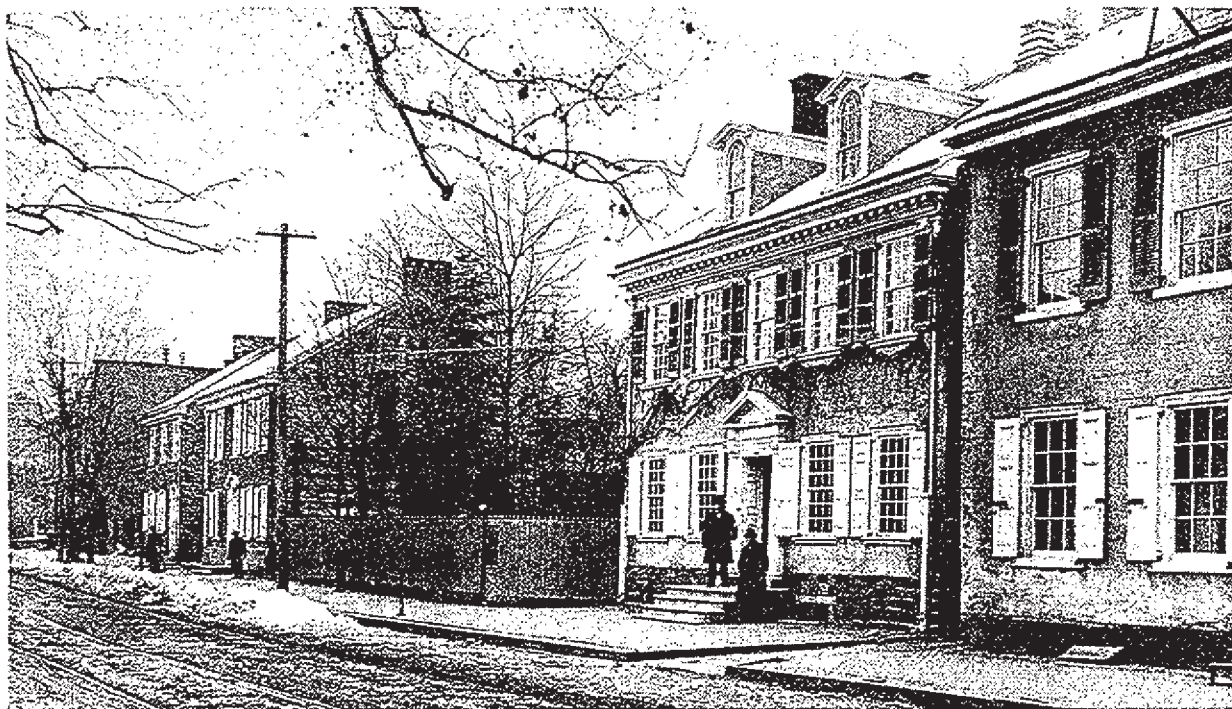
Plate 4. Historic photo showing a portion of the east facade of the Bringhurst House as it looked c.1887. Note the scored stucco on the east wall and the six over six window sash.
