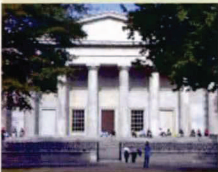
South facade of the building as it stands today.
