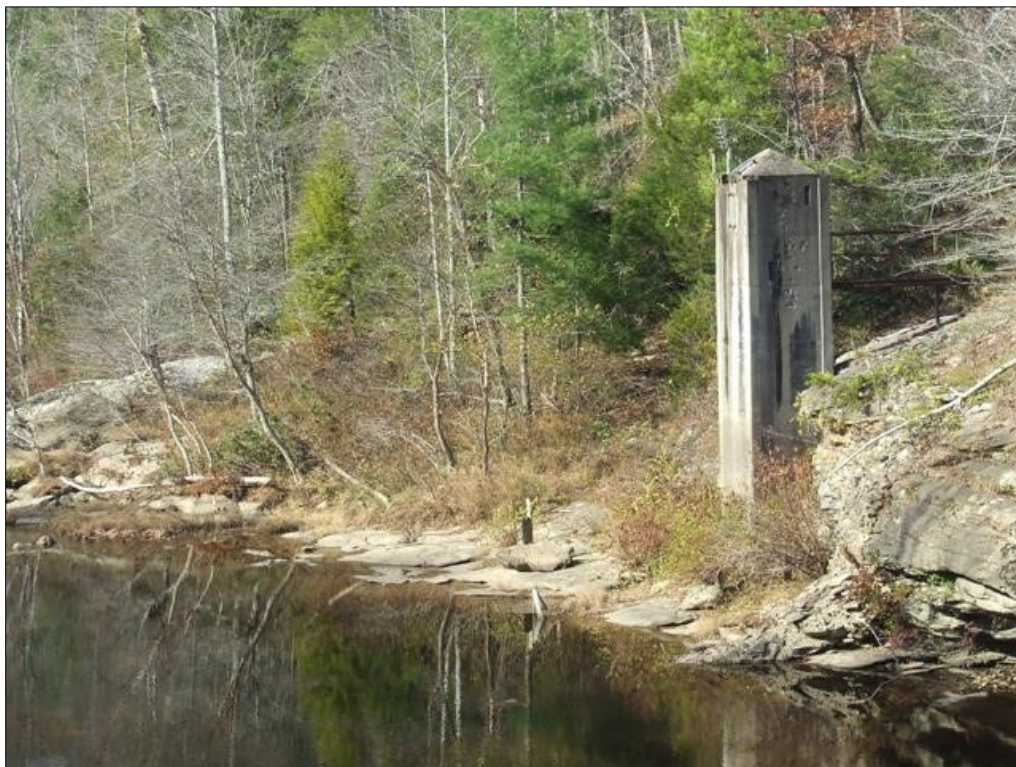
Figure SOP 6-2. USGS 03409500: Clear Fork near Robbins stilling tower.
