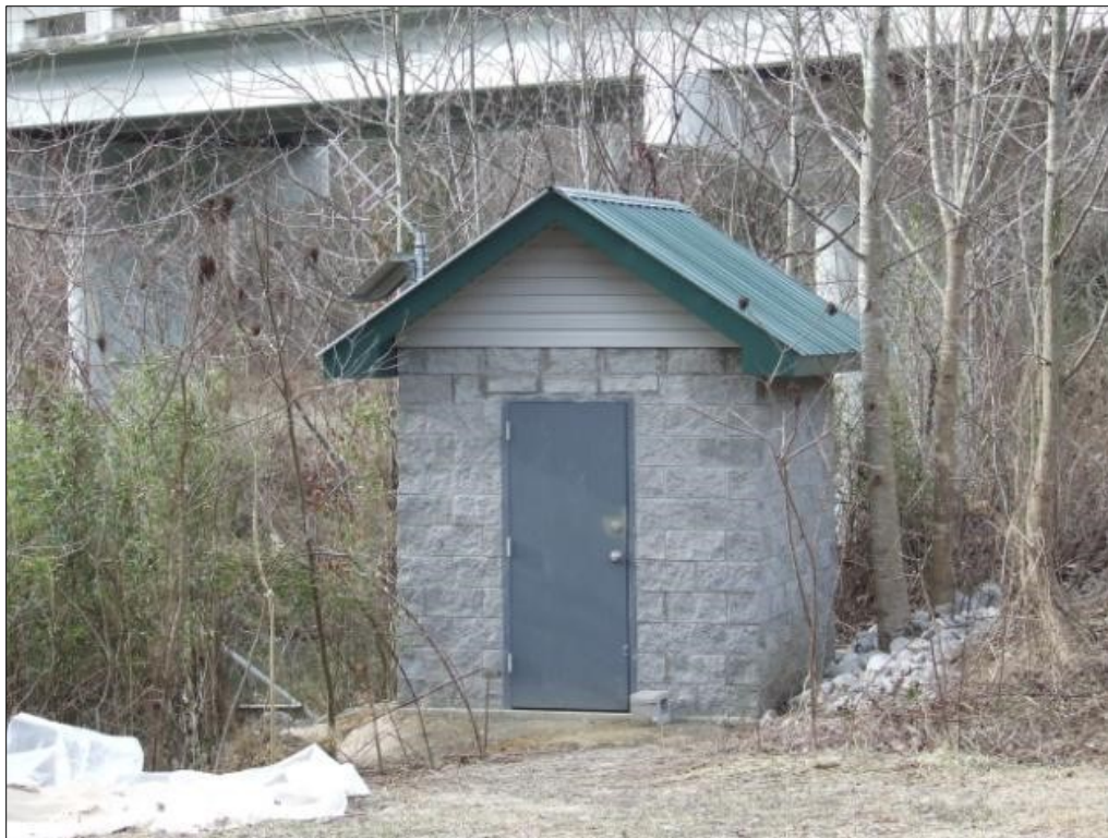
Figure SOP 6-1. USGS 03538830: Obed River at Adams Bridge gage housing.
