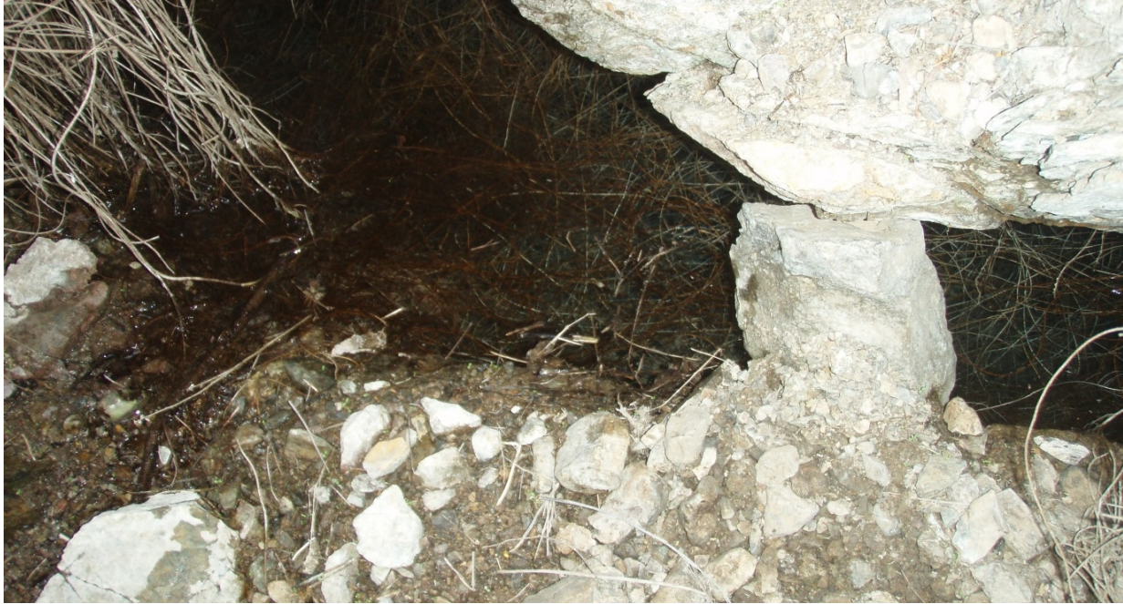
Figure 19. Diversion structure at Cornfield Spring. Photo by MOJN Field Crew.
