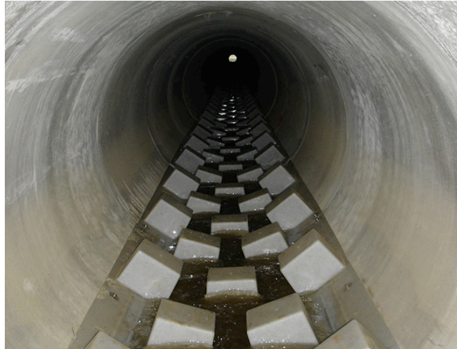
Baffles inside culvert
