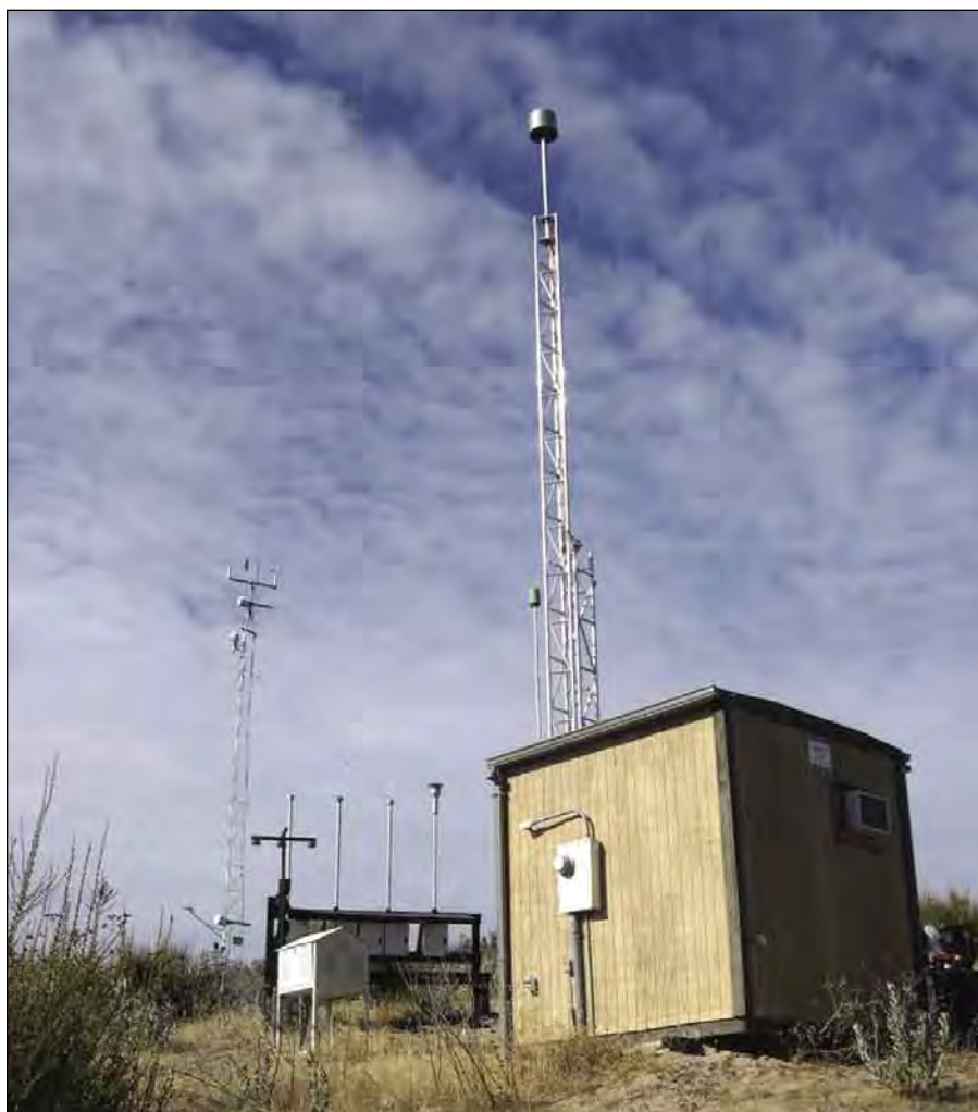
Pinnacles NM Ambient Air Quality Monitoring Station
