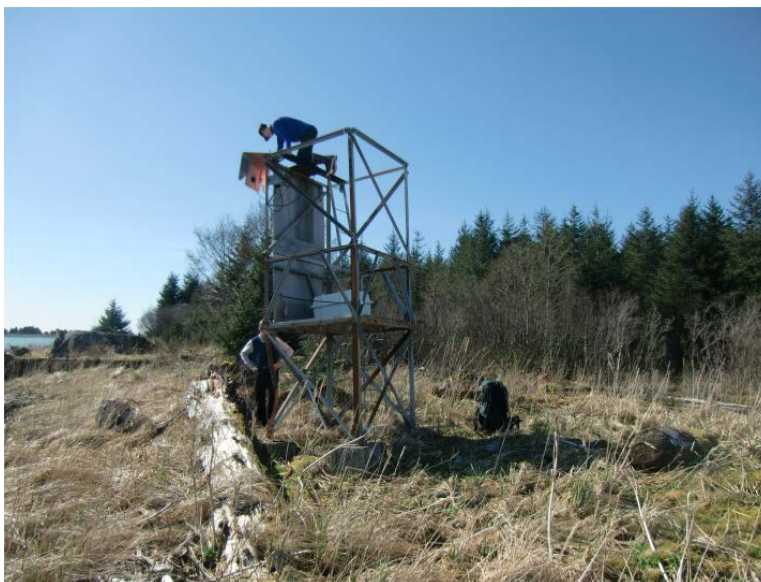
View of front (seaward) marker at Lituya Bay showing support structure and existing equipment.
