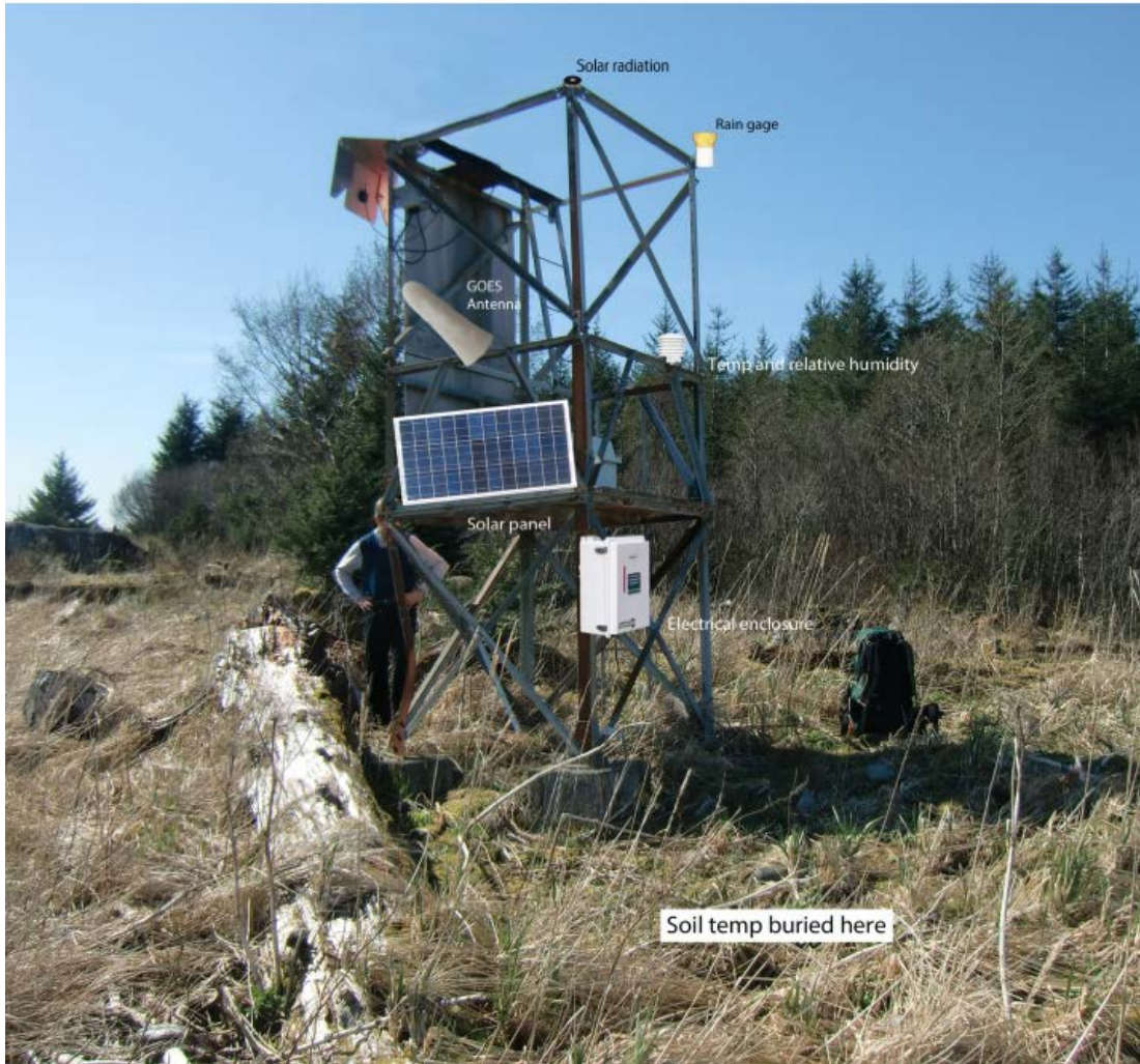
View of front (seaward) marker at Lituya Bay with approximate installation locations of proposed weather monitoring equipment. Sensors visible from this viewing angle include solar radiation, precipitation, temperature/relative humidity, and soil temperature. Additional power and communications equipment including a solar panel, satellite antenna, and equipment enclosure are also visible from this viewing angle.
