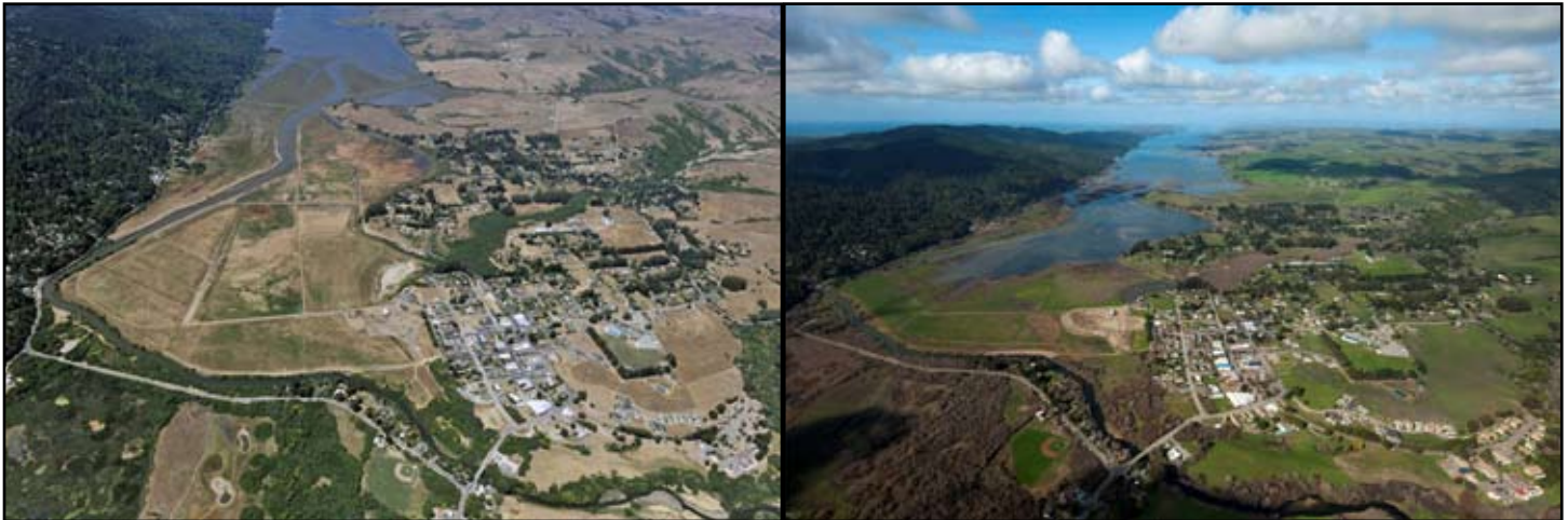
The Giacomini site in a photo taken in August 2008 before restoration (left) and in a photo taken in December 2008 after the restoration was complete (right). Photos courtesy of Robert Campbell.
