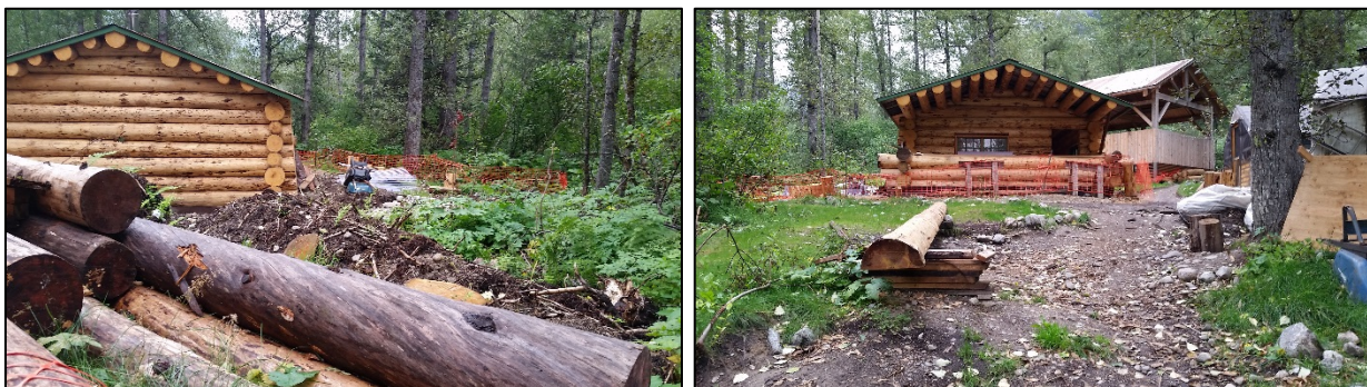
Figure 17. Disturbed areas around the new Sheep Camp warming cabin
