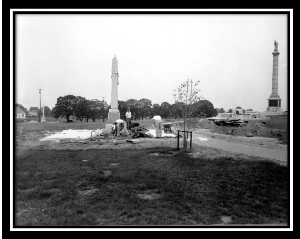
Figure 31: 20 th New York pad installation July. Antietam National Battlefield Archives 1963 Photograph 133.
