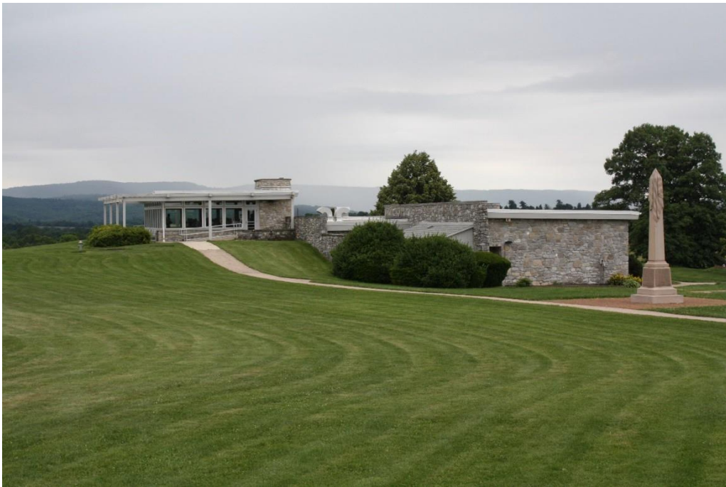
Figure 24: East elevation of the Visitor Center looking south and west (NCR CLP 2018).
