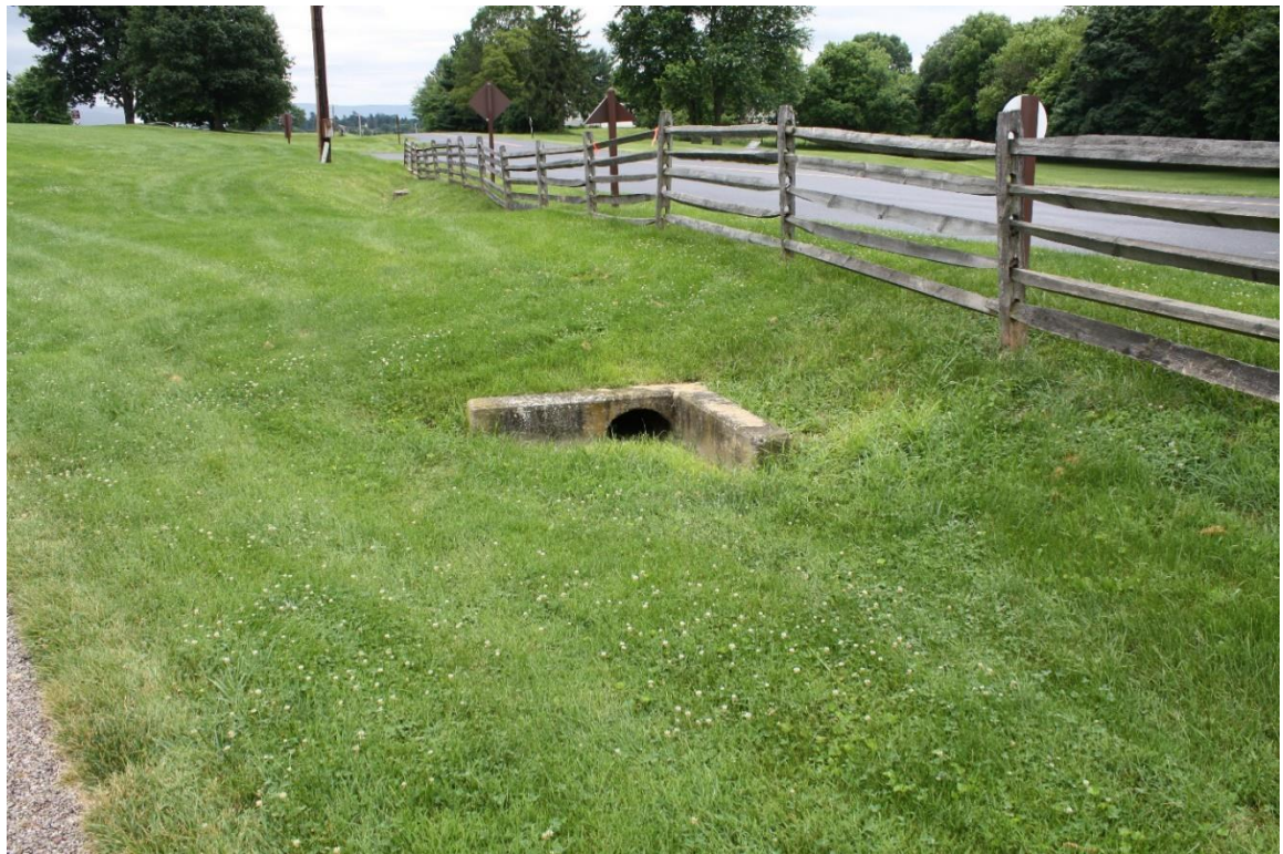
Figure 41: An example of a culvert and the post and rail fence in the study area (NCR CLP 2018).
