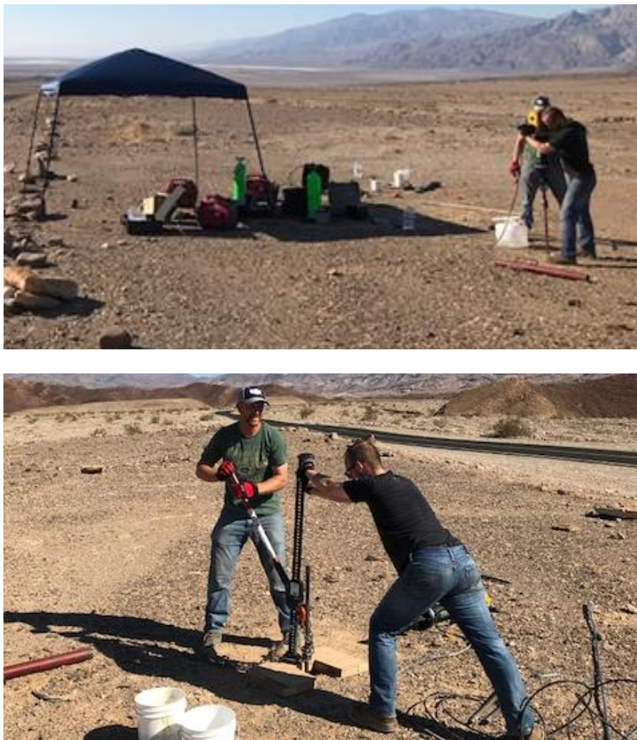
Figure 2. Installation and extraction using Geoprobe® rod and jack
