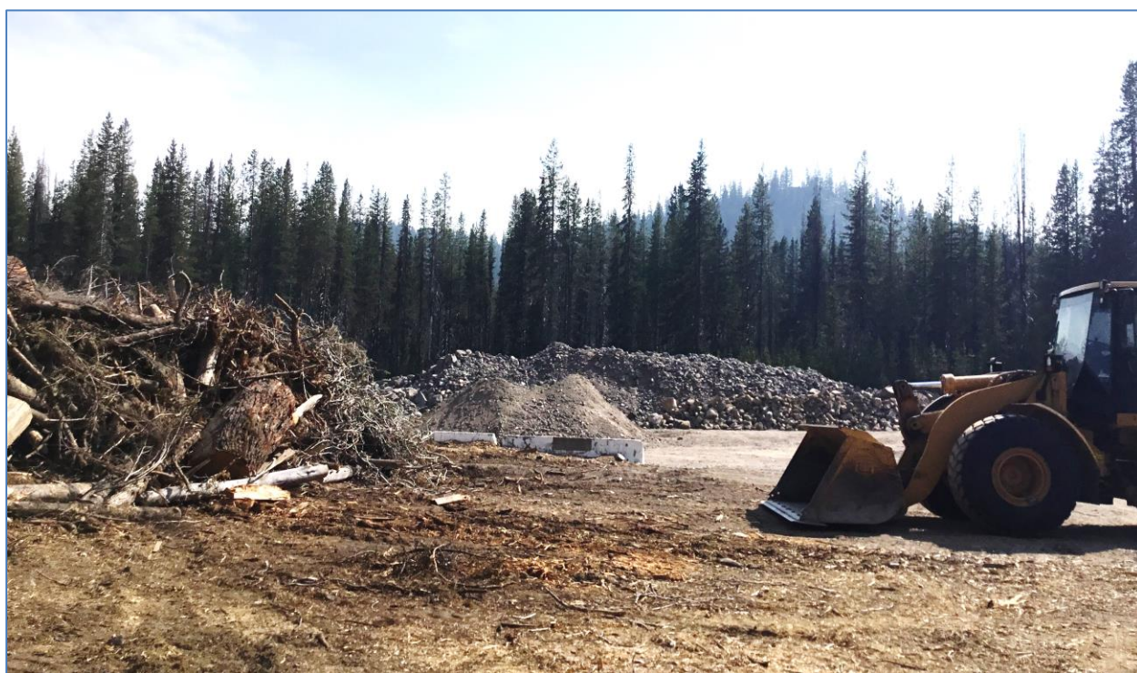
Figure 17. Materials stored for later use at the Pole Bridge Creek Quarry. Photo by Jen Hooke.
