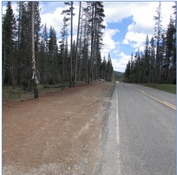
Figure 1. Heavy roadside disturbance along Highway 62. Photo by Jen Hooke.
