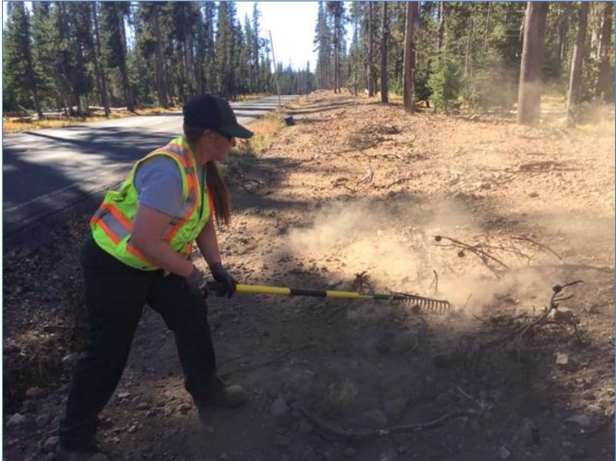
Figure 8. Raking in hand-broadcast seed mixes along Highway 62. Photo by Carrie Wyler.
