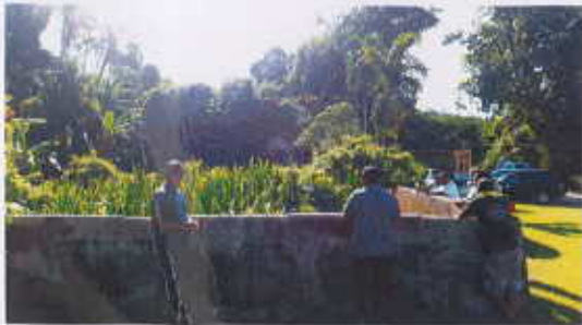
Site Cleaning at Japanese Water Pump, Koror
