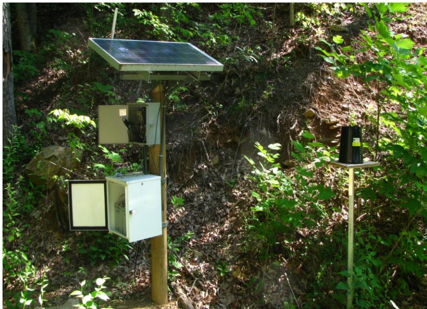
Figure 17. Station setup at HH showing solar panel, equipment boxes, and rain gauge.
