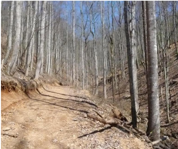
Figure 30. Road cut alongside Hembree Hollow stream within the Foothills Parkway monitoring area.
