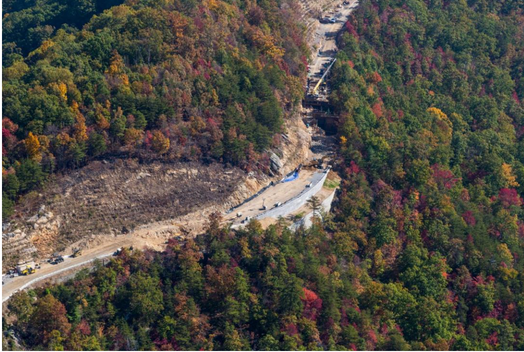
Figure 4. Aerial photo of Foothills Parkway construction highlighting land disturbance activities. (Photo Credit: Great Smoky Mountains National Park Service)
