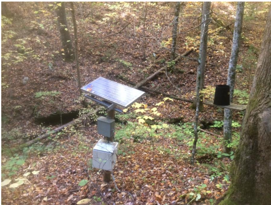
Figure 14. Dunn Hollow monitoring station at the Foothills Parkway stream monitoring site.
