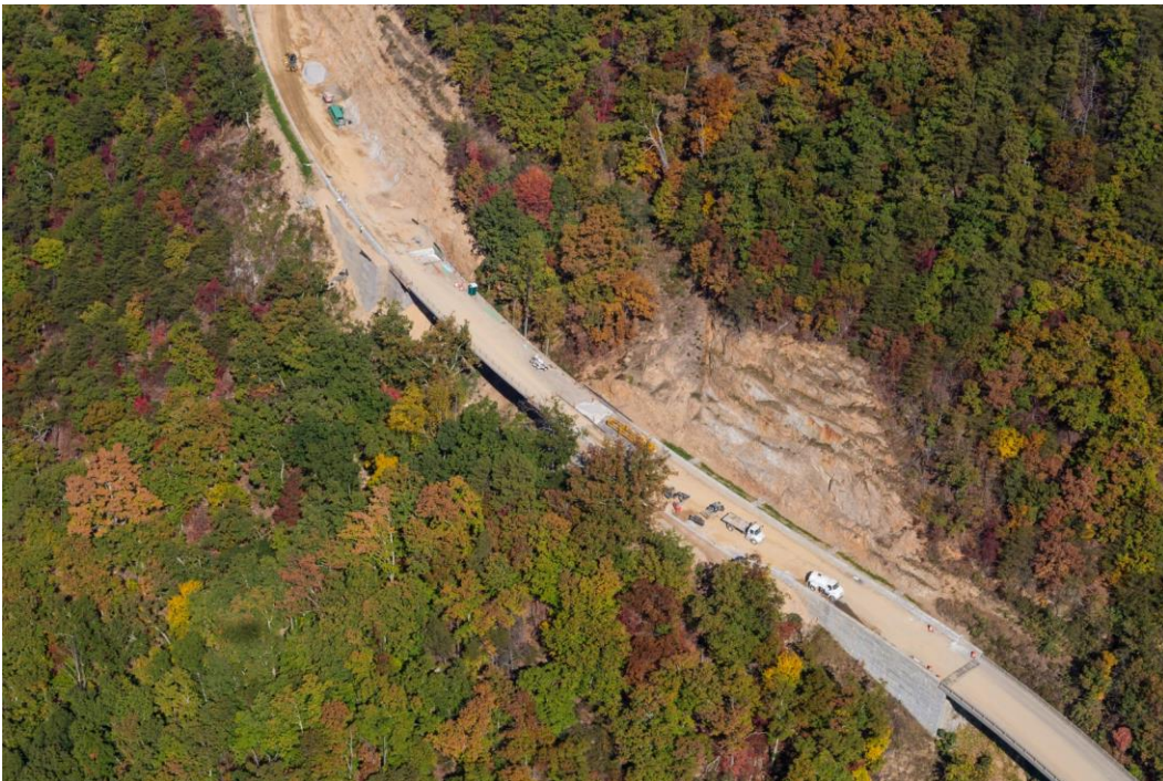
Figure 3. Aerial Photo of Foothills Parkway construction of Bridge 3. (Photo Credit: Great Smoky Mountains National Park Service).
