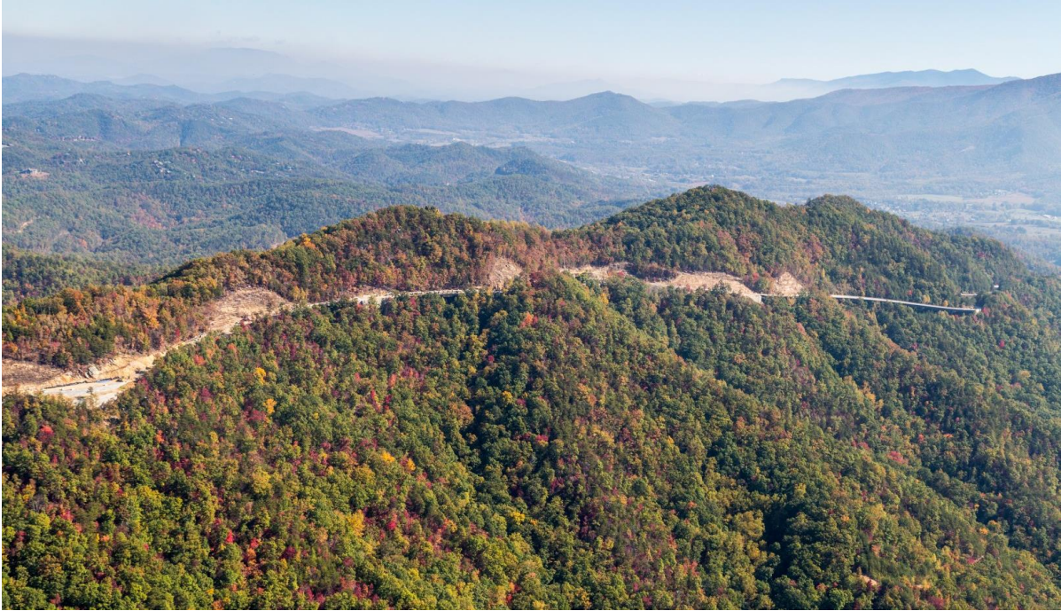
Figure 2. Aerial image of Foothills Parkway construction. (Photo Credit: Great Smoky Mountains National Park Service).
