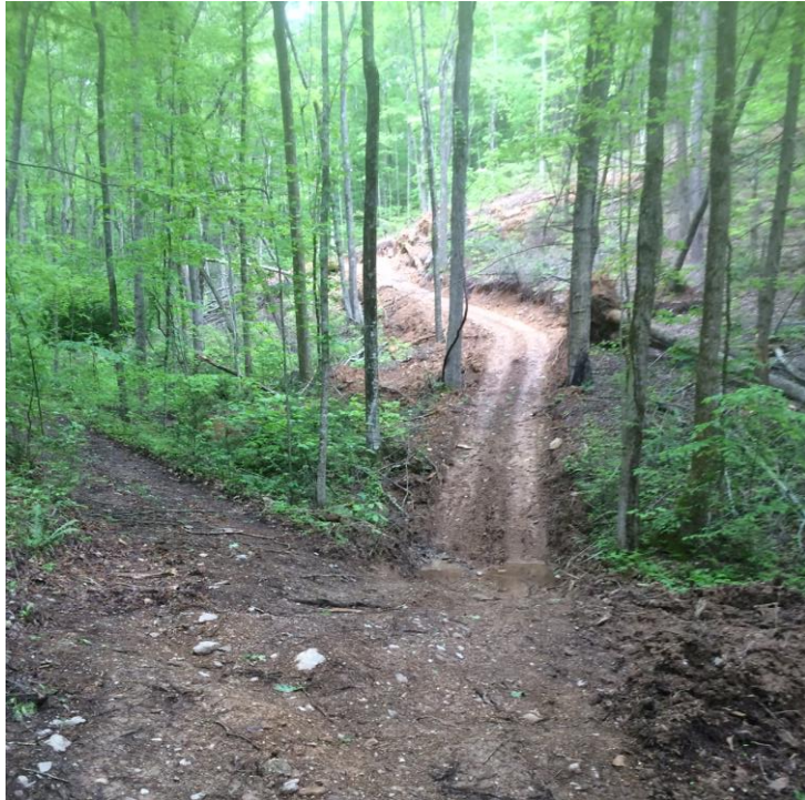
Figure 32. New road cut across Rudd Hollow stream within the Foothills Parkway monitoring area.
