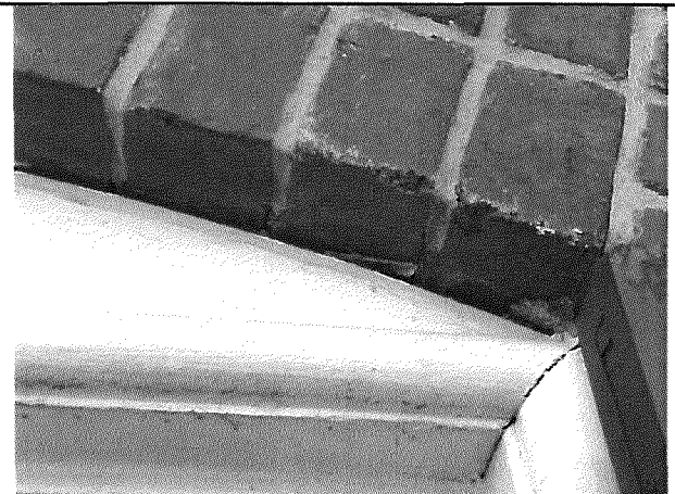
6. View of the window caulk (ACM), Sample No. 4.
