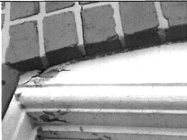
5. View of the window caulk (ACM), Sample No. 3.
