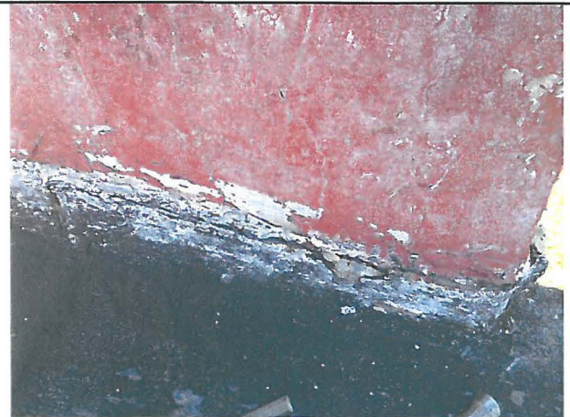
4. View of the chimney flashing (ACM), Samples 7-8.
