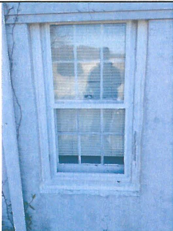
5. Typical view of the window.
