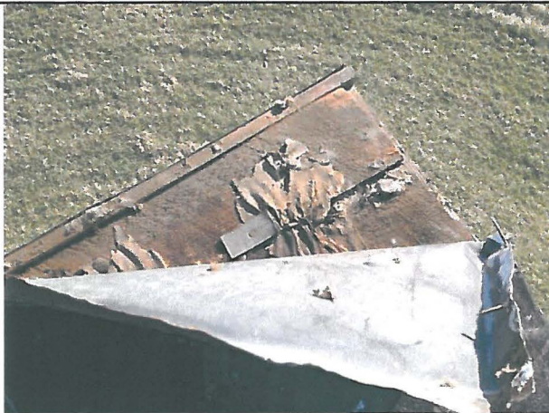
3. View of the paper membrane beneath the metal roof.
