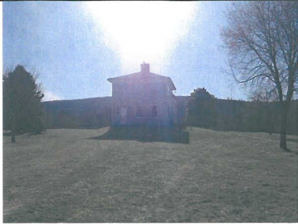
1. View of the Murphy Farm House, and front upper roof.
