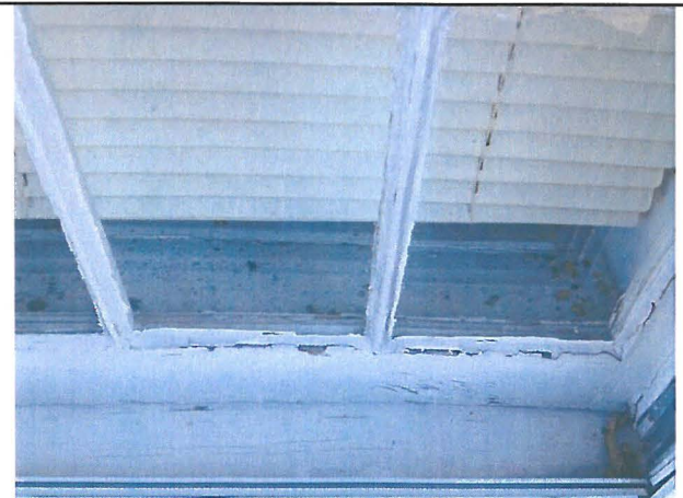
6. Typical view of the window glazing.
