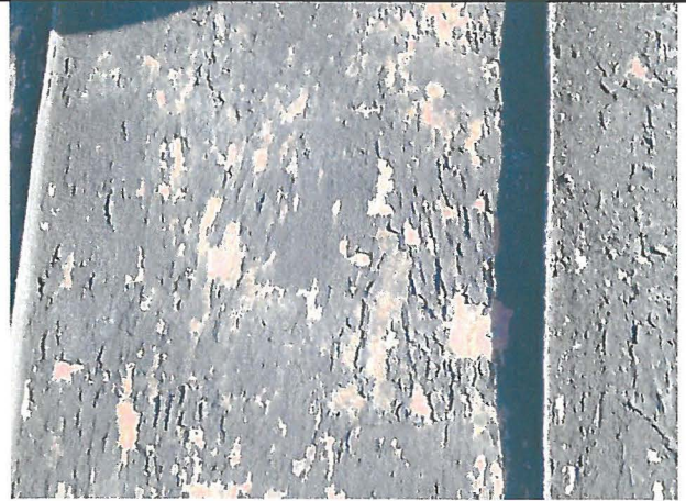
2. View of the lower metal roof with black membrane (ACM), Samples 1-2.
