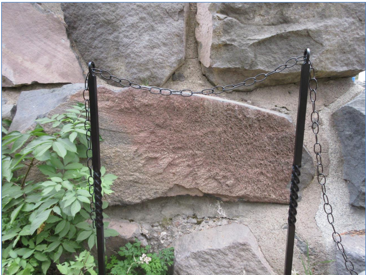
Figure 10. The new fence posts and chain for the Replace Rim Village Barriers project. Photo by Carrie Wyler.
