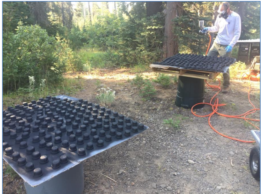
Figure 6. Painting caps for fence post receivers. Photo by Carrie Wyler.
