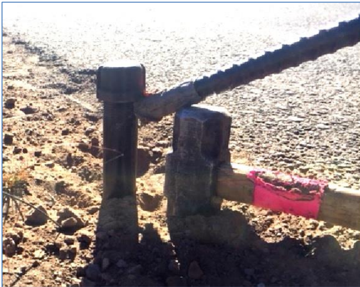
Figure 12. Using a cap as a lever point to remove a post receiver. Photo by Carrie Wyler.
