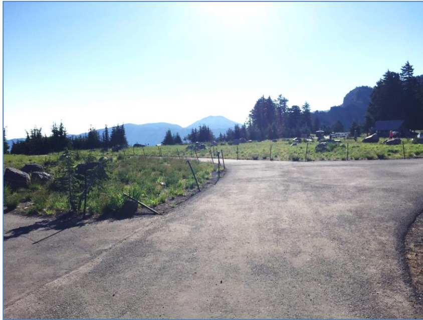
Figure 2. The old fencing was prone to leaning and/or falling over, as it was lightweight and easily dislodged, and its rebar stake supports were difficult to install in the compacted ground. Photo by Carrie Wyler.
