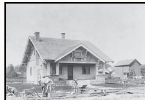
Green House built 1910
