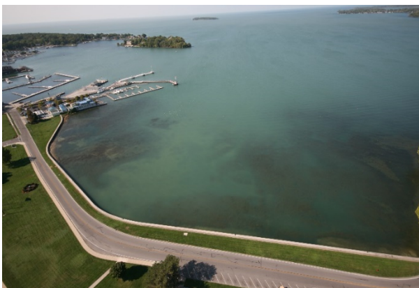
Figure 4-16: Put-in Bay and the expanse of Lake Erie as seen from the observation platform. CHG
