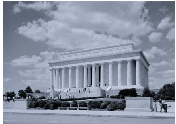
Figure 35. The Lincoln Memorial, 1976. (Source: Historic American Building Survey, HABS DC-3-2)
