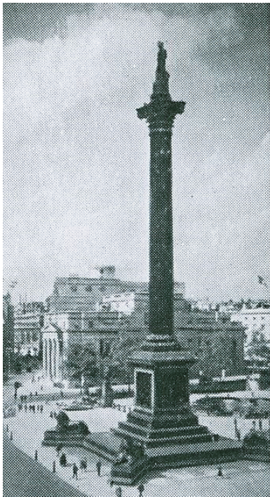
Figure 21. Nelson's Column, undated photograph. (Source: The New York Public Library Digital Collections.)
