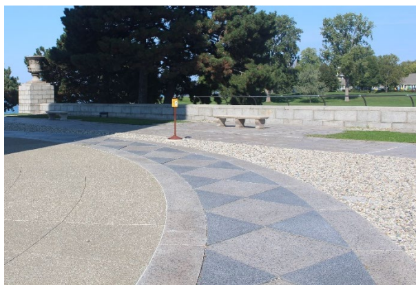
Figure 2-16: Granite pavers installed by the NPS in 1983–1984. To the left is the scored concrete band installed to replace the brick in 2012. CHG
