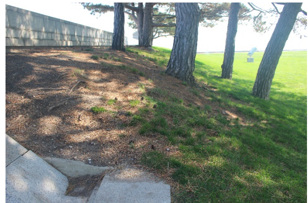
Figure 2-4: Area of erosion of the earthen berm under the Austrian pines. CHG
