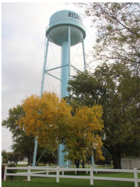
Water tower in Rising City, BU13-030.
