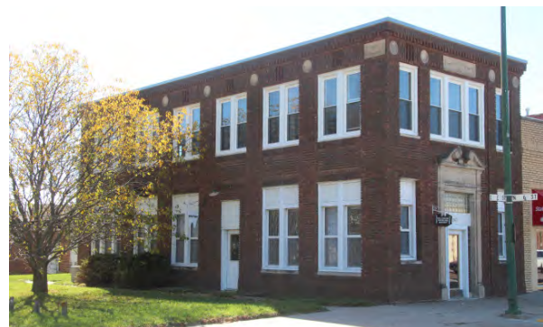
The Telephone Building in David City, BU05-028.
