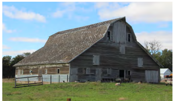
Barn near Rising City, BU00-216.
