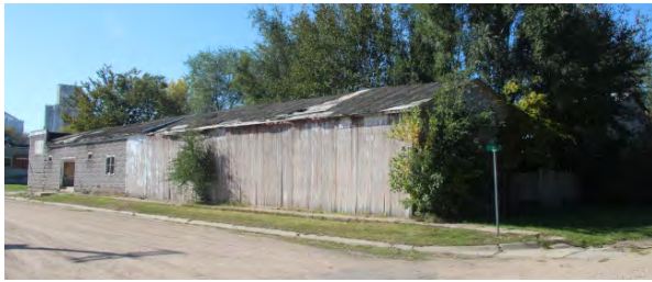
Ulysses Lumber Company complex, BU15-036.
