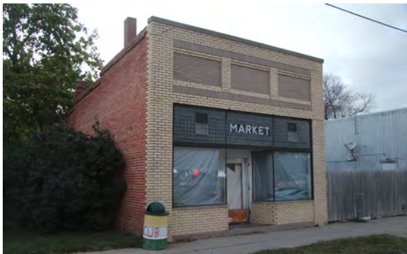
Commercial Building in Dwight, BU06-007.
