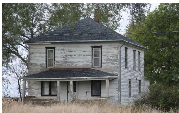
American Foursquare near Garrison, BU00-200.
