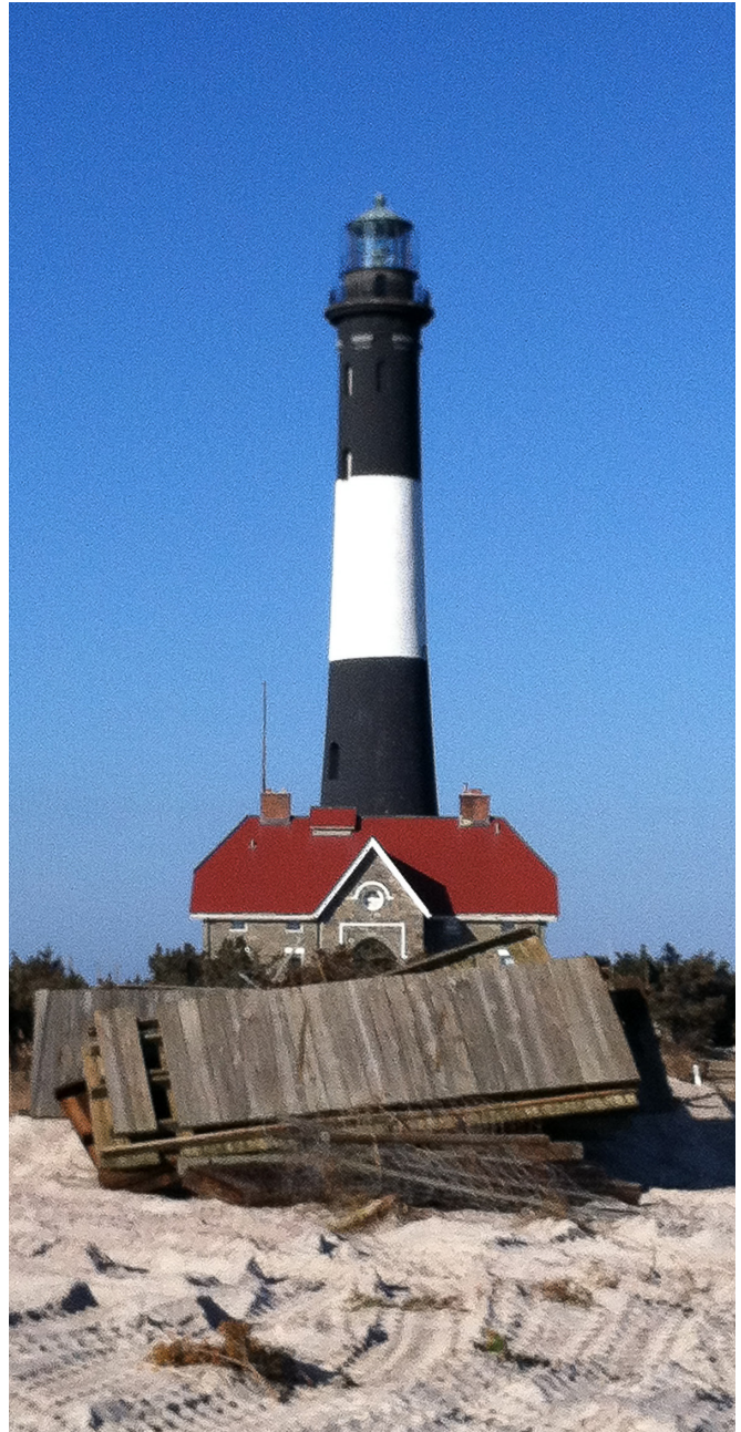
Damaged Boardwalk stacked for salvage and removal at Fire Island Lighthouse. Photo by NPS/Budzinski
