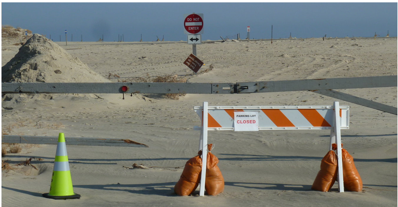
The entrance of a parking lot at Gateway National Recreation Area's Sandy Hook Unit is blocked off after the storm moved sand from the beach onto it's surface. Photo by NPS/Lynch
