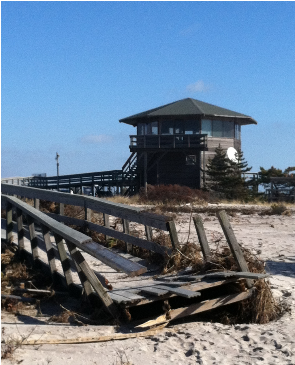
Fire Island's Wilderness Visitor Center and damaged boardwalk, post-Hurricane Sandy. Photo by NPS/Budzinski
