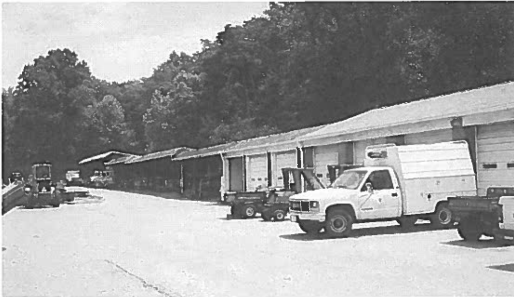
Figure 56 – East end of Maintenance Building, with extensions. (Robinson & Associates, Inc., July 28, 2005.)
