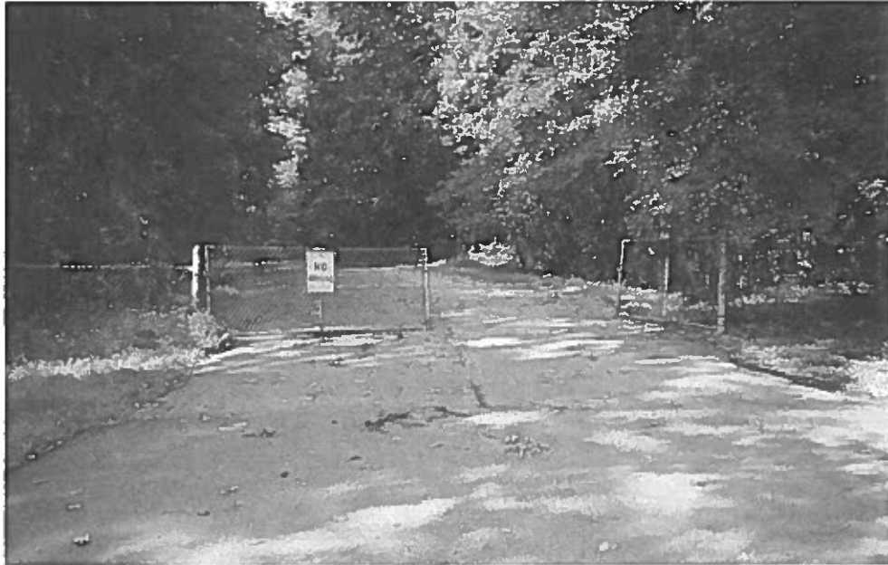
Figure 44 – Vehicle barrier along Park Central Road, south of the campground road. (Robinson & Associates, Inc., July 28, 2005.)
