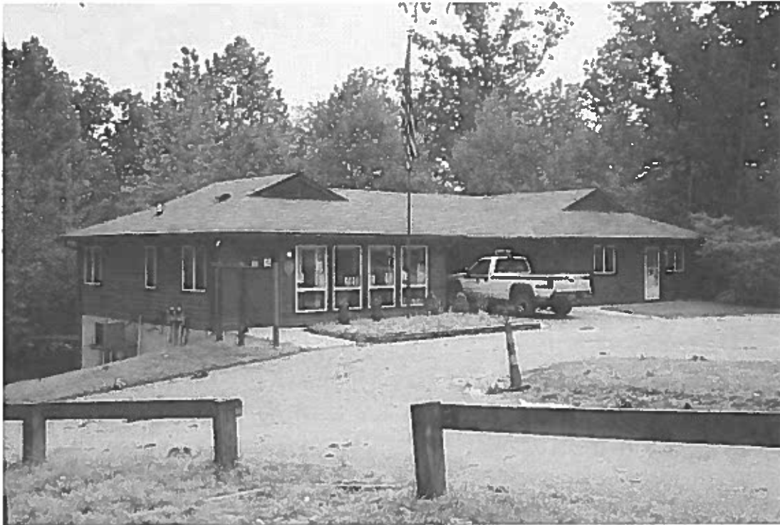
Figure 48 – Ranger Station. (Robinson & Associates, Inc., July 28, 2005.)
