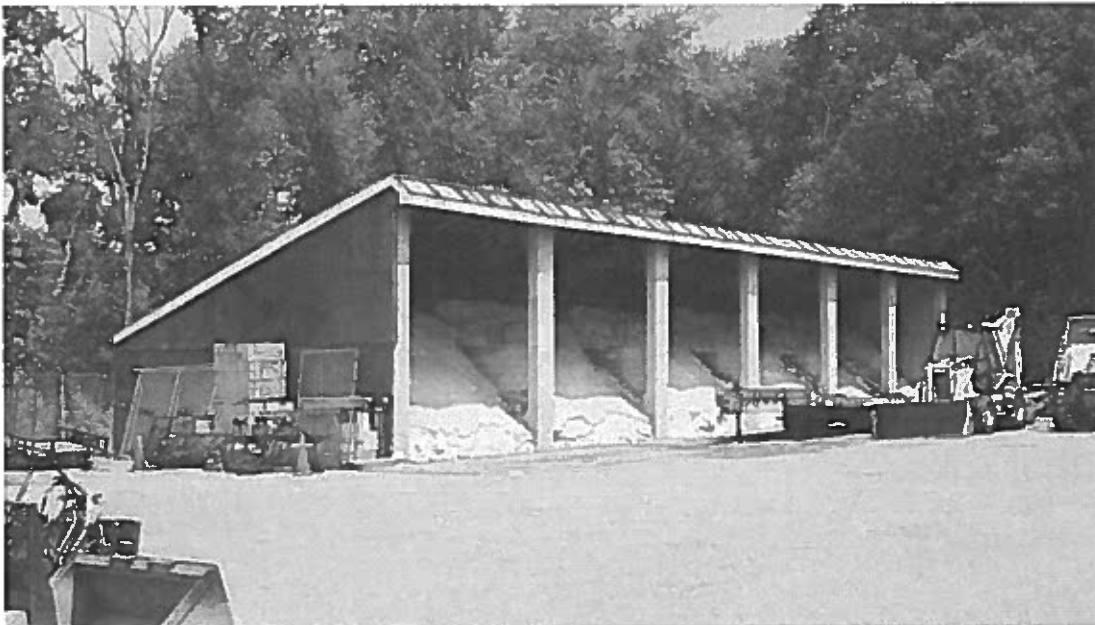
Figure 49 – Salt Shed. (Robinson & Associates, Inc., July 28, 2005.)
