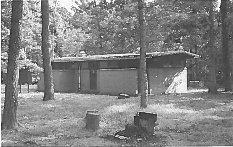
Figure 29 – Current view of Comfort Station, C Loop. (Robinson & Associates, Inc., July 28, 2005.)
