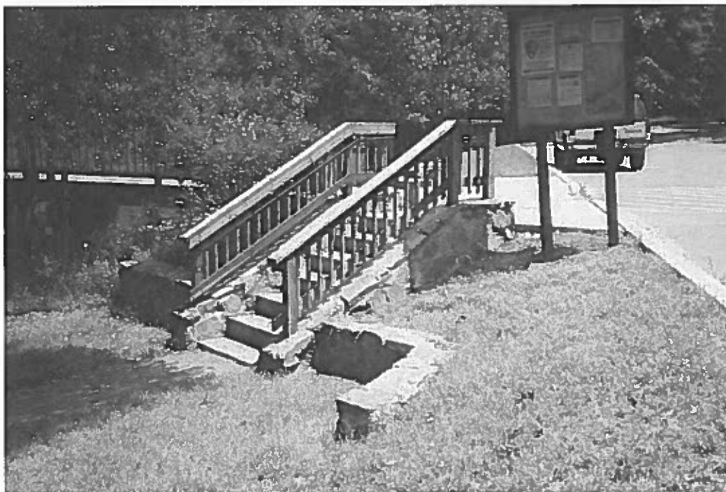
Figure 51 – Stair in front of Park Headquarters. (Robinson & Associates, Inc., July 28, 2005.)
