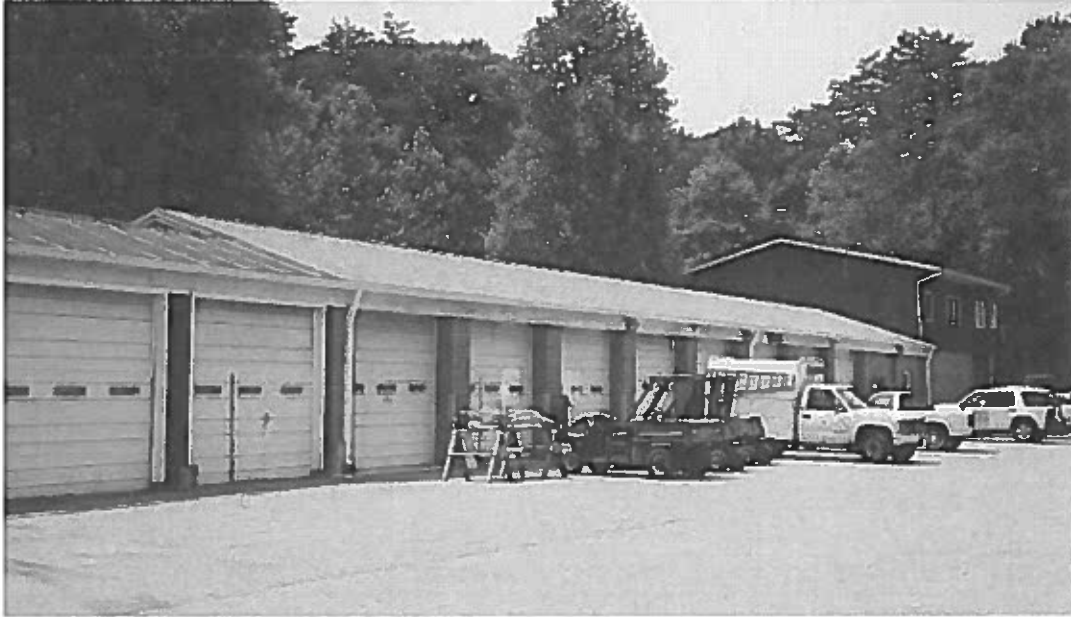
Figure 23 – Current View of original eight-bay Maintenance Building, located at the center. (Robinson & Associates, Inc., July 28, 2005.)
