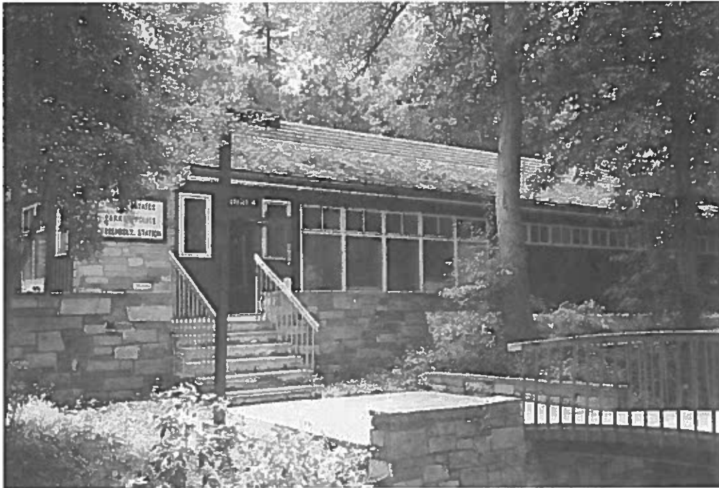
Figure 54 – Park Police Station. (Robinson & Associates, Inc., July 28, 2005.)
