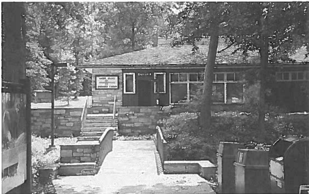
Figure 24 -- Current view of Park Police Station entrance. (Robinson & Associates, Inc., July 28, 2005.)
