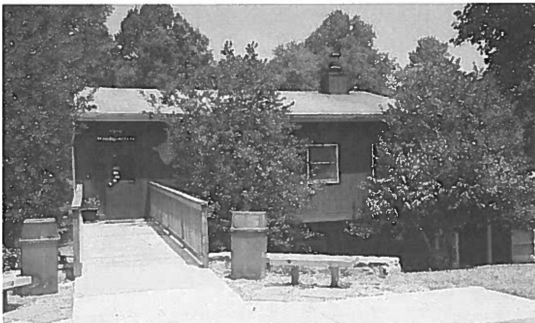
Figure 50 – Park Headquarters. (Robinson & Associates, Inc., July 28, 2005.)
