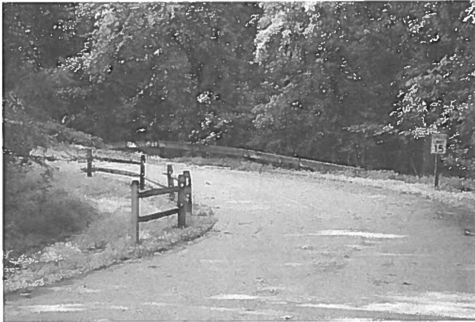
Figure 30 – Campground Road near C and D Loops. (Robinson & Associates, Inc., July 28, 2005.)
