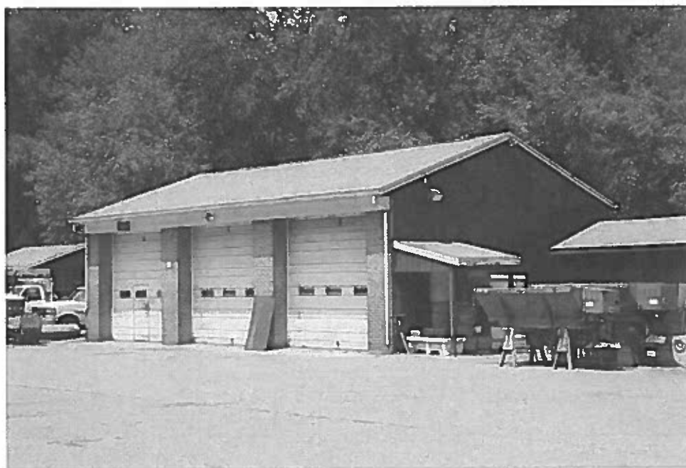
Figure 37. Current view of Auto Shed, looking northwest. (Robinson & Associates, Inc., July 28, 2005.)
