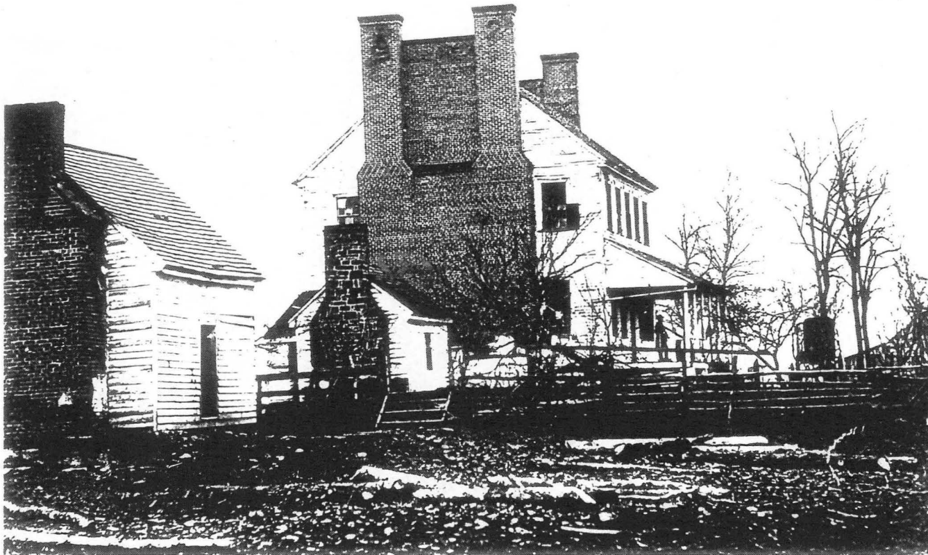
Fig. 3. "Portici" plantation mansion, 1862. Portici, one of the most impressive houses in the region, had descended in the Carter family. Frank Lewis was the owner at the time of the Civil War. Courtesy U.S. Army Military History Institute, Carlisle, Pa.
