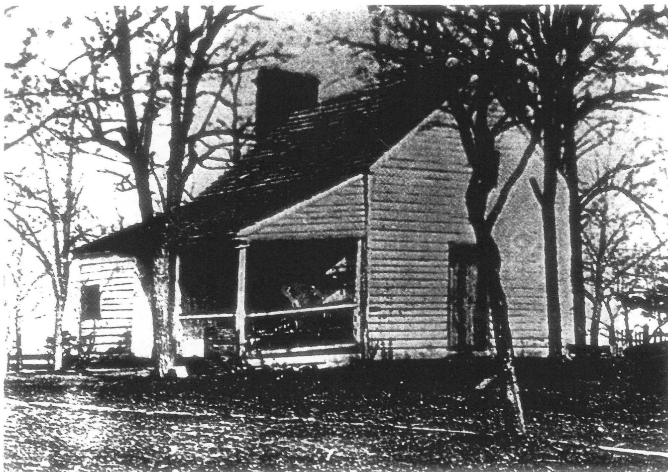
Fig. 1. James Robinson house, near the intersection of the Warrenton Turnpike and the Manassas-Sudley road (see Map, detail), 1862. "Gentleman Jim" Robinson was one of the most prosperous free blacks in the area before the Civil War. The house was enlarged after the Civil War, probably with the proceeds from Robinson's award from the Southern Claims Commission. Library of Congress collection, courtesy of the Manassas National Battlefield Park Library, Manassas, Va.
