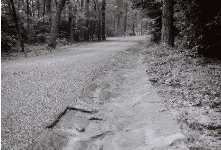
Figure 53. Stone gutters lining the gravel roadway in the Ridge Picnic Area (Robinson & Associates, Inc., August 7, 2003).
