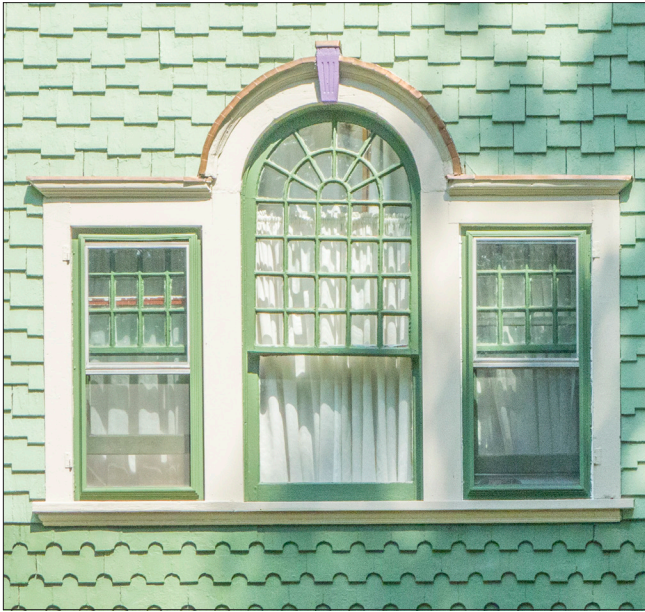
This tripartite window configuration, with multi-light upper sashes and central arch-headed sash, is a character-defining, historic feature. A Certificate of Appropriateness application for changes to windows must be submitted for BHAR review prior to the commencement of work.
