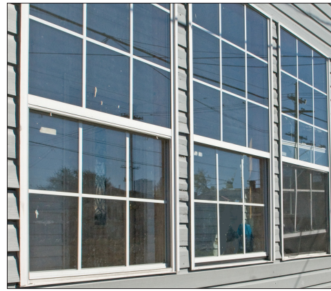
Vinyl windows with applied muntins lack the profiles and details of traditional wood windows and are not appropriate at historic buildings. They are also mounted flush to the outside wall without trim or casings.
