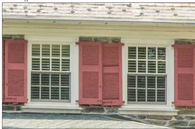
Half-screens installed at only the lower sash limits concealment of the historic windows provided the screen rails align with those of the historic windows.
