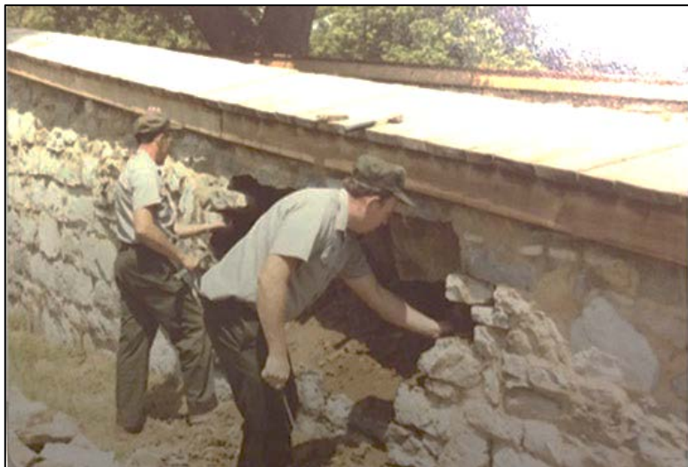
Figure 39. Maintenance workers repair the outer face of the spandrel wall in 1980. Photo: Antietam National Battlefield archives images.
