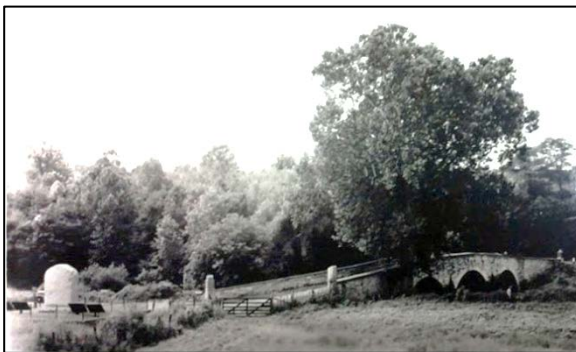
Figure 23. Photograph taken by W.H. Sheffield in 1940. View looking southwest toward the bridge. Memorials can be seen on the bridge. Photo: Antietam National Battlefield archives images.
