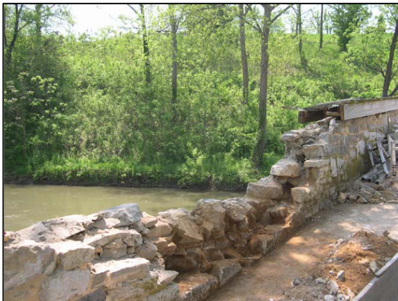
Figure 49. Looking southwest, the damaged masonry was removed down to sound material. Photo: NPS DSC eTIC No. ANTI 302 C10.
