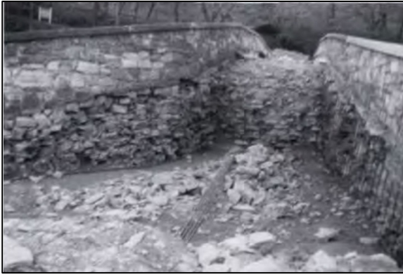
Figure 28. The 1955-56 work, seen above, included removing the fill above the arches, placing reinforcing bars against the spandrel walls. Note the condition of the back of the spandrel wall. Photo: Peck Peck & Associates and McMullan & Associates Pre-Design Bridge Composition & Analysis report, 2014.
