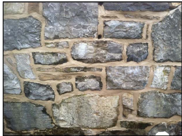
Figure 57, above. After pointing is completed. Photo: NPS DSC eTIC No. ANTI 302 127626.
