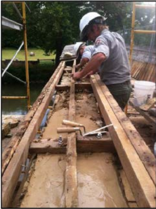
Figure 58. Installation of mortar wash atop stone parapet wall. Photo: NPS DSC eTIC No. ANTI 302 127626.
