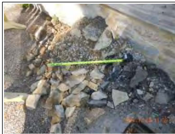
Figure 68. Fill material from the test pit behind the west abutment. Note the size of the stones. Photo: 2014 Pre-Design report.
