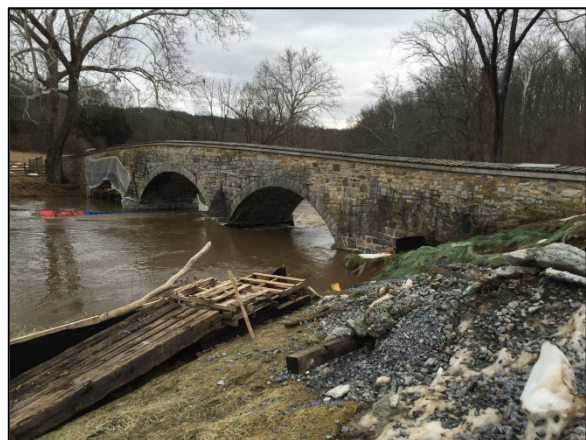
Figure 74. The north elevation of the three-span Burnside Bridge from the west bank with Antietam Creek flowing underneath and through it. Photo: HPTC, 02/25/16.
