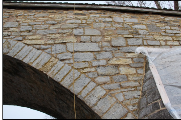
Figure 82. Voussoirs ring the arch. Photo: HPTC, 01/20/16.
