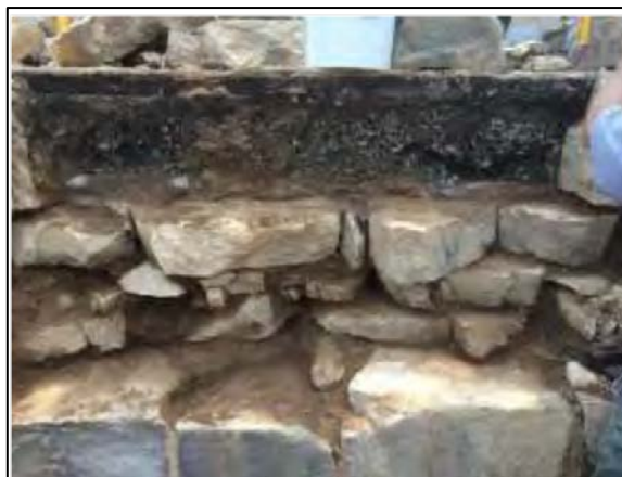
Figure 70. The stones below the asphalt and gravel are part of the spandrel wall. Note the smaller stone used to pin the larger stone overlaps between the wythes. Note also the lack of mortar. Photo: 2014 Pre-Design report.
