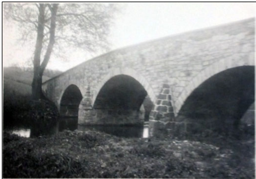
Figure 26. Photograph from 1947 of the repointing completed by Boonsboro contractor B.L. Smith. Photo: Antietam National Battlefield archives images.
