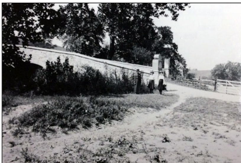
Figure 21, right. Photograph of Mrs. Fred Cross and her daughters, Dorothy and Bertha, from South Royalston, Massachusetts on June 16, 1919. The bridge now has concrete coping on top of the parapet walls. Photo: Antietam National Battlefield archives images.
