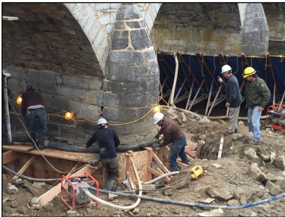
Figure 77. The two piers project from the face of the bridge spandrel walls and are rounded to ease water flow under the bridge. A footing is being poured around each pier during the current rehabilitation project. Photo: HPTC, 11/18/2015.
