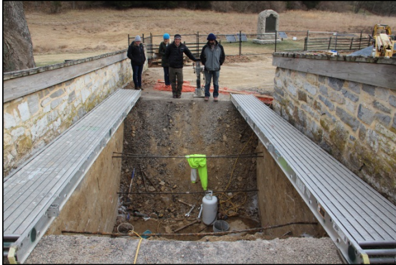
Figure 75. Fill was removed from between the spandrel walls during the currently ongoing rehabilitation project. Photo: HPTC, 01/20/16.
