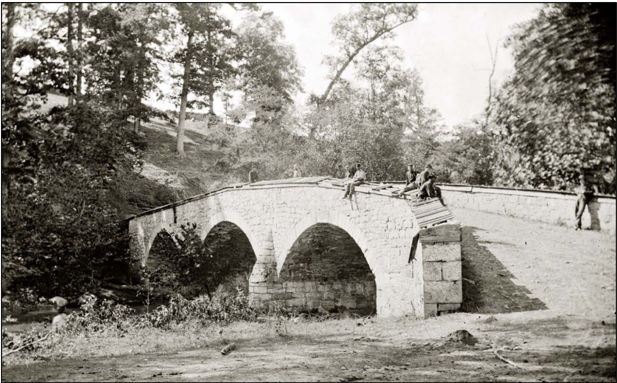
Figure 17. Alexander Gardner's photograph of soldiers sitting on the damaged wood coping of the bridge. This photograph is looking west across the bridge to the Confederate's position on the hill. Photo: Library of Congress, https://www.nps.gov/anti/learn/photosmultimedia/gardnerphotos.htm .
