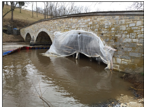
Figure 65. South elevation, from east bank, during Phase I of rehabilitation. Photo: HPTC, 02/25/16.
