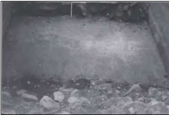
Figure 30. The 1955-56 work, seen above, included placing a concrete slab over the piers and the abutments a few feet above the springline and sloped to weep holes. Photo: Peck Peck & Associates and McMullan & Associates Pre-Design Bridge Composition & Analysis report, 2014.
