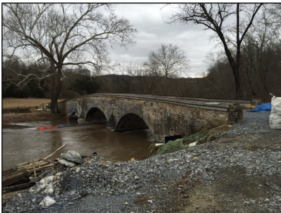
Figure 64. North elevation, from west bank, during Phase I of rehabilitation. Photo: HPTC, 02/25/16.
