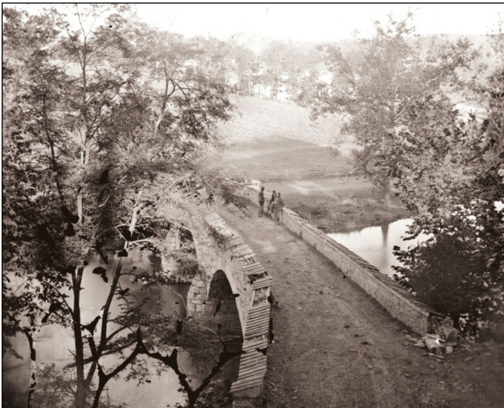
Figure 15. Alexander Gardner's photograph of Burnside Bridge after the Battle of Antietam. As can be seen, the coping of the bridge was heavily damaged, as was the southwest corner. Photo: Library of Congress, https://www.loc.gov/item/cwp2003006118/PP/ .
