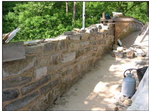
Figure 50. The stone was relaid with historic coursing and historic construction techniques. Photo: NPS DSC eTIC No. ANTI 302 C10.
