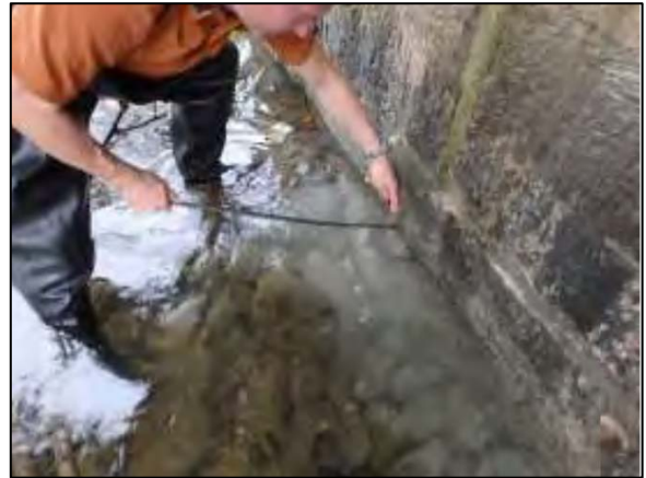
Figure 85. Probing under the East Pier with rebar that extended 2'-6" at one location. Photo: 2014 Pre-Design report.
