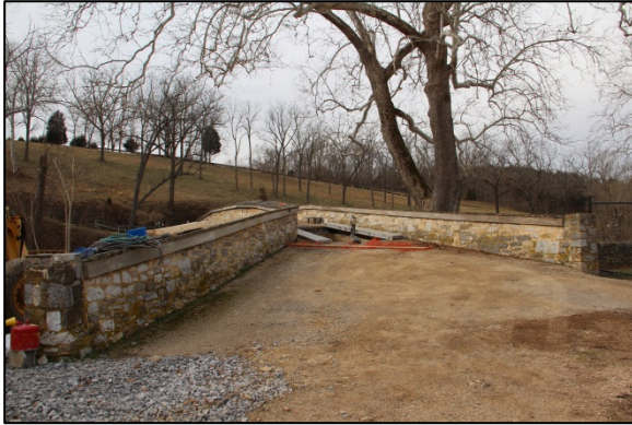
Figure 79. The south wing wall on the east bank (shown here) and the north wing wall on the west bank are splayed to accommodate turning vehicles onto the bridge. Photo: HPTC, 01/20/16.
