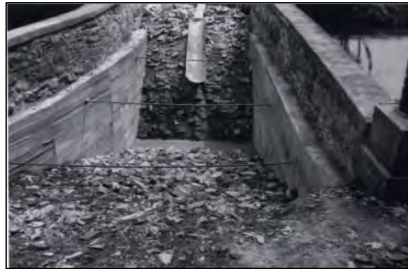
Figure 31. The 1955-56 work, seen above, included placing concrete walls against the spandrel walls with tie bars between. Note the concrete chute placed against the backside of the arch barrel stones. The walls are located over the piers and abutments do not extend to the centerline of the span. Photo: Peck Peck & Associates and McMullan & Associates Pre-Design Bridge Composition & Analysis report, 2014.
