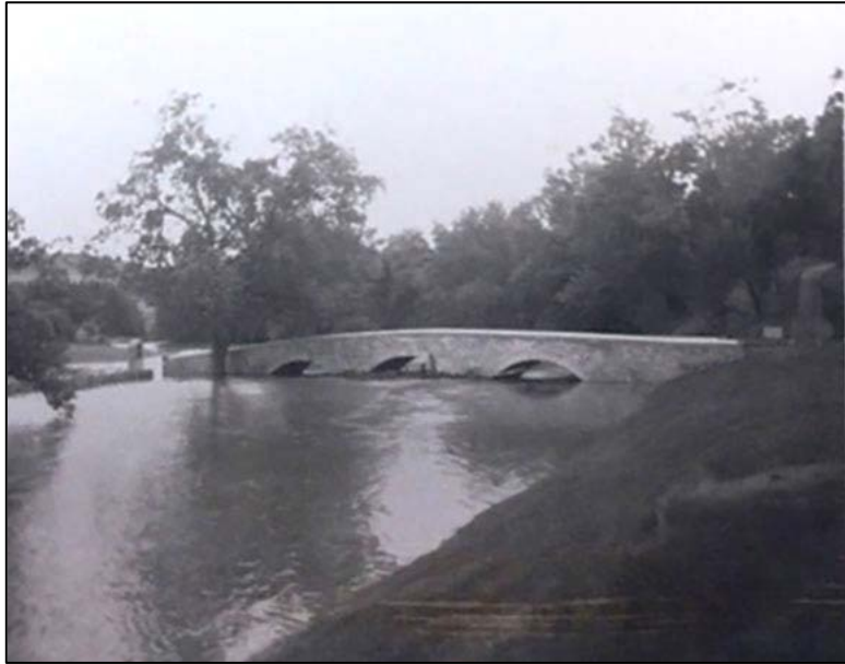
Figure 38. The creek rose during Hurricane Agnes. The bridge is partially submerged in water, as seen in this June 20, 1972 photograph. Photo: Antietam National Battlefield archives images.
