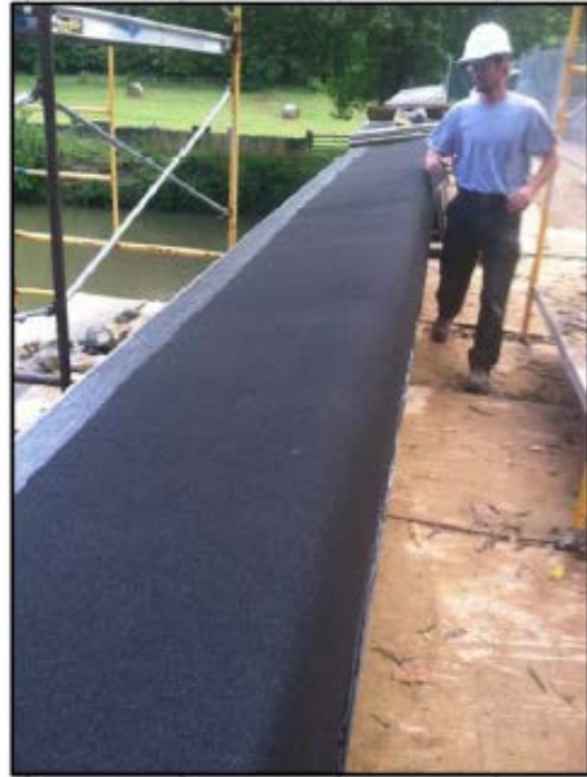
Figure 59. Installation of flashing above wood frame and below wood coping. Photo: NPS DSC eTIC No. ANTI 302 127626.
