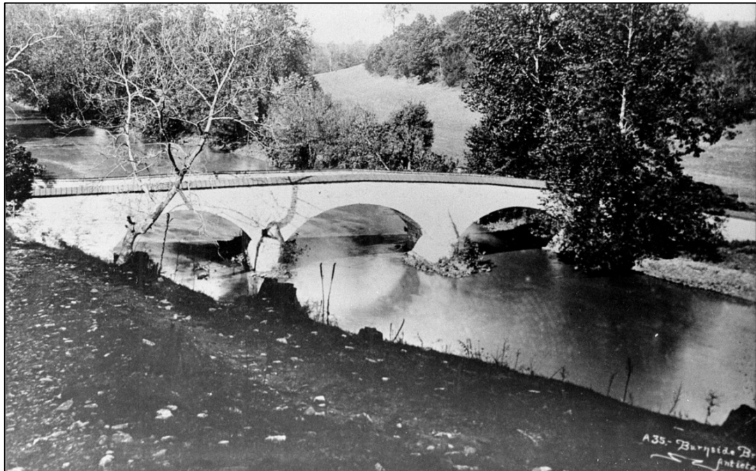
Figure 36. Photograph of Burnside Bridge taken from west bank looking north towards the bridge. Photo: NPS DSC eTIC No. ANTI 302 D15.
