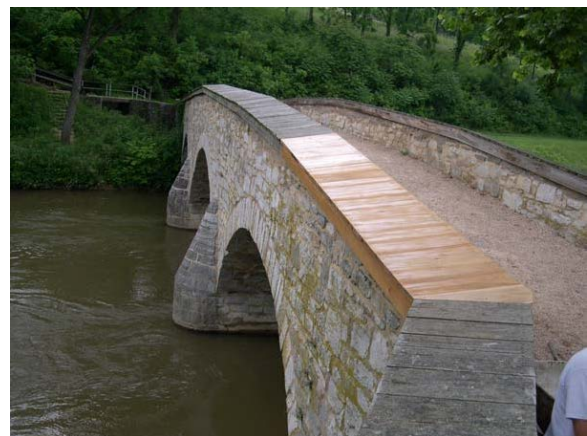
Figure 52. The completed repairs. Photo: NPS DSC eTIC No. ANTI 302 C10.
