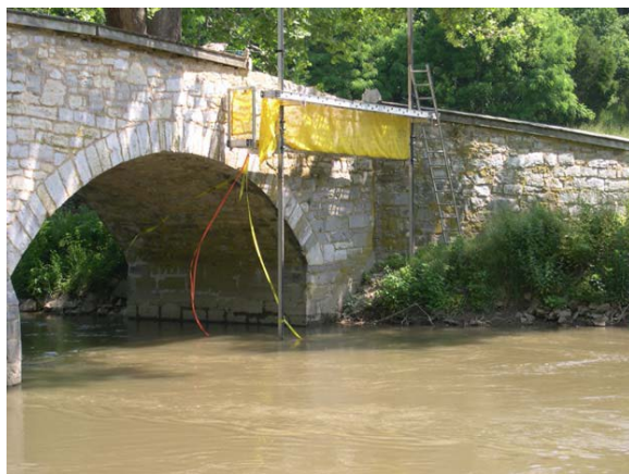
Figure 51. Scaffolding was installed on the south side of the bridge. Photo: NPS DSC eTIC No. ANTI 302 C10.
