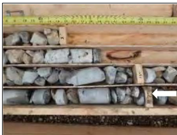
Figure 66. Material extracted from the interior of the piers. Note the material from the pier below the arch bearing indicated by the arrow. Photo: 2014 Pre-Design report.
