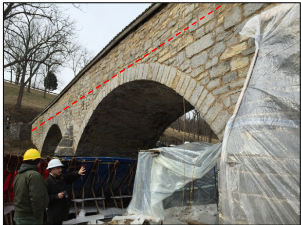
Figure 78. The parapet walls (above dotted line) are a continuation of the spandrel walls with no breaks or water tables. Photo: HPTC, 01/20/16.
