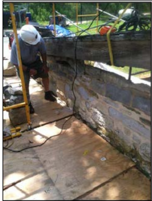
Figure 55. Removing the wood coping. Photo: NPS DSC eTIC No. ANTI 302 127626.
