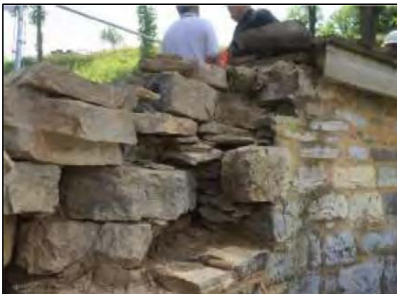
Figure 72. Construction of the parapet. Note the smaller flat stone units on the interior and the lack of mortar between the stones. There is little overlap between the two wythes of stones. Photo: 2014 Pre-Design report.
