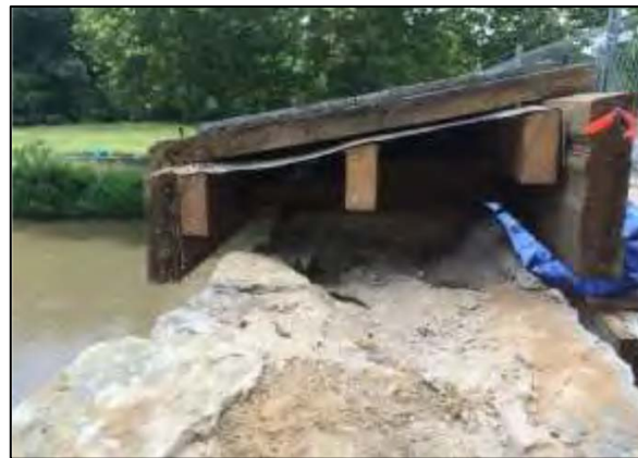
Figure 73. Construction of the wood coping over the parapet. Note the rough surface of the top of the parapet could allow water to sit and infiltrate the wall. Photo: 2014 Pre-Design report.
