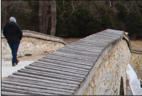
Figure 81. Wood coping boards run along the top of the parapets sloping toward the creek. Photo: HPTC, 01/20/16.
