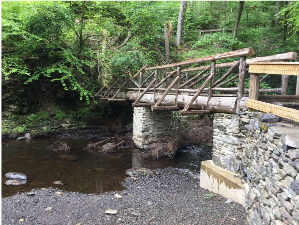
Figure 6. Looking upstream at Dingmans Creek in the Childs Park area. Note the collection of instream wood in the area of the footbridge. NPS – 2018.
