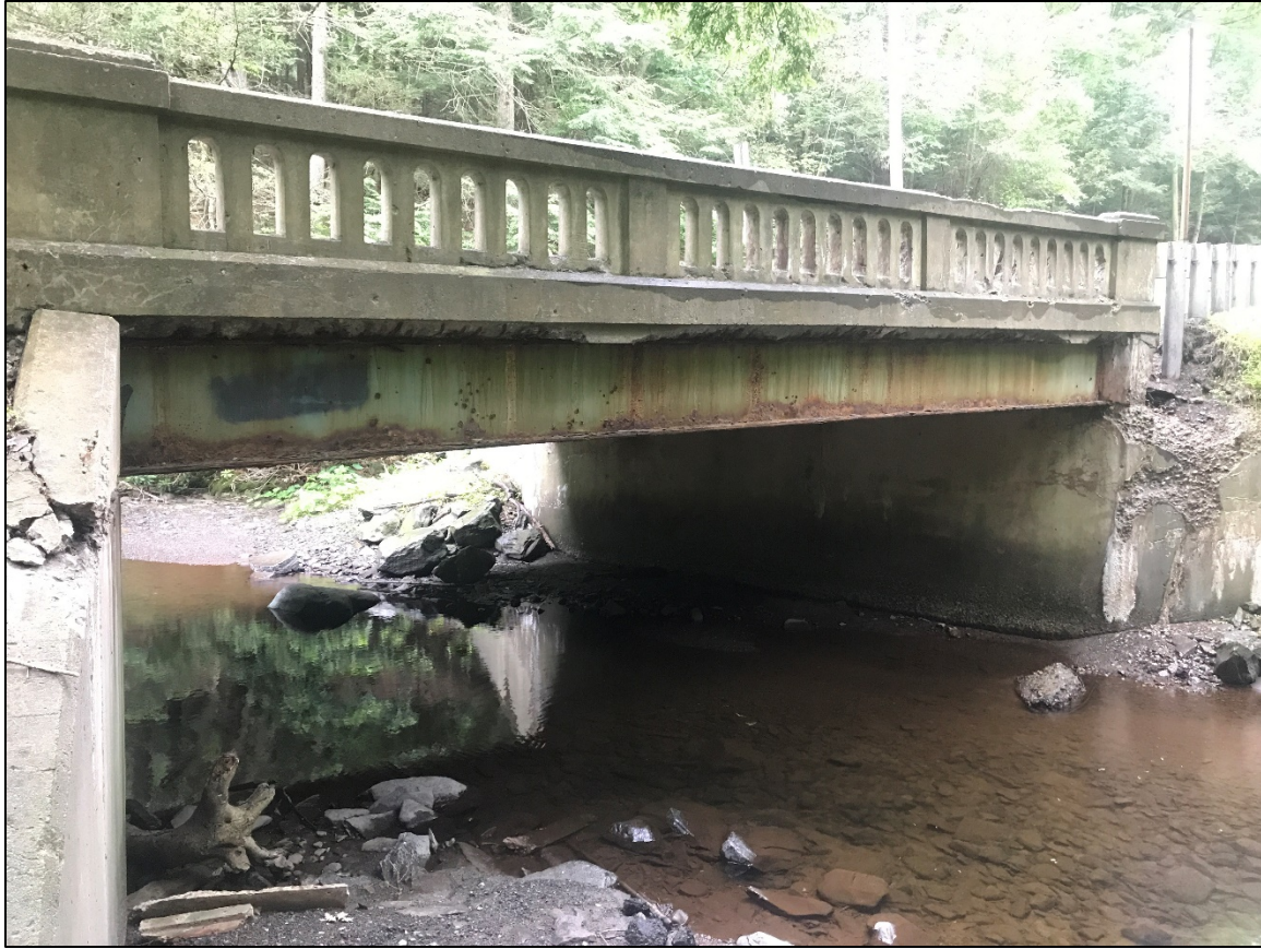
Photograph A2. Dingmans Creek looking downstream 185°S looking at the stream as it flows underneath the SR 2001 Bridge (41.232312, -74.910356). This bridge is indicative of the type of structures that would be vulnerable to instream wood movement within our assessment watersheds. As can be seen here, the bridge is single-span with no piers, which minimizes the chance of instream wood captures. This is the type of structure present at every major bridge crossing we examined as part of this study. Nevertheless, under certain conditions, a logjam could form at this type of bridge crossing leading to redirected flows and possibly damaging resources and infrastructure. A reconnaissance level survey of all bridge crossing after any large flow should be considered.
