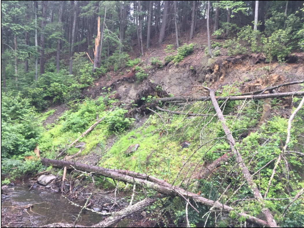
Figure 7. Slope failure immediately upstream of the upper bridge crossing on DFVC road. View is looking upstream. Several large logs that have been mobilized will wind up in the channel, and could block flow under the bridge.
