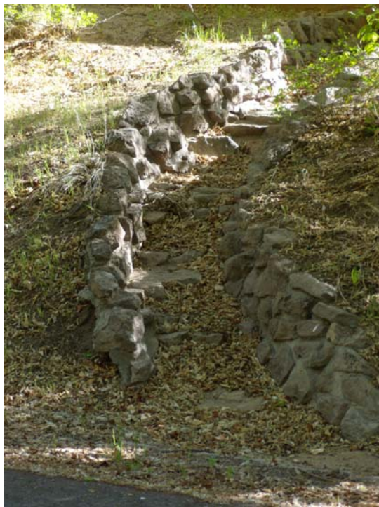
Figure 3. Implementation of Environmental Assessment remedial action #1 'construct an open stone culvert'. This is an example of completed work under the 1996 DDT EA.
