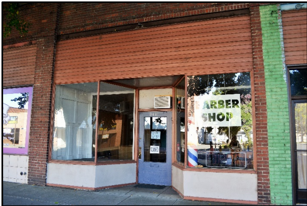
Figure 9. Storefront at 844 Main (Project Number 20); view to the south. Transom lights have been covered.
