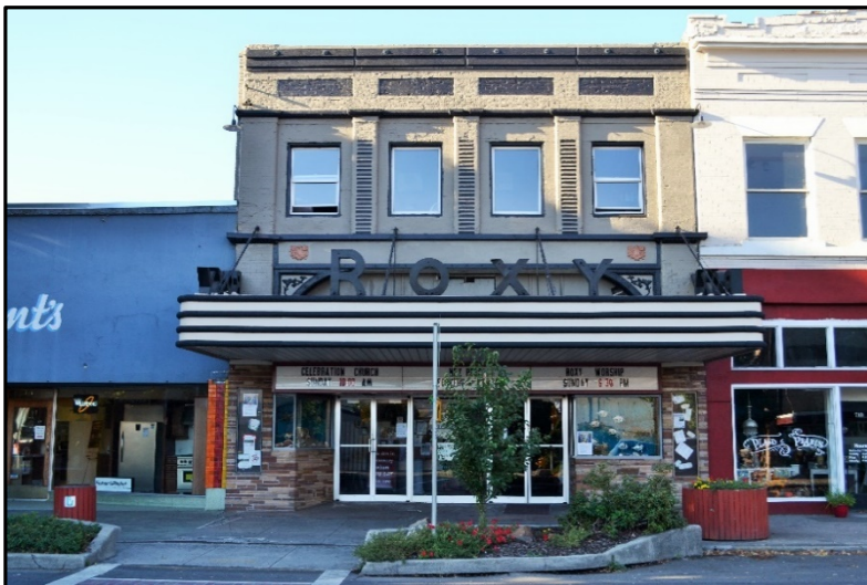
Figure 20. Classical Revival style (upper level): Building at 714 Main Street (Project Number 10), north (front) elevation.
