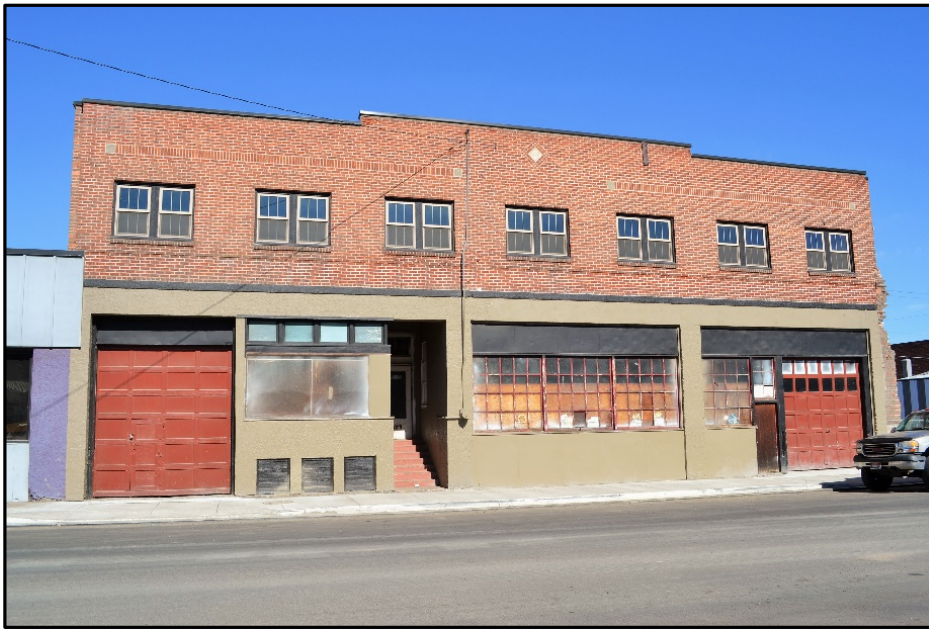
Figure 21. Early 20 th Century Commercial Vernacular style: Building at 835 F Street (Project Number 61), south (front) elevation.
