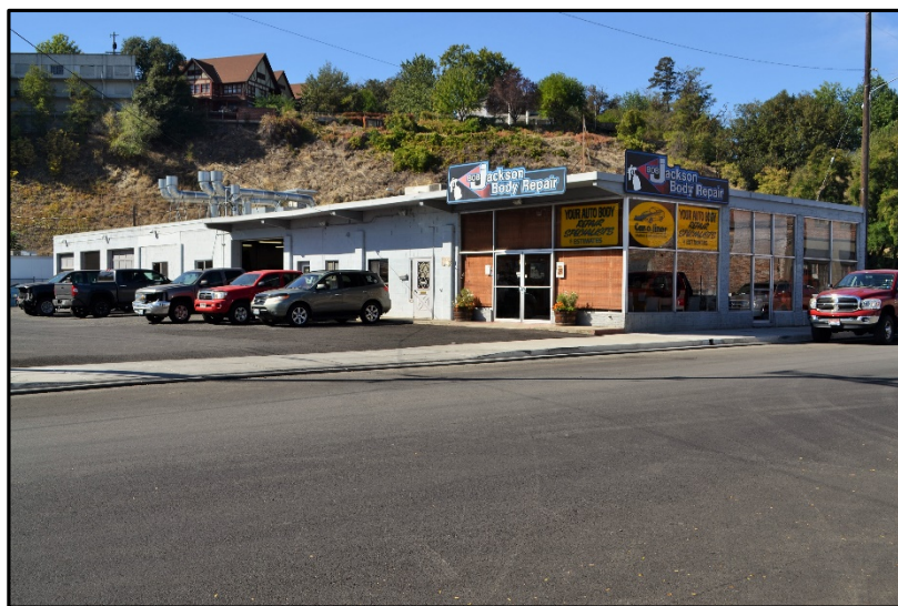
Figure 24. International style: Building at 856 F Street (Project Number 71), east (front) and north sides.
