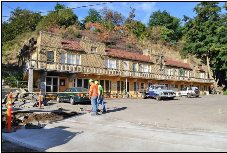
Figure 22. Spanish Eclectic style: Apartment building at 240 New 6 th Street (Project Number 69), east and south (front) sides.
