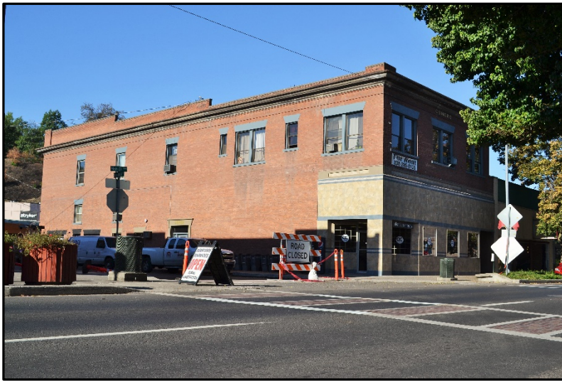
Figure 18. Colonial Revival style: Building at 816 and 818 Main (Project Number 16), east and north (front) sides.
