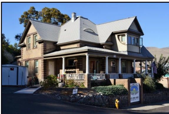
Figure 17. Queen Anne – Free Classic style: House at 224 9 th Street (Project Number 75), south and east (front) sides.
