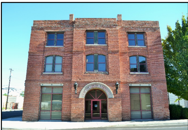
Figure 13. Former bottling plant, former commercial laundry; view to southeast.
