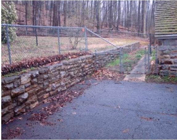
Figures 196, left, and 197, right. A three-foot tall stone retaining wall runs nearly the entire length of the building site in the rear yard (approximately 97'-0") and divides the upper and lower terraces. Photos: HPTC (03/21/12).
