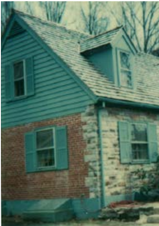
Figure 94. The brick north façade wall was exposed until at least ca. 1991. Photo: CATO Bldg 128 building file.
