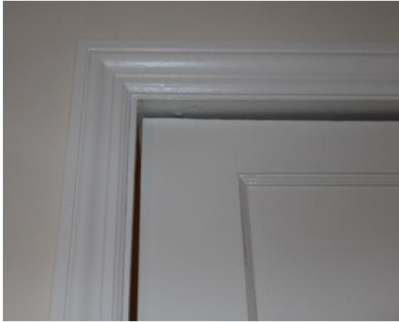
Figure 164. Painted wood door casing on a first-floor door is original. Photo: HPTC (06/12/12).
