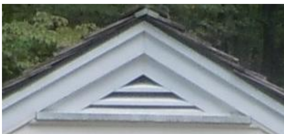
Figure 106. The gable-end louvers have been replaced with metal-clad louvers. Photo: HPTC (08/29/12).
