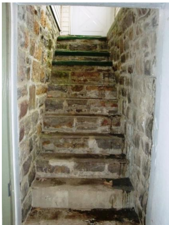
Figure 174. The stone exterior basement staircase; the four upper treads are covered with AstroTurf. Photo: HPTC (04/21/12).
