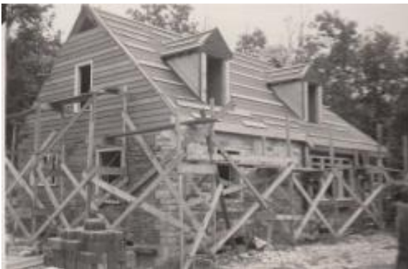
Figure 90. The rough-faced, broken ashlar stone turns the corner to create quoins on the brick north façade. Photo: CATO archives (07/28/48).
