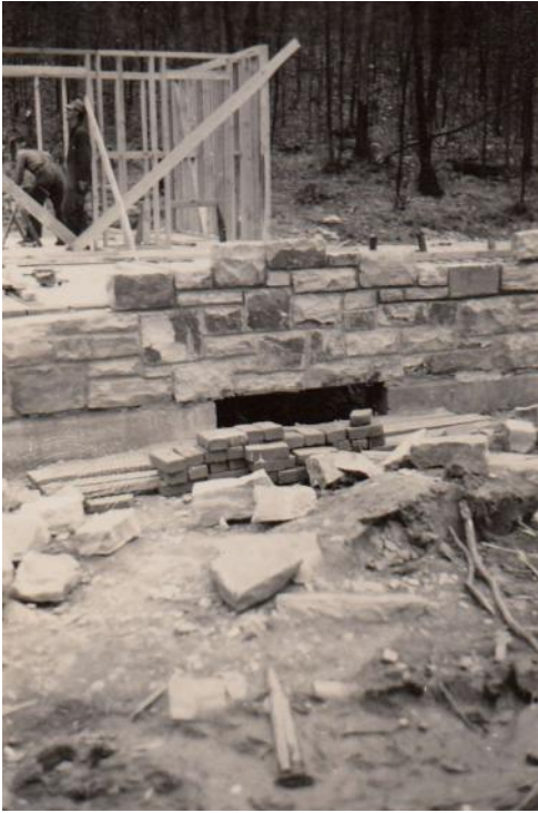
Figure 89. A brick backing can be seen behind the stone facing of the west façade. Note the cement-block backing on the north wall. Photo: CATO archives (04/28/48).
