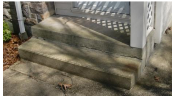
Figure 173. The lowest tread of the exterior stair is now level with the grade. Photo: HPTC (04/21/12).
