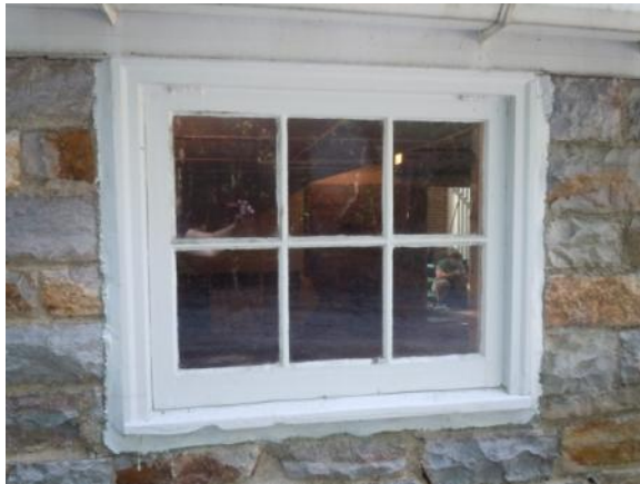
Figure 319, above. The wood six-lite hopper garage windows are original and character-defining features. Photo: HPTC (07/17/12).
