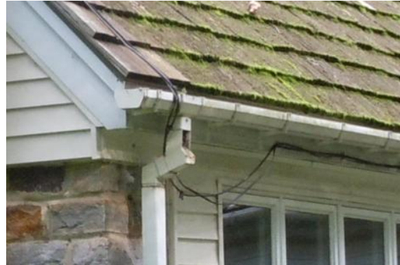
Figure 109. The metal-clad soffit of the sun porch gable roof. Photo: HPTC (08/29/12).
