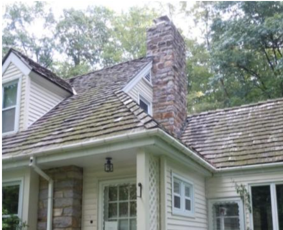
Figure 323. The rear shed dormer projects from the main block gable roof. Photo: HPTC (02/14/12).
