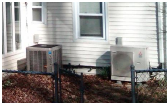
Figure 177. The condenser units for the first-floor forced-air system (left) and the sun porch and second-floor mini-split system (right) is located between the sun porch and eastern ell. Photo: HPTC (04/21/12).
