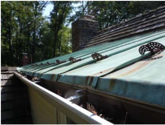
Figure 317. The standing-seam metal covering of the rear dormer shed roof is not original, but is a character-defining feature. Photo: HPTC (07/17/12).
