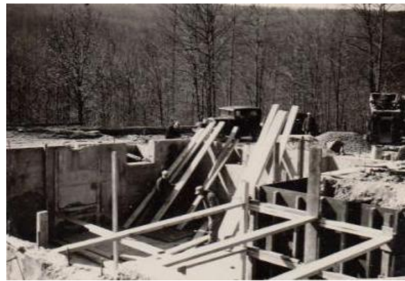
Figure 73. Framework and bracing at the north wall and corner of Room 004. Photo: CATO archives (04/03/48).
