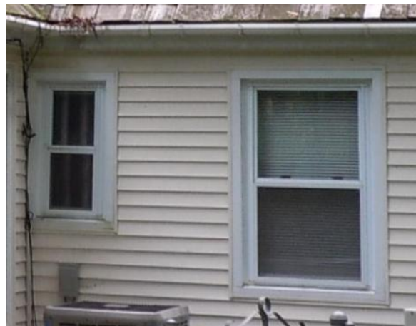
Figure 119. The bathroom and bedrooms windows have been replaced with vinyl-clad, double-hung units. Note the absence of divided lites. Photo: HPTC (08/29/12).
