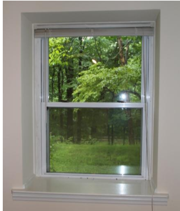
Figure 239. W102 is a vinyl replacement window. Photo; HPTC (06/12/12).
