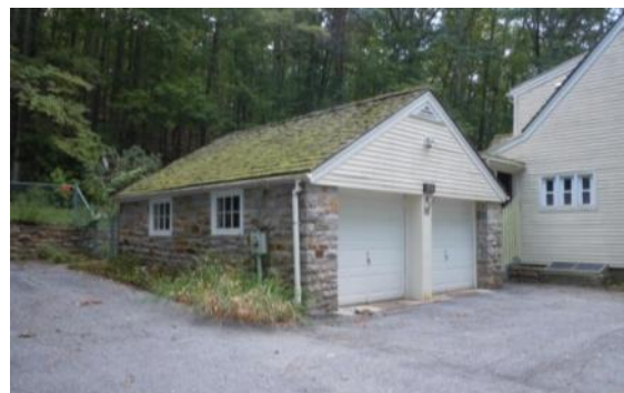
Figure 316. The garage retains its original shape and mass. Photo: HPTC (082912).
