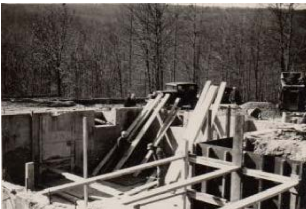
Figure 30. April 3, 1948 photograph showing the reconstruction of portions of the foundation. Photo: Progress Pictures of Custodian's Residence and Garage (Reconstruction). Catoclin Mountain Park archives. See Appendix C for larger copy of photograph.
