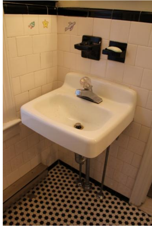
Figure 314. The bathroom sink in Room 209 is likely original. Photo: HPTC (06/12/12).
