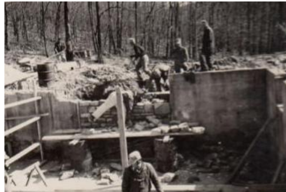
Figure 71. The central stone chimney foundation (south wall in Room 004) was rebuilt after the fire. Photo: CATO archives (04/03/48).
