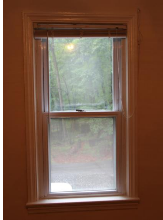
Figure 292. W201 is a vinyl replacement window. Photo: HPTC (06/12/12).
