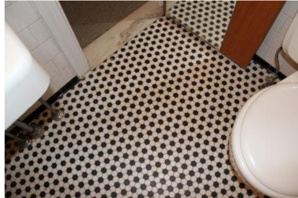
Figure 310. The original ceramic hex-tile on the floor. Photo: HPTC (06/12/12).
