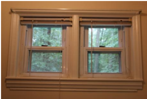
Figure 248. W106 and W107 are vinyl replacement units. Photo: HPTC (06/12/12).
