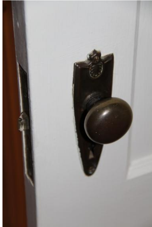
Figure 300. Historic mortise lock set and knob at D204. Photo: HPTC (06/12/12).
