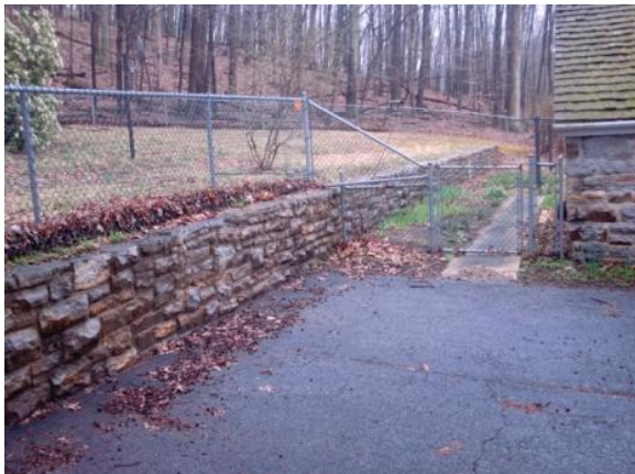
Figure 59. The stone retaining wall dates to 1941 (first complex). Photo: HPTC (04/21/12).
