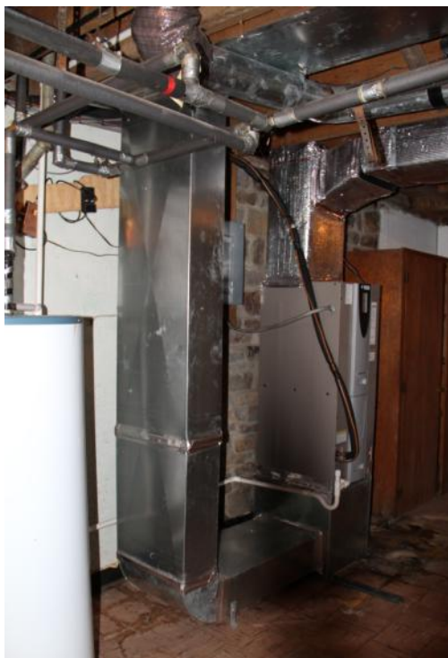
Figure 177. The condenser units for the first-floor forced-air system (left) and the sun porch and second-floor mini-split system (right) is located between the sun porch and eastern ell. Photo: HPTC (04/21/12).
