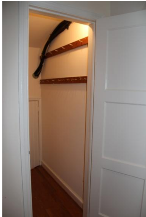
Figure 302. The south wall of Room 204. Photo: HPTC (06/12/12).
