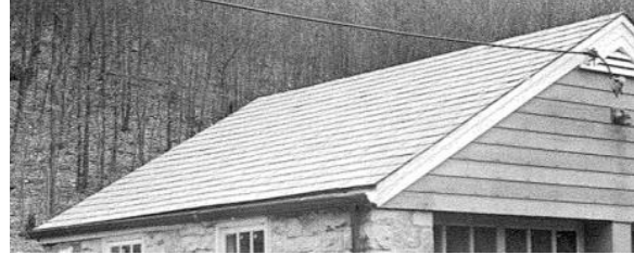
Figure 138. As seen in this ca. 1950 photograph, the garage gable roof was originally clad in slate. Photo: CATO Bldg. 129 building file.
