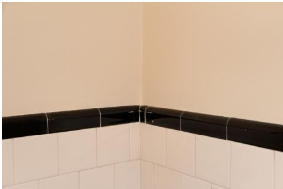
Figure 258. The upper half of the walls in Room 107 are painted plaster; the lower half of the walls are covered with ceramic tile. Photo: HPTC (06/12/12).
