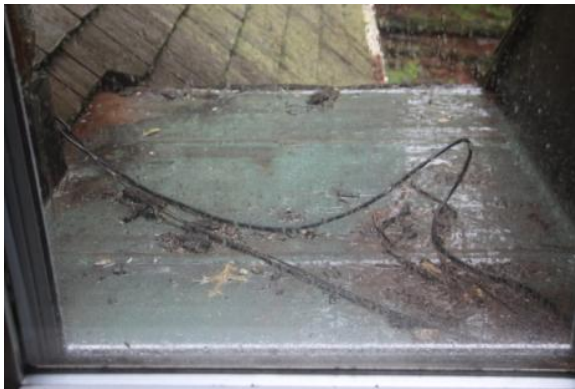
Figure 143. The areaway outside of W204 is flashed with copper. Photo: HPTC (06/12/12).
