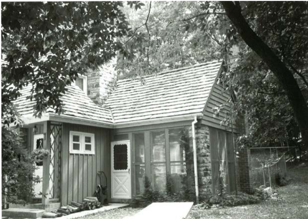
Figure 50. A ca. 1992 photograph shows the chain-link fence installed in 1991 and the sun porch's brick chimney constructed in 1992; it does not show the enclosing windows installed in 1994. Photo: Catoclin Mountain Park building file, Building No. 128 Superintendent's Quarters.
