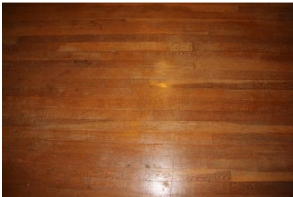
Figure 297. The oak-strip floor in Room 203. Photo: HPTC (06/12/12).
