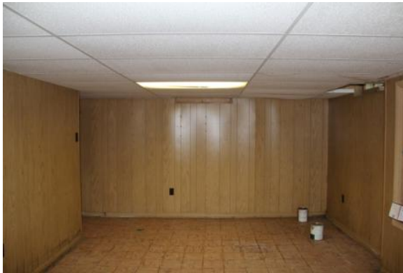
Figure 207. Room 001 looking west. Photo: HPTC (06/20/12).
