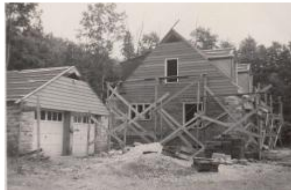
Figure 105. The second-floor gable-end walls of the garage were originally clad in wood lap siding. Photo: CATO archives (07/28/48).
