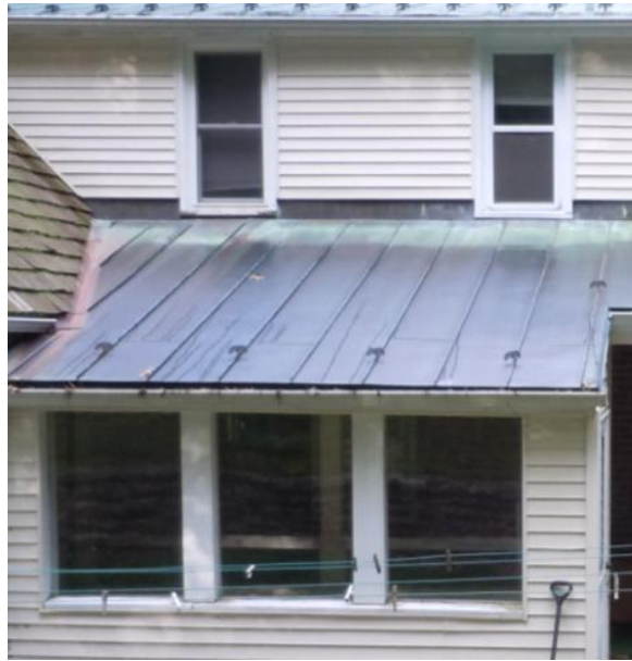
Figure 120. The north elevation kitchen windows have been replaced with vinyl-clad, double-hung units. Photo: HPTC (08/29/12).
