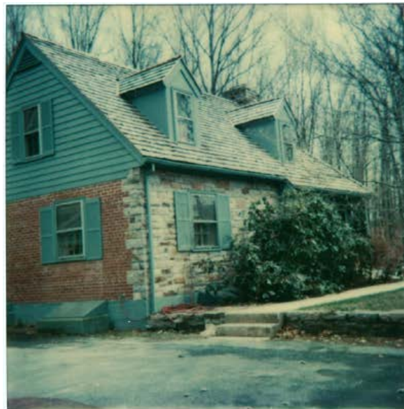
Figure 338. The roofs (except the rear dormer) were originally clad in slate, as seen in this ca. 1950 photograph. The extant wood shakes and metal are not character-defining features. Photo: Catoctin Mountain Park building file, Building No. 128 Superintendent's Quarters.
