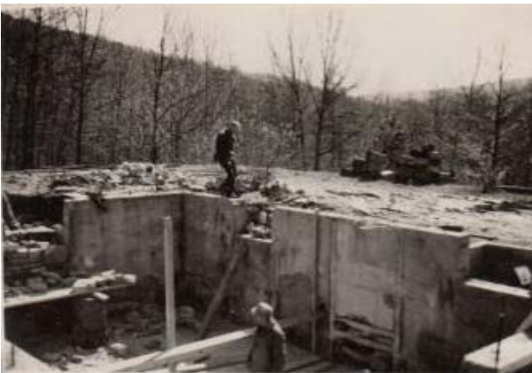
Figure 24. April 3, 1948 photograph of repairs being made to first residence's foundation for reuse on the second residence. Photo: Progress Pictures of Custodian's Residence and Garage (Reconstruction). Catoclin Mountain Park archives. See Appendix C for larger copy of photograph.
