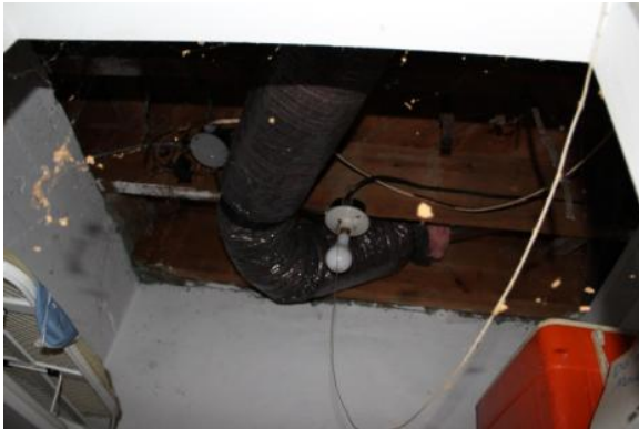
Figure 223. Exposed first-floor structural floor frame at the ceiling. Photo: HPTC (06/20/12).
