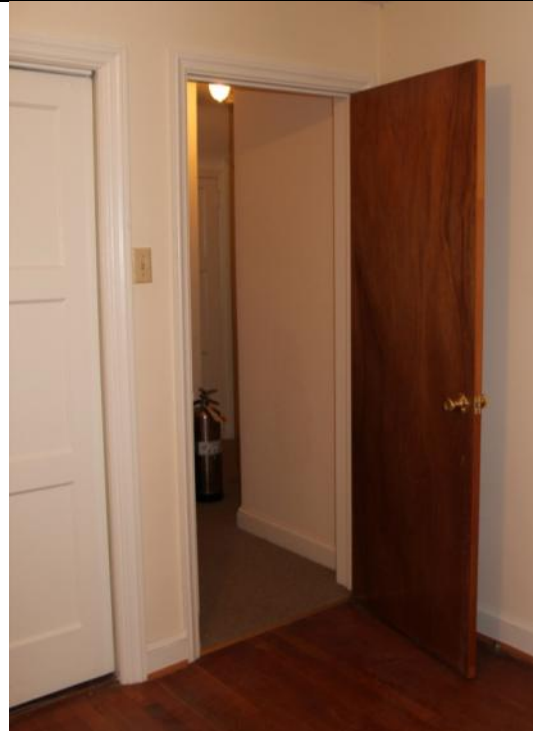
Figure 155. D109 is a replacement hollow-core wood door; conversely the adjacent D108 is an original sliding closet door. Photo: HPTC (06/12/12).
