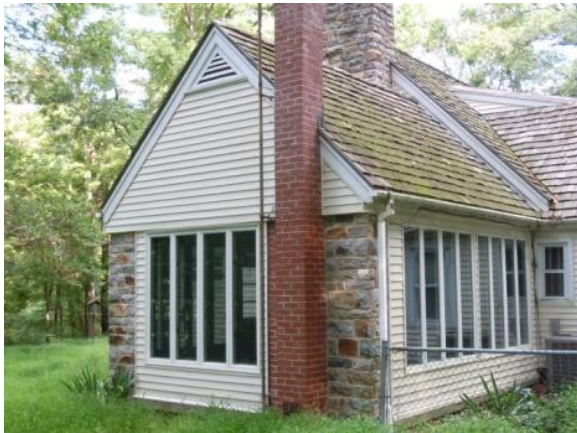
Figure 104. The wood-frame exterior walls of the sun porch, including the lower portion of the infill window walls, are clad with modern vinyl siding. Photo: HPTC (08/29/12).
