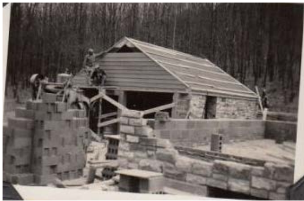
Figure 34. April 24, 1948 photograph showing the reconstruction of the garage. Photo: Progress Pictures of Custodian's Residence and Garage (Reconstruction). Catoclin Mountain Park archives. See Appendix C for larger copy of photographs.
