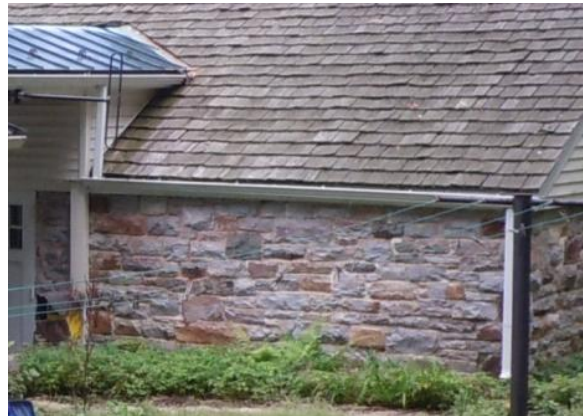
Figure 148. The aluminum drainage system on the south elevation (eastern portion) of the garage. Photo: HPTC (08/29/12).
