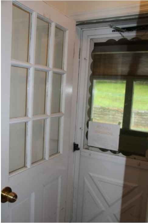
Figure 126. D110E was replaced in 1995. Photo: HPTC (06/12/12).
