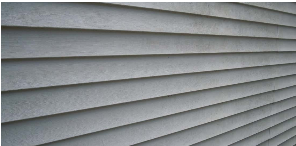
Figure 355. Modern vinyl siding covers the north elevation brick wall of the main block. Photo: HPTC (08/29/12).
