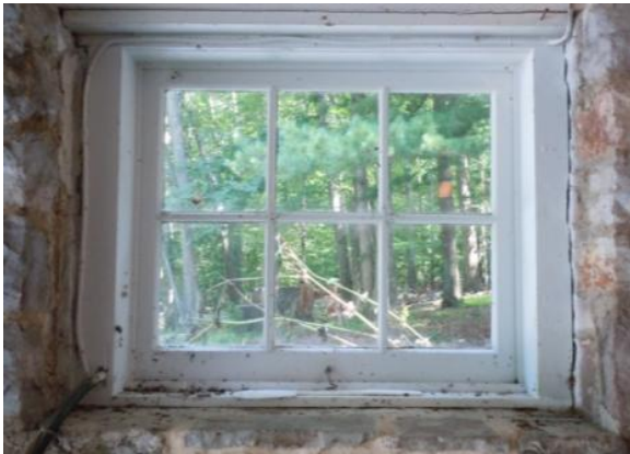
Figure 284. WG101 is an original wood hopper window. Photo: HPTC (07/17/12).
