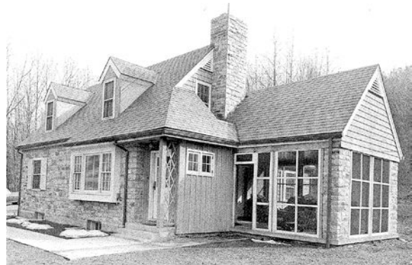
Figure 99. In this ca. 1950 photograph, the front dormer walls were clad in beaded wood siding. The main block gable end walls were clad in wood lap siding. Photo: CATO Bldg. 128 building file.
