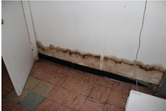
Figure 229. The frame partition walls are covered with painted particle board. Photo: HPTC (06/20/12).
