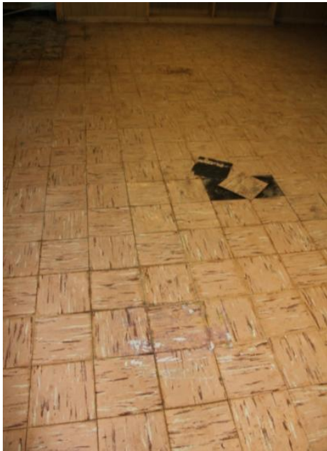
Figure 209. The concrete floor slab is covered with rigid tile. Photo: HPTC (06/20/12).
