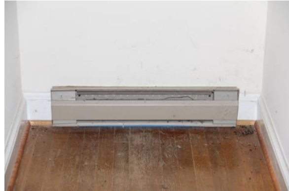
Figure 181. An electric baseboard heater in a second-floor room. Photo: HPTC (06/12/12).
