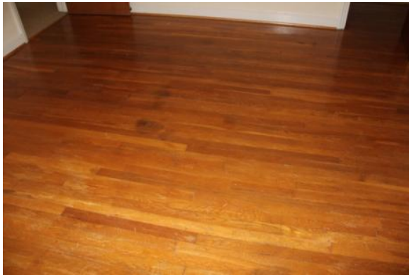
Figure 289. Oak-strip flooring in Room 201. Photo: HPTC (06/12/12).
