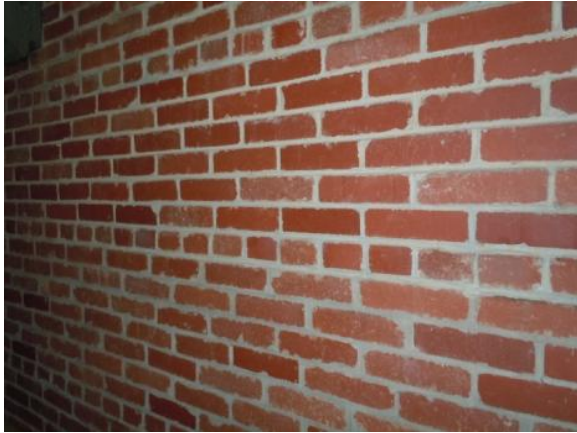
Figure 96. The brick is still exposed on the east façade (6:1 common bond with partial-Portland cement mortar. Photo: HPTC (08/29/12).
