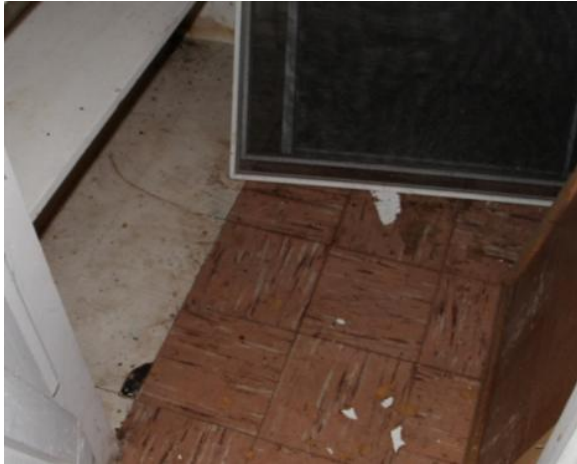
Figure 80. The basement concrete floor slab is entirely covered with tile in Room 003. Photo: HPTC (06/20/12).
