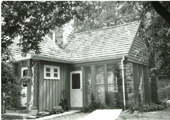
Figure 100. The vestibule was originally clad in board and batten siding, as seen in this ca. 1992 photograph. Photo: CATO Bldg. 128 building file.
