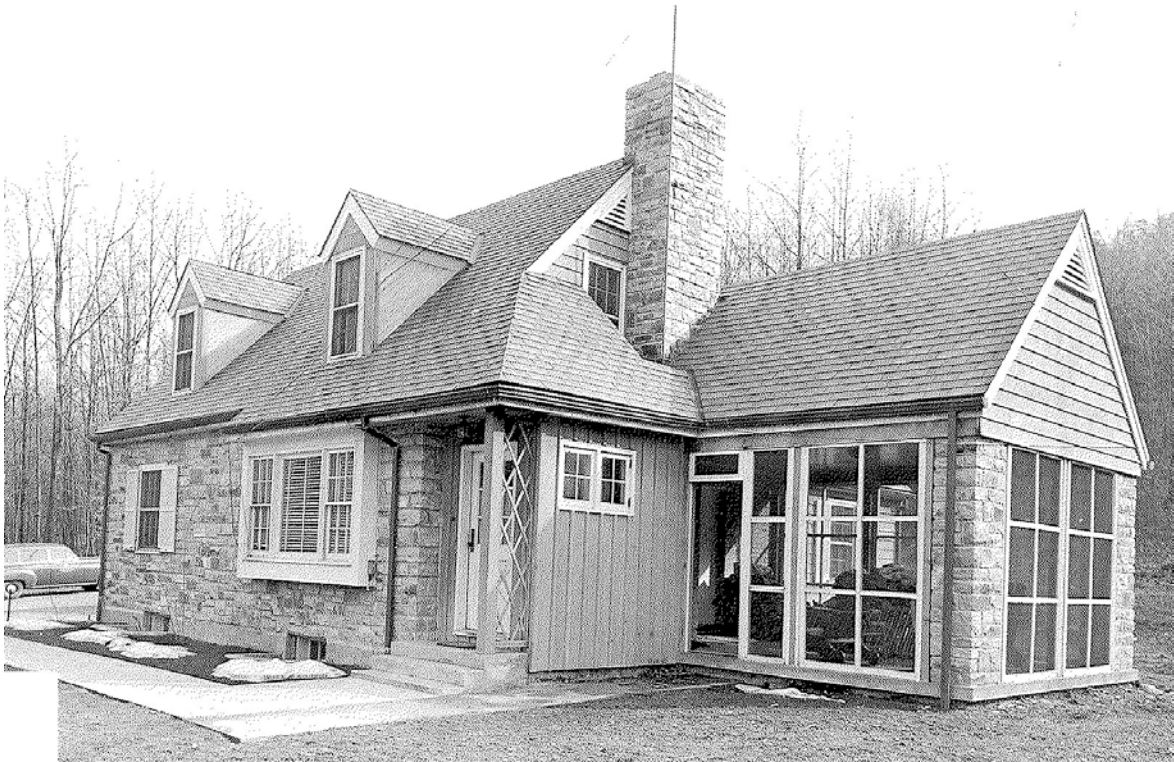
Figure 42. A ca. 1950 photograph of the Quarters 1 residence from the southwest corner. The pole on the chimney is a television antenna, not a lightning protection system. Photo: Catoclin Mountain Park building file, Building No. 128 Superintendent's Quarters. See Appendix C for larger copies of photographs.
