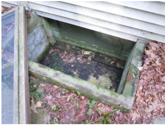
Figure 78. The below-grade basement window openings include concrete-parged brick window wells. Photo: HPTC (08/29/12).
