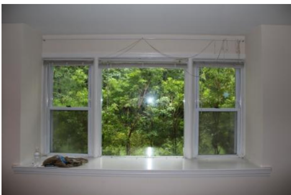
Figure 244. W103-W105 are located in the front elevation bay window. Photo: HPTC (06/12/12).
