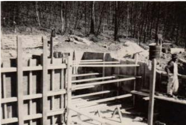
Figure 28. April 3, 1948 photograph showing the reconstruction of portions of the foundation. Photo: Progress Pictures of Custodian's Residence and Garage (Reconstruction). Catoclin Mountain Park archives. See Appendix C for larger copy of photograph.
