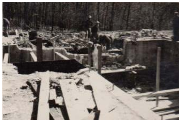
Figure 25. April 3, 1948 photograph of the reconstruction of the stone chimney foundation. Photo: Progress Pictures of Custodian's Residence and Garage (Reconstruction). Catoclin Mountain Park archives. See Appendix C for larger copy of photograph.
