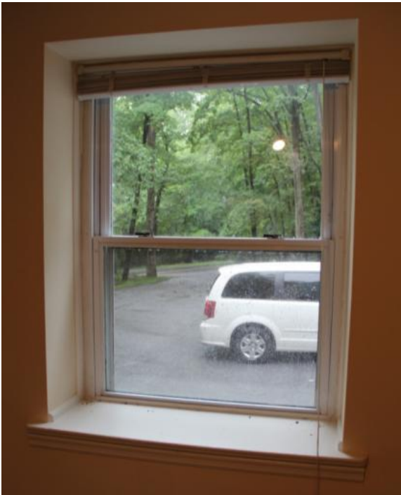
Figure 238. W101 is a vinyl replacement window. Photo: HPTC (06/12/12).
