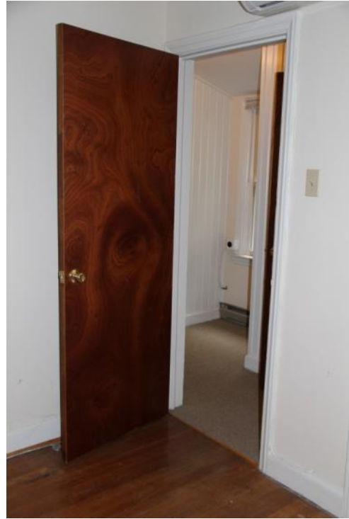
Figure 159. D203 is a replacement hollow-core door on the second floor. Photo: HPTC (06/12/12).
