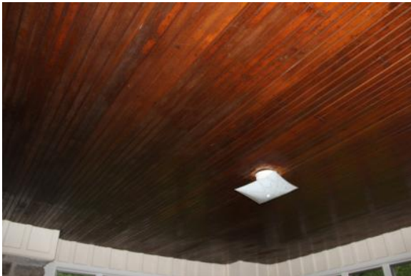
Figure 252. The stained wood beadboard ceiling in Room 106. Photo: HPTC (06/12/12).
