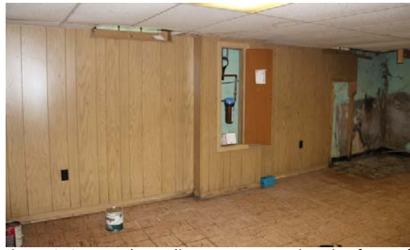
Figure 349. Wood paneling covers many interior faces of the foundation walls hiding the condition of the concrete behind. Photo: HPTC (06/12/12).
