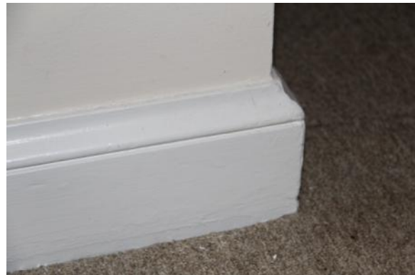
Figure 331. Original wood baseboard can be seen throughout most of the first and second floors. Photo: HPTC (06/12/12).
