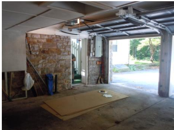
Figure 281. Room G101 looking towards the southwest corner. Photo: HPTC (07/17/12).
