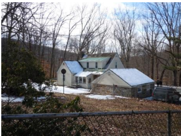
Figure 200. The rear lawn is separated from Quarters 1 by a stone retaining wall. Photo: HPTC (02/14/12).
