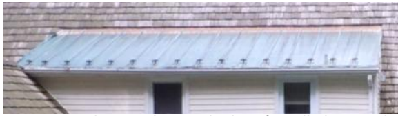
Figure 135. The rear dormer shed roof is clad in standing-seam copper. Photo: HPTC (08/29/12).
