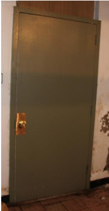
Figure 124. D004E is a replacement solid-core wood door. Photo: HPTC (06/20/12).
