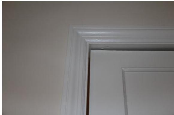
Figure 333. Original interior wood door trim can be seen throughout Quarters 1. Photo: HPTC (06/12/12).
