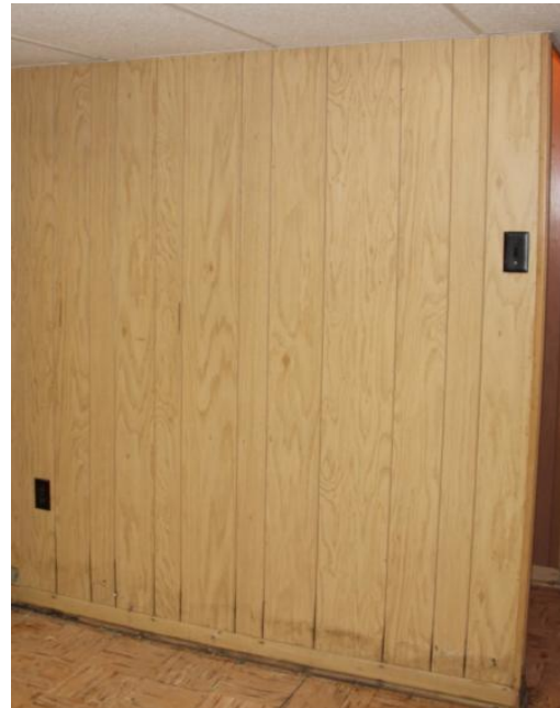
Figure 210. The walls are covered with faux-wood paneling. Photo: HPTC (06/20/12).
