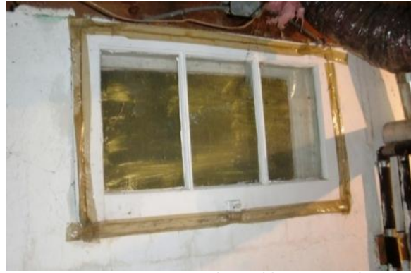
Figure 230. W005 is an original wood hopper window with original hinges and locking hardware. Photo: HPTC (03/21/12).
