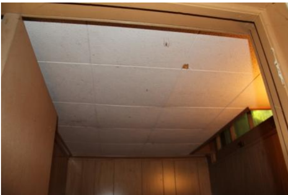
Figure 217. The ceiling is covered with acoustical tiles (not suspended). Photo: HPTC (06/20/12).
