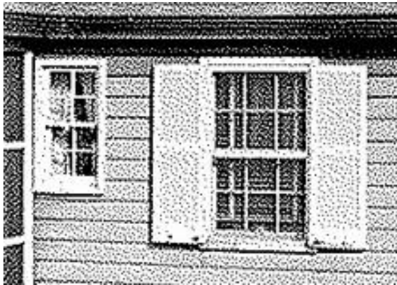
Figure 342. The original windows were composed of wood and had divided lites. The extant vinyl replacement units are not character-defining features. Photo: Catoclin Mountain Park building file, Building No. 128 Superintendent's Quarters.
