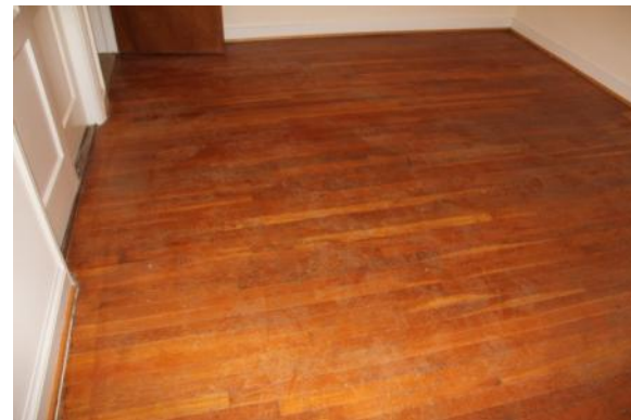
Figure 335. Wood-strip flooring is original and character defining. Photo: HPTC (06/12/12).
