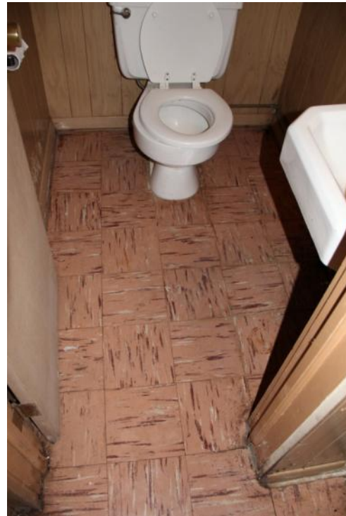
Figure 216. The concrete floor slab is covered with rigid tiles. Photo: HPTC (06/20/12).
