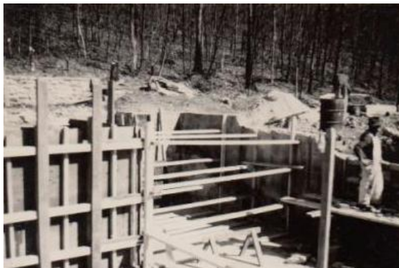
Figure 72. The north wall and corner of Room 004 were re-cast; note the framework and bracing. Photo: CATO archives (04/03/48).
