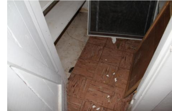
Figure 222. The concrete floor slab is covered with rigid tile. Photo: HPTC (06/20/12).
