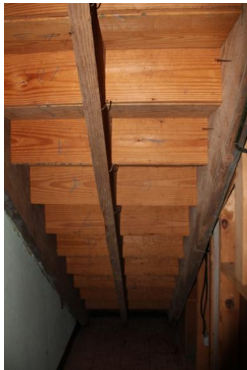
Figure 169. The basement stairs are composed of wood frame. Photo: HPTC (06/20/12).
