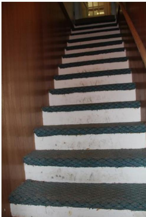
Figure 168. The basement stairs have painted risers, carpeted treads, and an unpainted banister. Photo: HPTC (06/20/12).
