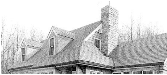
Figure 338. The roofs (except the rear dormer) were originally clad in slate, as seen in this ca. 1950 photograph. The extant wood shakes and metal are not character-defining features. Photo: Catoctin Mountain Park building file, Building No. 128 Superintendent's Quarters.
