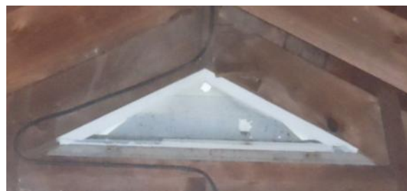
Figure 107. The interior of the north garage louver has a screen. Photo: HPTC (07/17/12).
