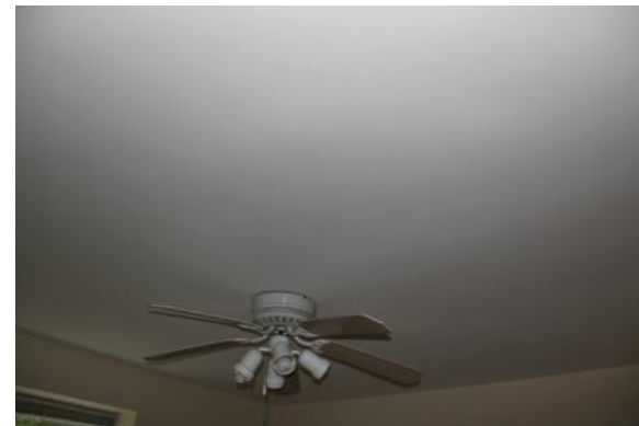
Figure 237. The ceiling is composed of painted plaster. Note the modern ceiling fan-light fixture. Photo: HPTC (06/12/12).
