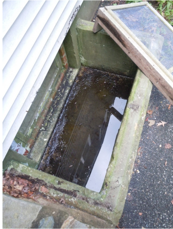
Figure 390. Neutral and negative drainage can be seen across the rear elevation. Photo: HPTC (08/29/12).
