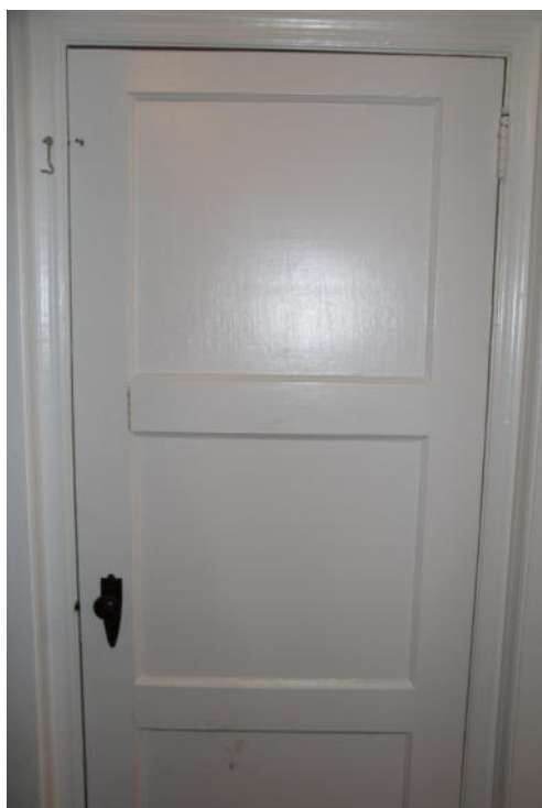
Figure 272. D110B is an original wood door which leads to the basement stair. Note the original mortise knob set and the original hinges. Photo: HPTC (06/12/12).
