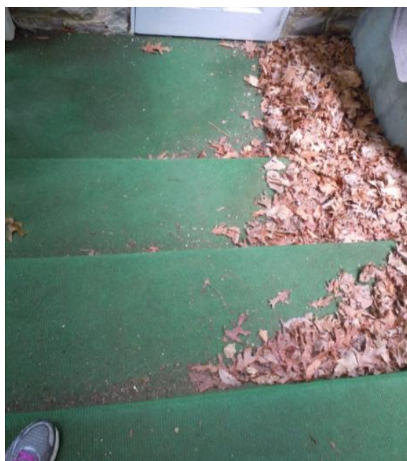
Figure 175. The breezeway stair is composed of concrete covered with AstroTurf. Photo: HPTC (08/20/12).
