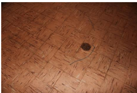
Figure 227. The concrete floor slab is covered with rigid tiles. Photo: HPTC (06/20/12).
