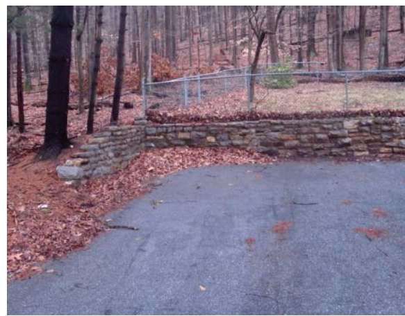
Figures 196, left, and 197, right. A three-foot tall stone retaining wall runs nearly the entire length of the building site in the rear yard (approximately 97'-0") and divides the upper and lower terraces. Photos: HPTC (03/21/12).
