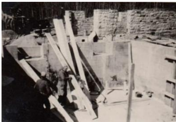
Figure 74. The north wall of Room 001 was reused from the 1941 building. Note the garage shell with 1941 stone walls. Photo: CATO archives (04/03/48).
