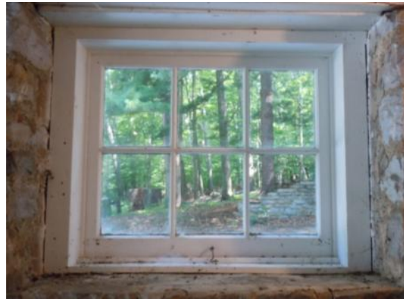
Figure 285. WG102 is an original wood hopper window. Photo: HPTC (07/17/12).
