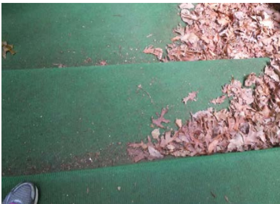
Figure 352. Astroturf-style carpet covers the breezeway concrete slab. Photo: HPTC (08/29/12).
