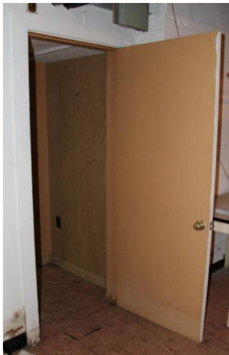
Figure 153. A replacement hollow-core basement door (D004). Photo: HPTC (07/17/12).
