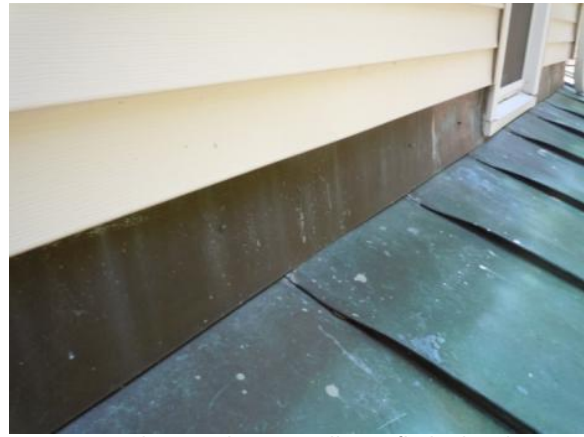
Figure 142. The rear dormer walls are flashed with copper. Photo: HPTC (07/17/12).
