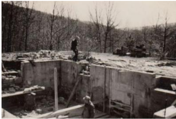
Figure 70. The west foundation wall of Rooms 001, 002, and 003 were reused from the 1941 building. Photo: CATO archives (04/03/48).
