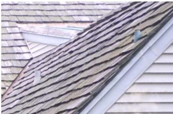
Figure 149. Two copper pipe vents penetrate the southern slope of the main block's eastern ell. Photo: HPTC (08/29/12).
