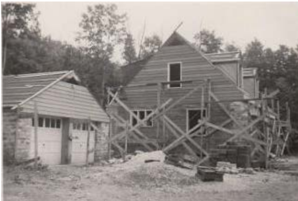
Figure 38. July 24, 1948 photograph of the north elevation. Photo: Progress Pictures of Custodian's Residence and Garage (Reconstruction). Catoclin Mountain Park archives. See Appendix C for larger copy of photograph.
