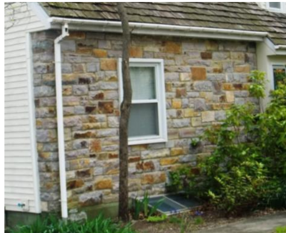
Figure 91. The stone masonry west façade as seen in 2012. Photo: HPTC (04/21/12).
