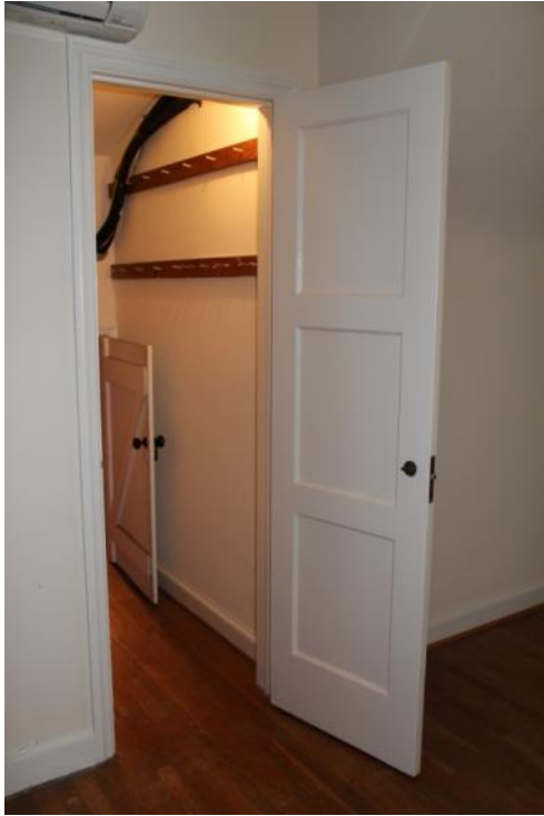
Figure 158. D204 is an original 3-panel door on the second floor. Photo: HPTC (06/12/12).
