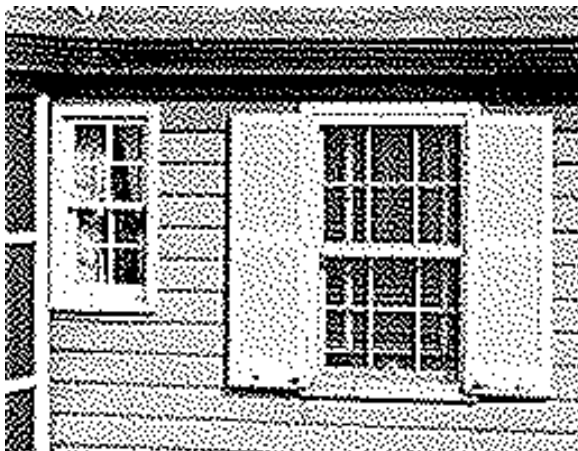
Figure 118. This ca. 1950 photograph shows the bathroom window (left) was originally a 4/4 double-hung wood unit; the bedroom windows were 6/6 double-hung wood units. Photo: CATO Bldg. 128 building file.
