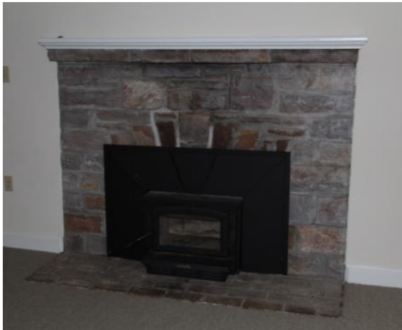
Figure 166. The living room fireplace is original; the metal insert is modern. Photo: HPTC (06/12/12).
