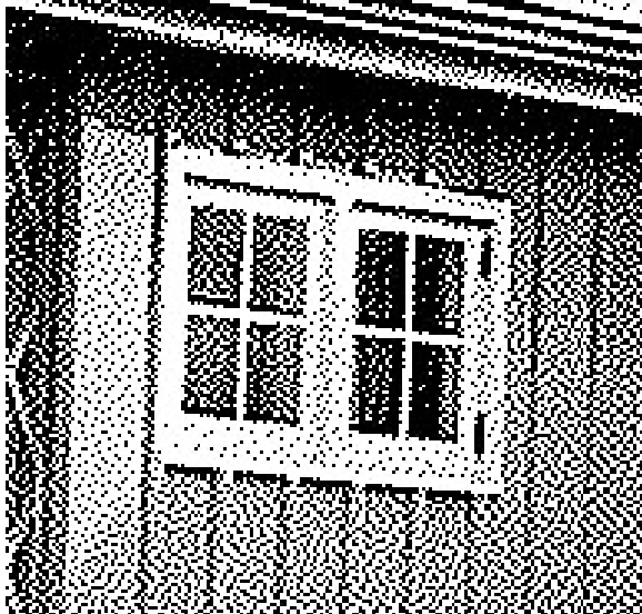
Figure 116. This ca. 1950 photograph shows the vestibule windows were originally four-lite wood casement units. Photo: CATO Bldg. 128 building file.
