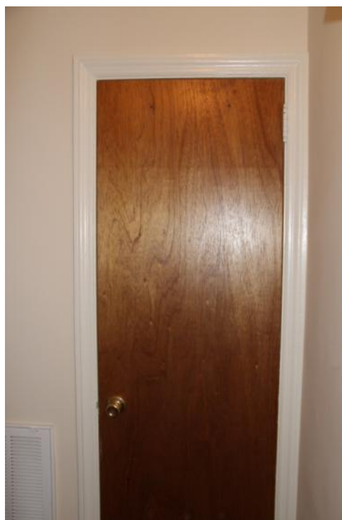
Figure 273. D111 is a replacement hollow-core closet door. It has a modern knob set and historic hinges. Photo: HPTC (06/12/12).
