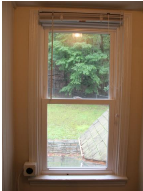
Figure 306. W205 is a modern replacement unit. Photo: HPTC (06/12/12).
