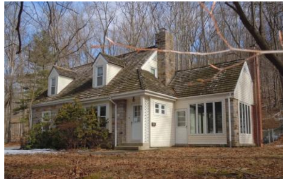
Figure 56. Quarters 1 from the southwest. Photo: HPTC (02/14/12).
