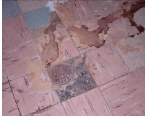
Figure 81. One of the two floor drains in Room 004. Photo: HPTC (04/21/12).
