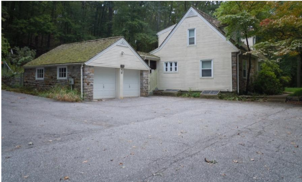
Figure 189. The parking areas to the west and south of the garage are paved. Photo: HPTC (08/29/12).
