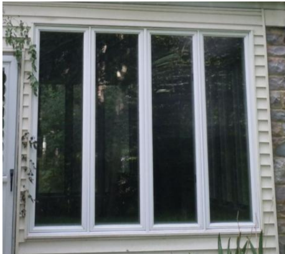
Figure 122. The sun porch was infilled with windows in 1994; these windows have since been replaced. Photo: HPTC (08/29/12).
