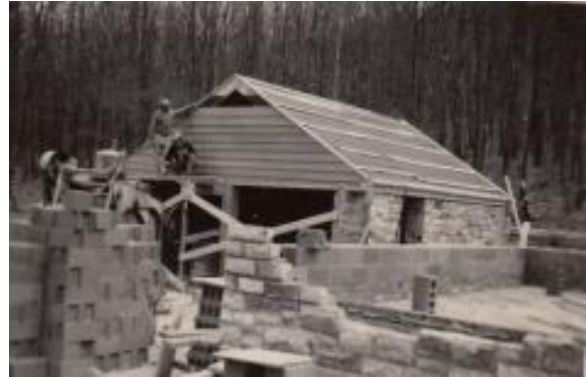
Figure 89. A brick backing can be seen behind the stone facing of the west façade. Note the cement-block backing on the north wall. Photo: CATO archives (04/28/48).
