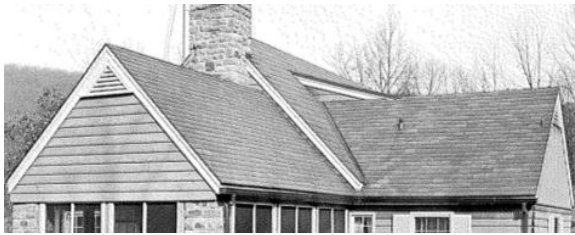
Figure 137. As seen in this ca. 1950 photograph, the eastern ell and sun porch gable roofs were originally clad in slate. Photo: CATO Bldg. 128 building file.
