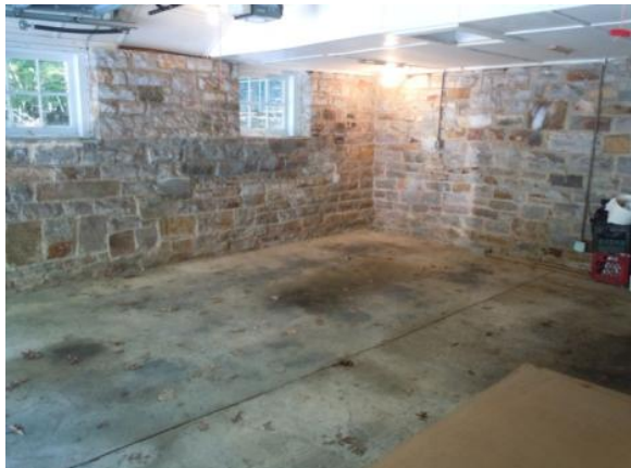
Figure 280. Room G101 looking towards the northeast corner. Photo: HPTC (07/17/12).
