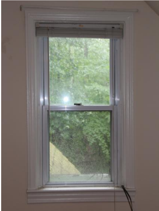
Figure 299. W204 is a vinyl replacement window. Photo: HPTC (06/12/12).
