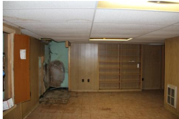
Figure 208. Room 001 looking east. Photo: HPTC (06/20/12).
