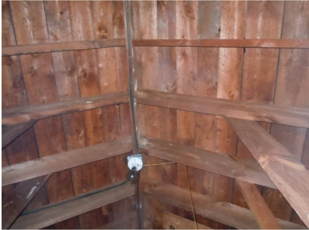
Figure 87. The garage roof structural frame can be seen through a scuttle from the first floor. Photo: HPTC (07/17/12).
