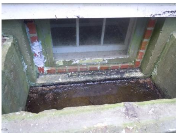
Figure 110. All of the basement windows are original. Photo: HPTC (08/29/12).
