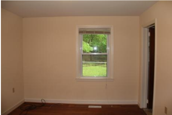
Figure 264. Room 109 looking south. Photo: HPTC (06/12/12).
