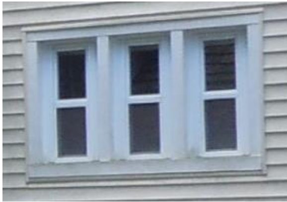
Figure 120. The north elevation kitchen windows have been replaced with vinyl-clad, double-hung units. Photo: HPTC (08/29/12).
