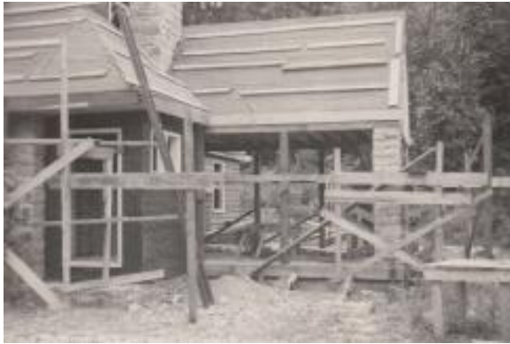
Figure 102. Stone piers support the roof and gable-end wall frames of the sun porch. Photo: CATO archives (07/28/48).
