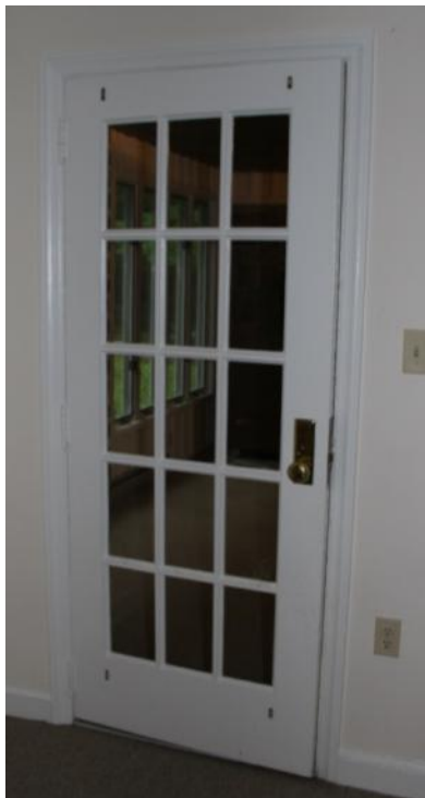
Figure 156. D106 became an interior door after the sun porch was enclosed in 1994. Photo: HPTC (06/12/12).
