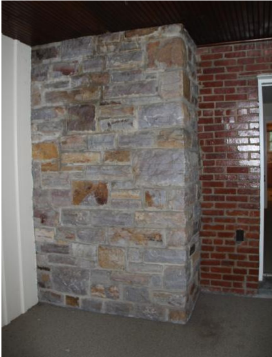
Figure 92. The main block broken-ashlar stone chimney walls can be seen in the sun porch. Note the exposed brick wall. Photo: HPTC (06/12/12).
