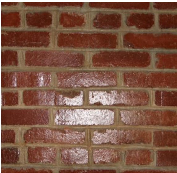
Figure 324. The gable end walls and the rear (east) façade of the main block are constructed of brick in a 6:1 common bond pattern. Photo: HPTC (06/12/12).
