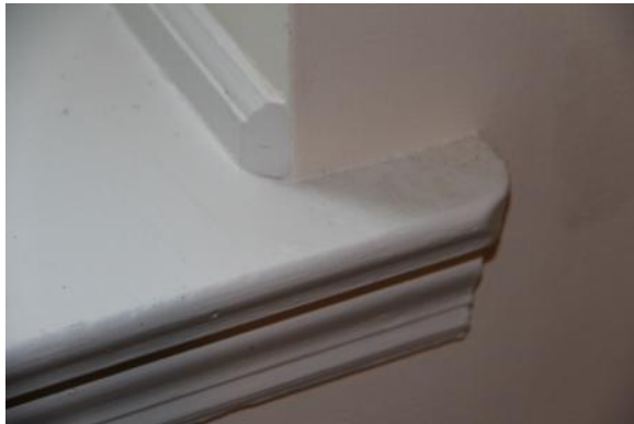
Figure 332. Original interior wood window trim can be seen throughout Quarters 1. Photo: HPTC (06/12/12).
