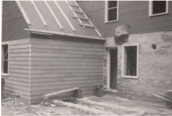
Figure 98. The eastern ell was originally clad in wood lap siding. Photo: CATO archives (07/28/48).
