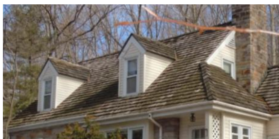
Figure 134. The main block gable and hipped roof and the front dormer gable roofs are now clad in cedar shakes. Photo: HPTC (02/14/12).
