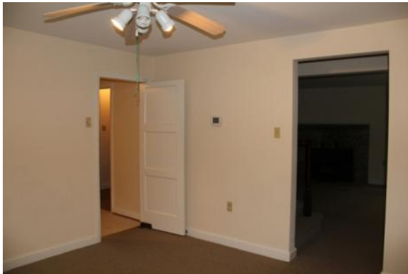
Figure 234. Room 101 looking southeast. Note the inconspicuous swinging door hinges on D101. Photo: HPTC (06/12/12).
