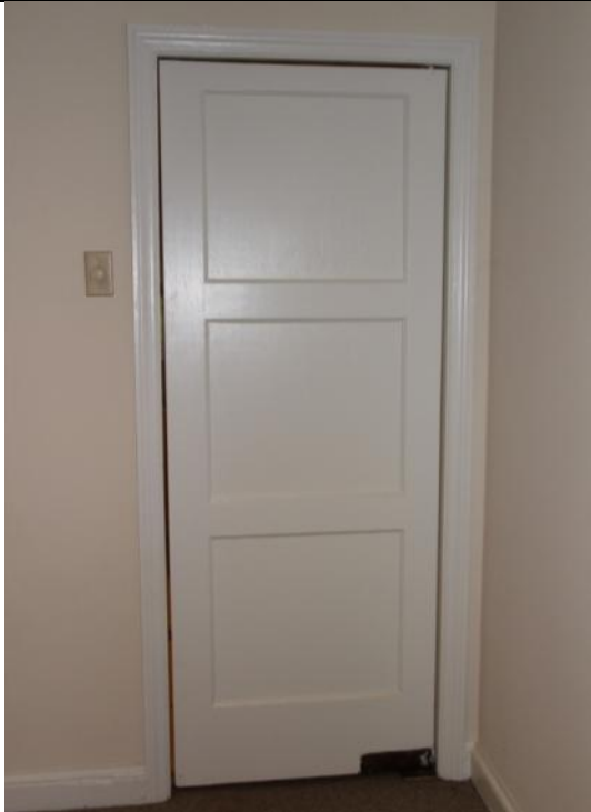
Figure 154. D101 is an original 3-panel painted wood swinging door between the dining room and kitchen. Photo: HPTC (06/12/12).
