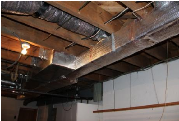
Figure 84. The exposed first-floor structural floor frame as seen from Room 004. Photo: HPTC (06/20/12).
