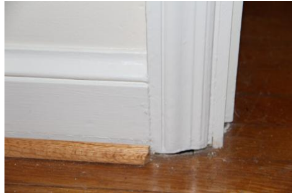
Figure 165. Painted wood baseboard with unpainted quarterround and painted wood door casing on the second floor. Photo: HPTC (06/12/12).
