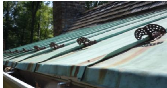
Figure 329. The rear dormer shed roof with handcrafted standing-seam metal roof. Photo: HPTC (07/17/12).
