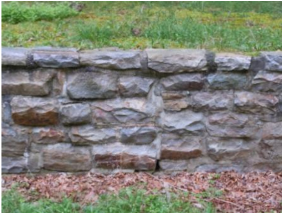
Figure 326. Original Stone retaining walls can be seen on the east and west elevations of Quarters 1. Photo: HPTC (06/12/12).
