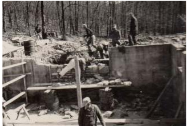
Figure 27. April 3, 1948 photograph showing the reconstruction of the stone chimney foundation. Photo: Progress Pictures of Custodian's Residence and Garage (Reconstruction). Catoclin Mountain Park archives. See Appendix C for larger copy of photograph.
