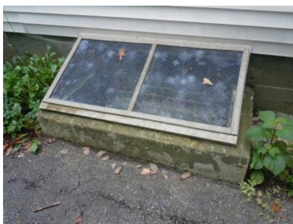
Figure 111. The basement window openings include screened frames above the window well. Photo: HPTC (08/29/12).
