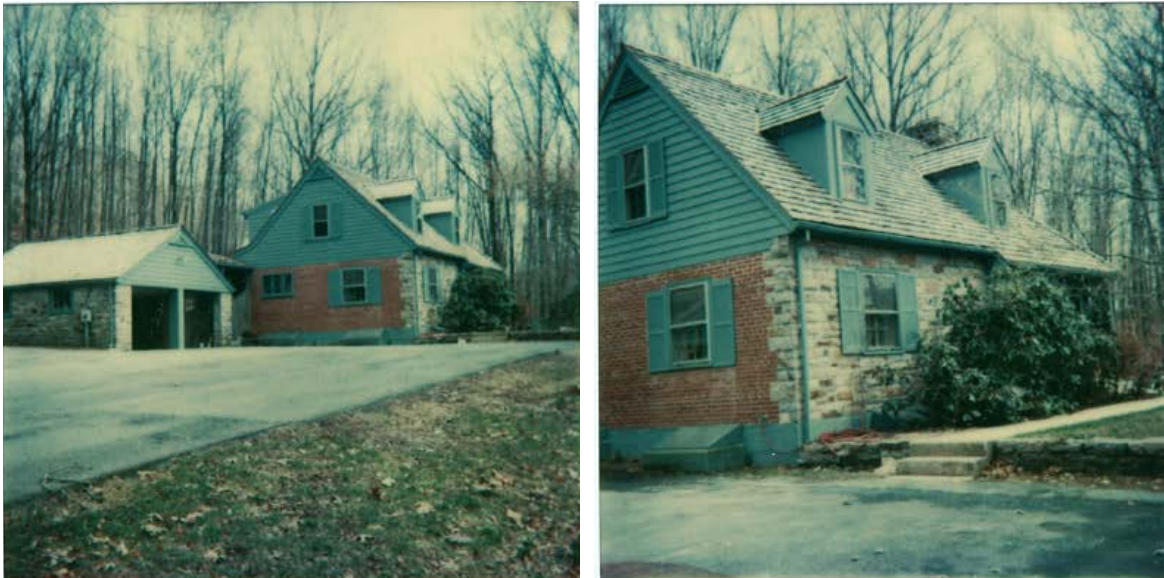
Figure 48, left, and Figure 49, right. These undated photographs may depict Quarters 1 after the exterior was painted in 1991. Photo: Catoclin Mountain Park building file, Building No. 128 Superintendent's Quarters.
