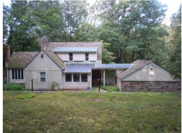
Figure 101. All of the wood-frame exterior walls have been clad with modern vinyl siding. Photo: HPTC (08/29/12).
