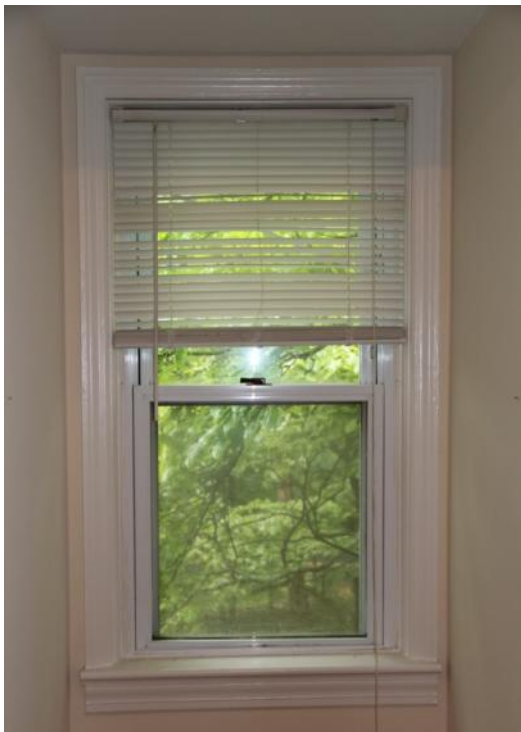
Figure 293. W202 is a vinyl replacement window. Photo: HPTC (06/12/12).
