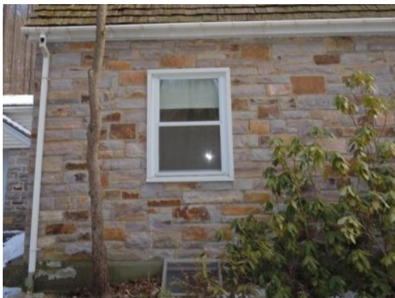
Figure 145. The vinyl drainage system on the west elevation of the main block. Photo: HPTC (04/21/12).
