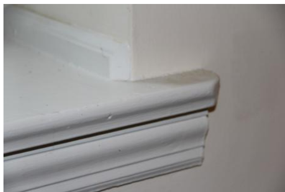
Figure 163. Painted wood window sill and stool at a first-floor window. Photo: HPTC (06/12/12).
