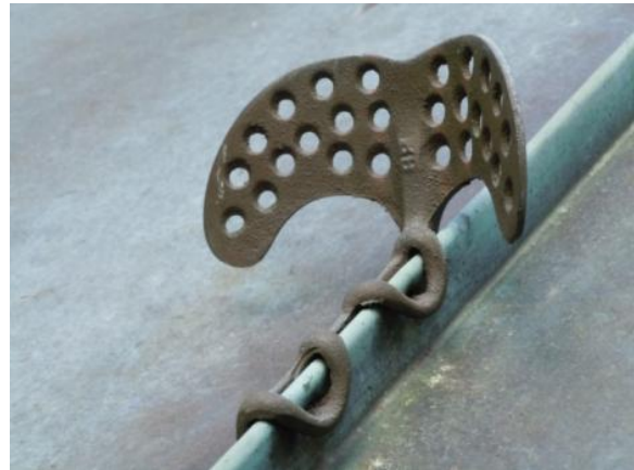
Figure 136, right. Metal snow guards are located at every seam on the metal roofs. Photo: HPTC (08/29/12).
