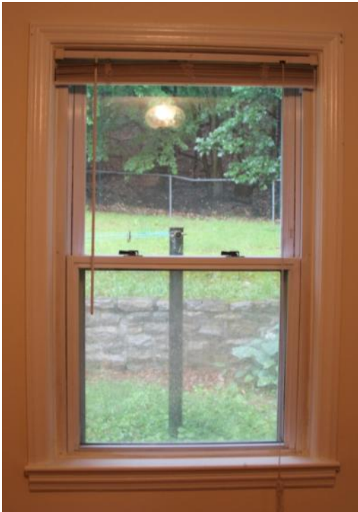
Figure 268. W126 is a vinyl replacement window. Photo: HPTC (06/12/12).
