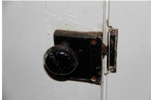
Figure 224. The entry to Room 003 includes an original rim lock. Photo: HPTC (06/20/12).
