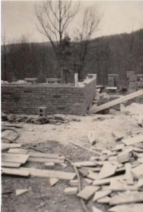
Figure 32. April 24, 1948 photograph showing the construction of the brick exterior walls. Photo: Progress Pictures of Custodian's Residence and Garage (Reconstruction). Catoclin Mountain Park archives. See Appendix C for larger copy of photographs.
