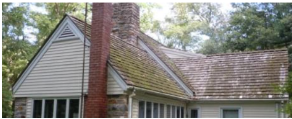
Figure 139. The eastern ell and sun porch gable roofs are now clad in cedar shakes. Photo: HPTC (08/29/12).
