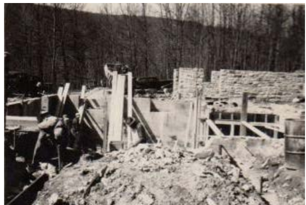
Figure 31. April 3, 1948 photograph showing the first residence's foundation and garage exterior walls to be reused. Photo: Progress Pictures of Custodian's Residence and Garage (Reconstruction). Catoclin Mountain Park archives. See Appendix C for larger copy of photograph.
