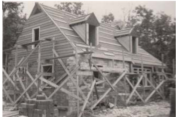
Figure 39. July 24, 1948 photograph of the residence from the northeast corner. Photo: Progress Pictures of Custodian's Residence and Garage (Reconstruction). Catoclin Mountain Park archives. See Appendix C for larger copy of photograph.
