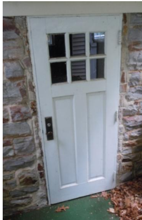
Figure 129. Exterior door DG103 is original to 1948. Photo: HPTC (08/29/12).
