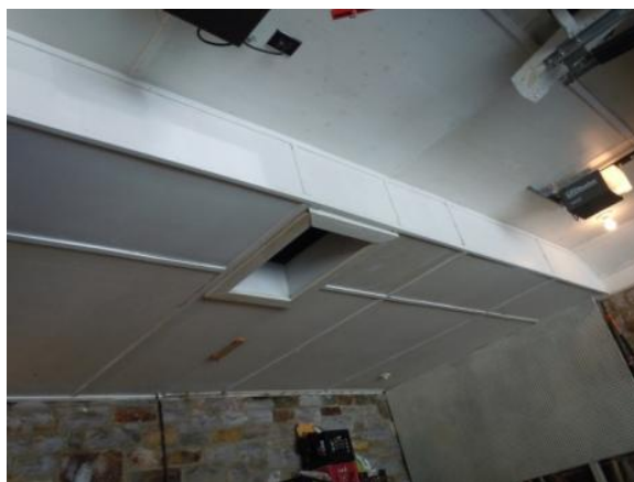
Figure 283. The painted board and batten wood ceiling of Room G101. Photo: HPTC (07/17/12).
