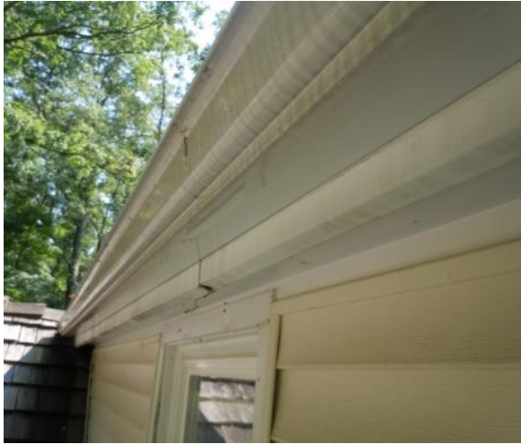
Figure 108. The metal-clad soffit of the rear dormer shed roof. Photo: HPTC (07/17/12).
