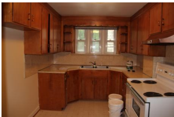
Figure 160. Wood base and wall cabinets with Formica countertops are located on the west, north, and east walls of the kitchen. Photo: HPTC (06/12/12).
