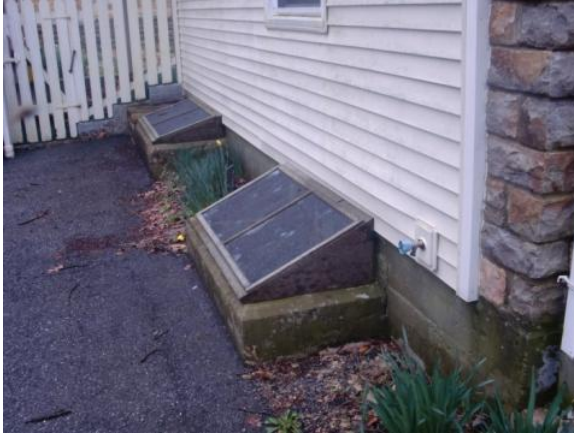
Figure 204, left, and Figure 205, right. Two areas most affected by poor site drainage are the north (left) and east (right) elevations mainly due to their orientation to the grade of the site causing the entrapment of moisture. Photos: HPTC: (03/21/12).
