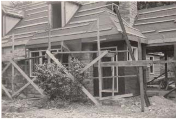
Figure 40. July 24, 1948 photograph of the front vestibule. Photo: Progress Pictures of Custodian's Residence and Garage (Reconstruction). Catoclin Mountain Park archives. See Appendix C for larger copy of photograph.
