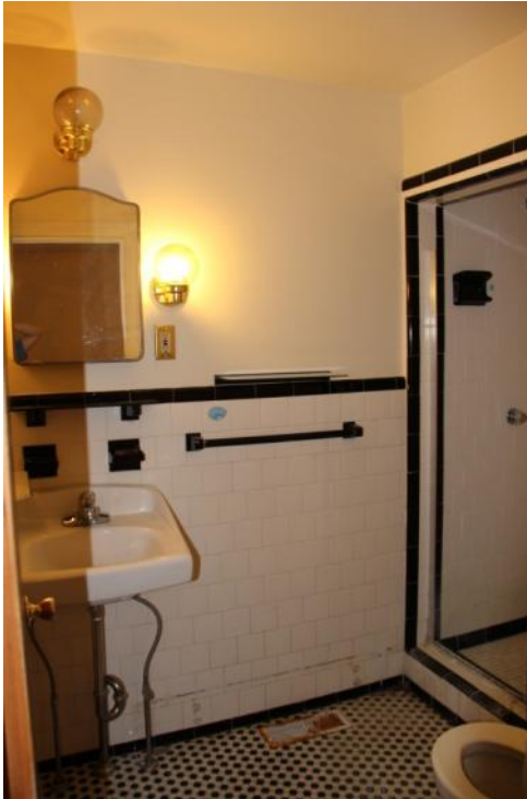
Figure 256. Room 107 looking northwest. Photo: HPTC (06/12/12).
