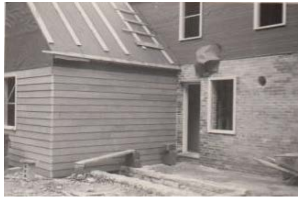
Figure 37. July 24, 1948 photograph of the eastern ell, exterior basement entry, and rear kitchen entry door. Photo: Progress Pictures of Custodian's Residence and Garage (Reconstruction). Catoclin Mountain Park archives. See Appendix C for larger copy of photograph.
