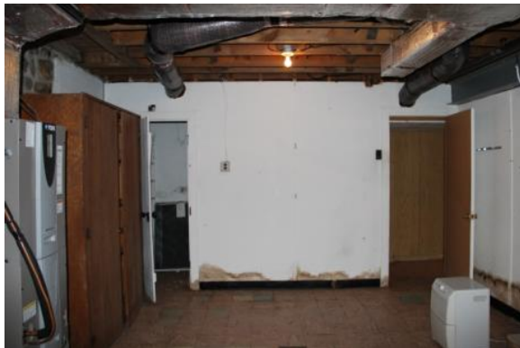
Figure 225 Room 004 looking west. Photo: HPTC (06/20/12).
