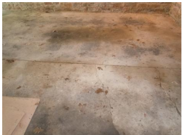
Figure 83. The garage concrete floor slab dates to 1941. Photo: HPTC (07/17/12).
