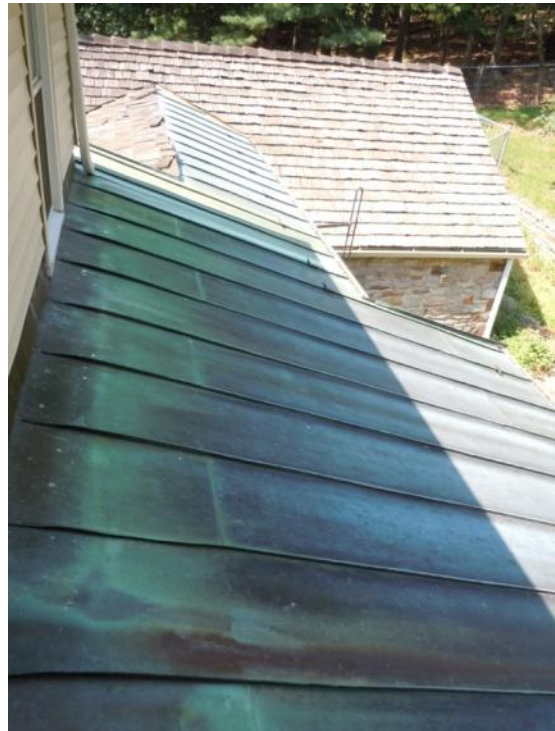
Figure 317. The standing-seam metal covering of the rear dormer shed roof is not original, but is a character-defining feature. Photo: HPTC (07/17/12).
