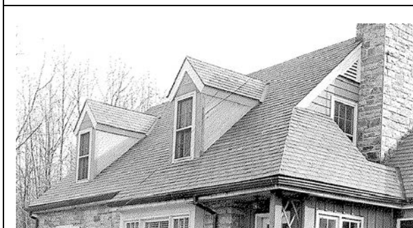
Figure 133. As seen in this ca. 1950 photograph, the main block gable/hipped roof and the front dormer gable roofs were originally slate. Photo: CATO Bldg. 128 building file.
