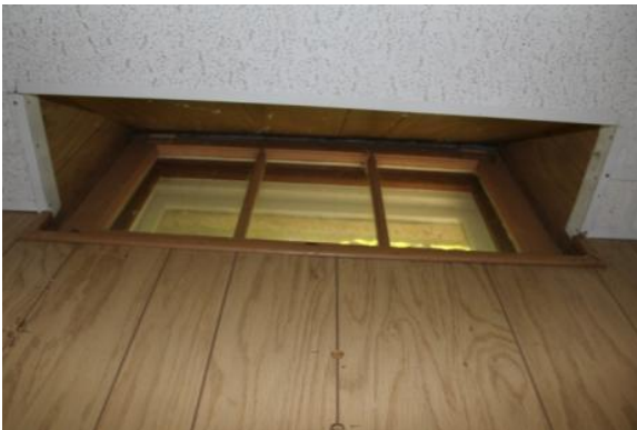
Figure 213. W003 is located on the west wall of Room 001; it is original. Photo: HPTC (06/20/12).
