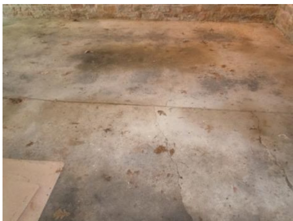
Figure 282. The exposed concrete slab floor of Room G101. Photo: HPTC (07/17/12).
