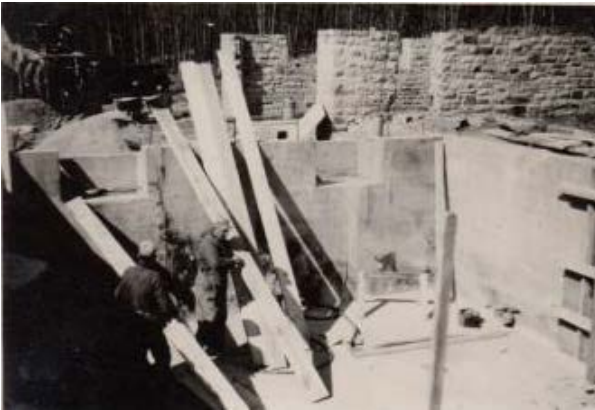
Figure 26. April 3, 1948 photograph of the first residence's foundation and garage exterior walls to be reused. Photo: Progress Pictures of Custodian's Residence and Garage (Reconstruction). Catoclin Mountain Park archives. See Appendix C for larger copy of photograph.
