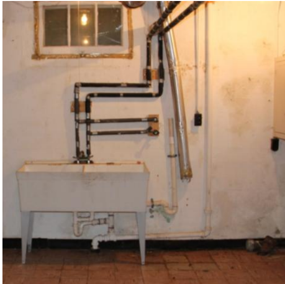
Figure 231. A modern laundry sink sits adjacent to washing machine hook-ups on the east wall. Photo: HPTC (06/20/12).
