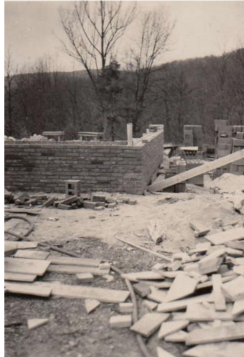
Figure 93. The north and east façade brick walls during construction; cement-block backing is located behind the brick. Photo: CATO archives (04/28/48).
