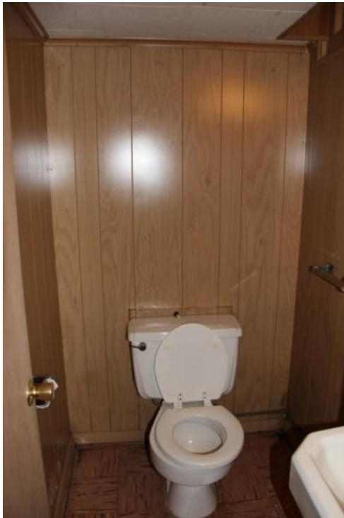
Figure 215. Room 002 looking south. Photo: HPTC (06/20/12).
