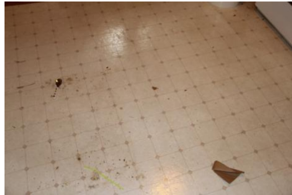
Figure 275. The modern vinyl floor covering in Room 112. Photo: HPTC (06/12/12).
