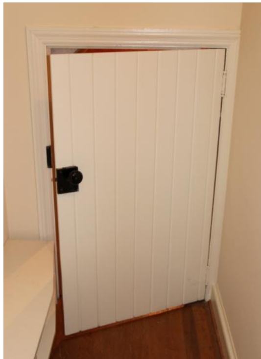
Figure 157. D205 is an original batten-style door on the second floor. Photo: HPTC (06/12/12).
