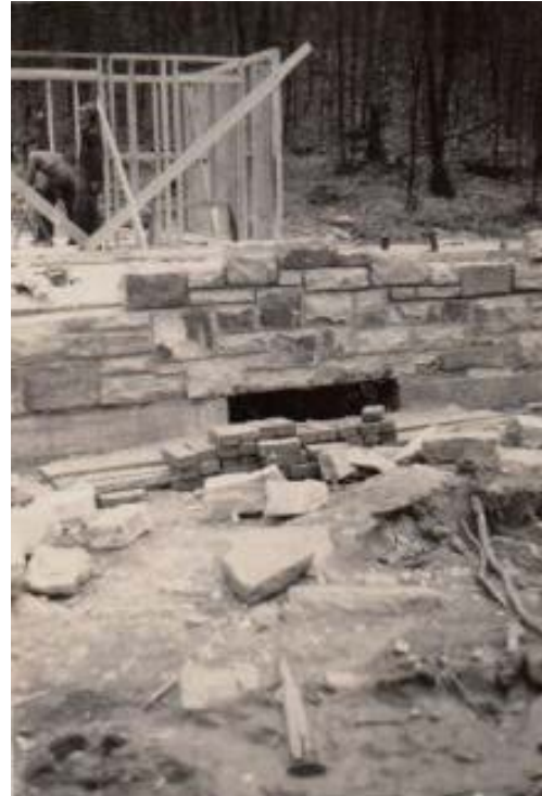
Figure 33. April 24, 1948 photograph showing the construction of the stone exterior wall. Photo: Progress Pictures of Custodian's Residence and Garage (Reconstruction). Catoclin Mountain Park archives. See Appendix C for larger copy of photographs.
