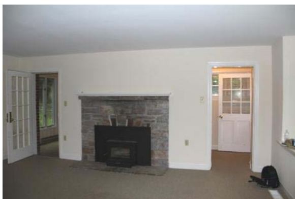
Figure 240. Room 103 looking south. The door opening, with historic door, to the left (D106) of the fireplace leads to Room 106; the door to the right (D103; historic door has been removed) leads to Room 104. Photo: HPTC (06/12/12).
