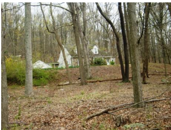
Figure 52. The front (west) elevation of Quarters 1 as seen from Park Central Road. Photo: HPTC (03/21/12).
