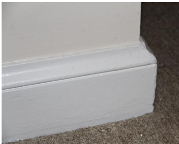
Figure 162. Painted wood baseboard with cyma reversa molding on the first floor. Photo: HPTC (06/12/12).
