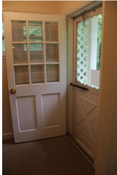
Figure 125. D104E was replaced in 1995. Photo: HPTC (06/12/12).
