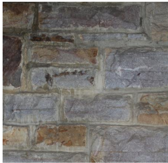
Figure 325. The west (front) façade and chimney of the main block and the garage exterior walls are constructed of local stone (likely Catoctin greenstone). Photo: HPTC (06/12/12).
