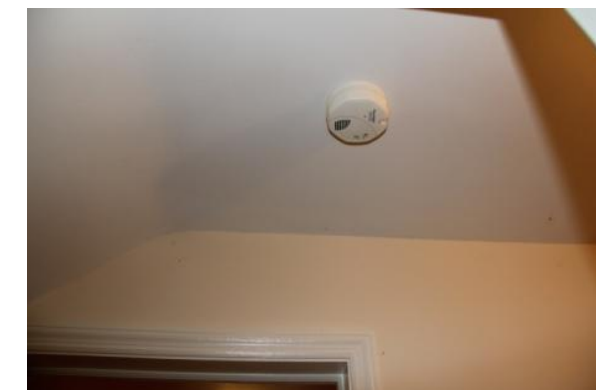
Figure 271. The ceiling is painted plaster. The battery-operated smoke and carbon monoxide detector is inoperable. Photo: HPTC (06/12/12).
