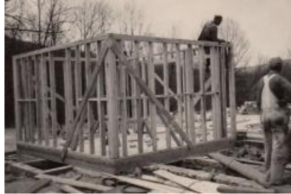
Figure 97. The eastern ell of the main block is frame construction. Photo: CATO archives (04/28/48).
