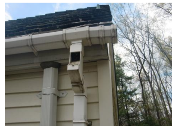
Figure 146. The vinyl drainage system on the south elevation of the eastern ell. The downspouts exhibit ice-dam prevention spouts. Photo: HPTC (04/21/12).
