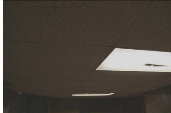
Figure 212. The ceilings are covered with a suspended acoustical tile system. Photo: HPTC (06/20/12).
