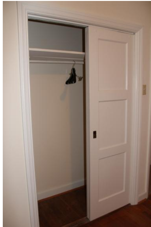
Figure 269. The interior of the closet (Room 108). The two original closet doors each have three panels with original recessed door pulls. Photo: HPTC (06/12/12).
