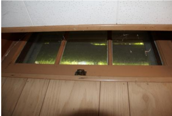
Figure 219. W004 is an original wood hopper window. Note the original locking hardware on the bottom rail. Photo: HPTC (06/20/12).
