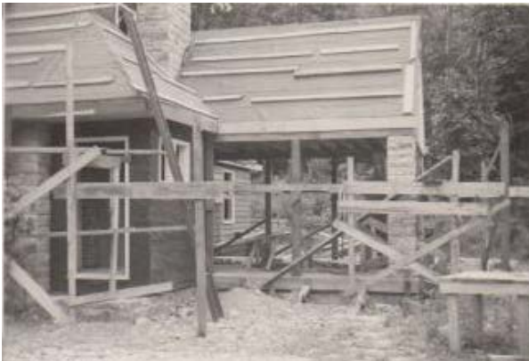
Figure 36. July 24, 1948 photograph showing the sun porch and vestibule. Photo: Progress Pictures of Custodian's Residence and Garage (Reconstruction). Catoclin Mountain Park archives. See Appendix C for larger copy of photograph.
