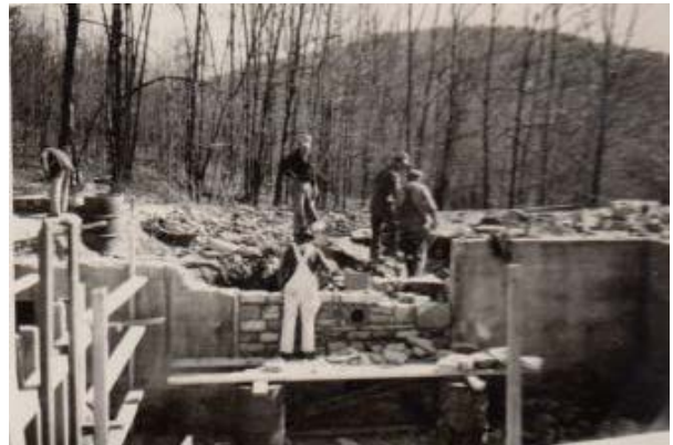
Figure 29. April 3, 1948 photograph showing the reconstruction of the stone chimney foundation. Photo: Progress Pictures of Custodian's Residence and Garage (Reconstruction). Catoclin Mountain Park archives. See Appendix C for larger copy of photograph.
