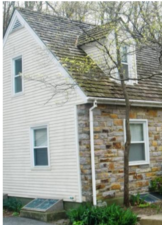
Figure 95. The brick on the north wall has been covered with vinyl siding. Photo: HPTC (04/21/12).
