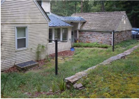
Figure 390. Neutral and negative drainage can be seen across the rear elevation. Photo: HPTC (08/29/12).
