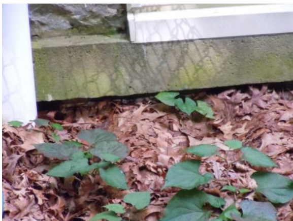
Figure 82. The 0'-5"-thick sun porch concrete slab is exposed on the exterior. Photo: HPTC (08/29/12).
