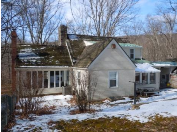
Figure 57. Quarters 1 from the southeast. Photo: HPTC (02/14/12).
