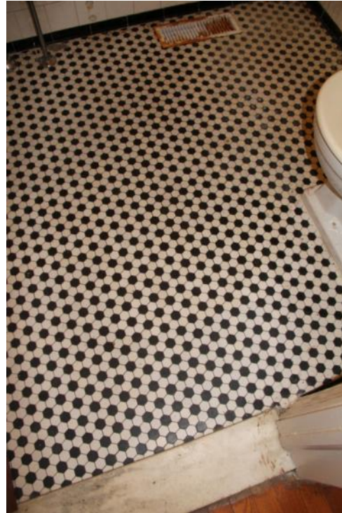
Figure 257. The floor of Room 107 includes historic ceramic hex-tile. Note the original marble door threshold. Photo: HPTC (06/12/12).
