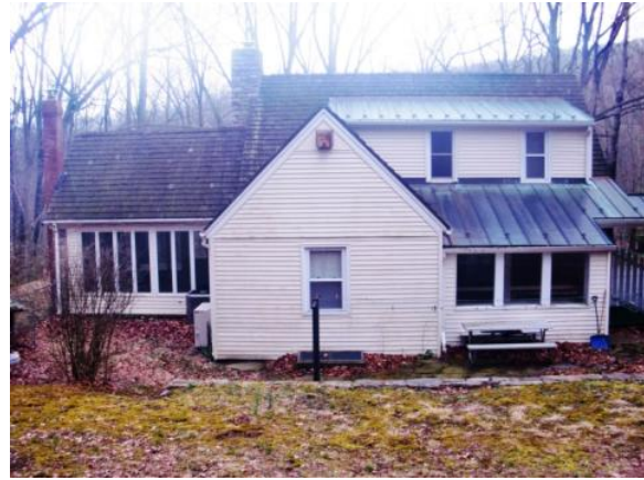
Figure 204, left, and Figure 205, right. Two areas most affected by poor site drainage are the north (left) and east (right) elevations mainly due to their orientation to the grade of the site causing the entrapment of moisture. Photos: HPTC: (03/21/12).
