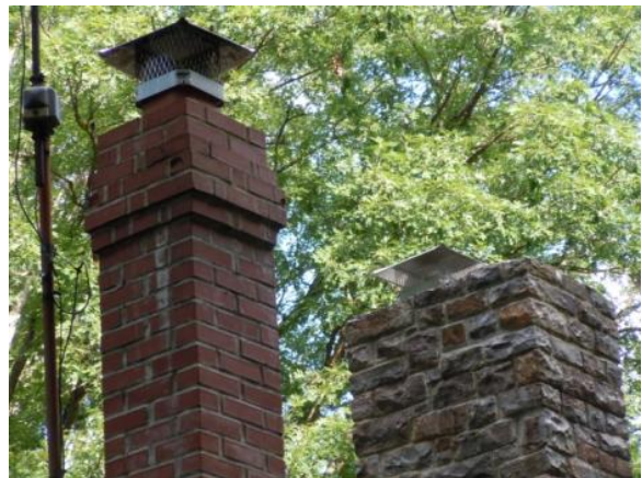
Figure 150. The main block stone chimney is original; the sun porch brick chimney was built in 1992. Photo: HPTC (08/29/12).
