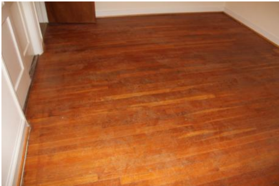
Figure 266. The original oak-strip flooring is exposed in Room 109. Photo: HPTC (06/12/12).
