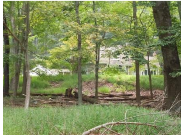
Figure 327. Quarters 1 is located on a heavily wooded lot in Catoctin Mountain Park. Photo: HPTC (06/12/12).
