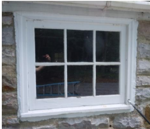
Figure 123. The 6-lite garage hopper windows are originally to the 1948 rebuild of Quarters 1. Photo: HPTC (08/29/12).
