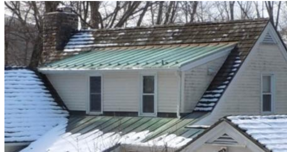
Figure 323. The rear shed dormer projects from the main block gable roof. Photo: HPTC (02/14/12).
