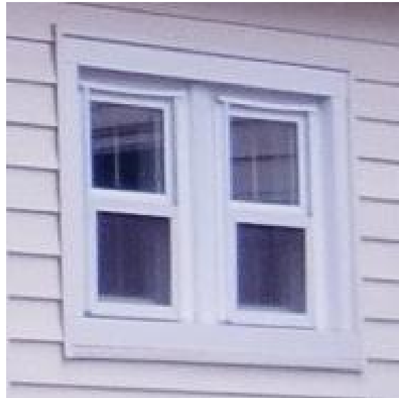
Figure 117. The vestibule windows have been replaced with vinyl-clad, double-hung units. Photo: HPTC (04/21/12).
